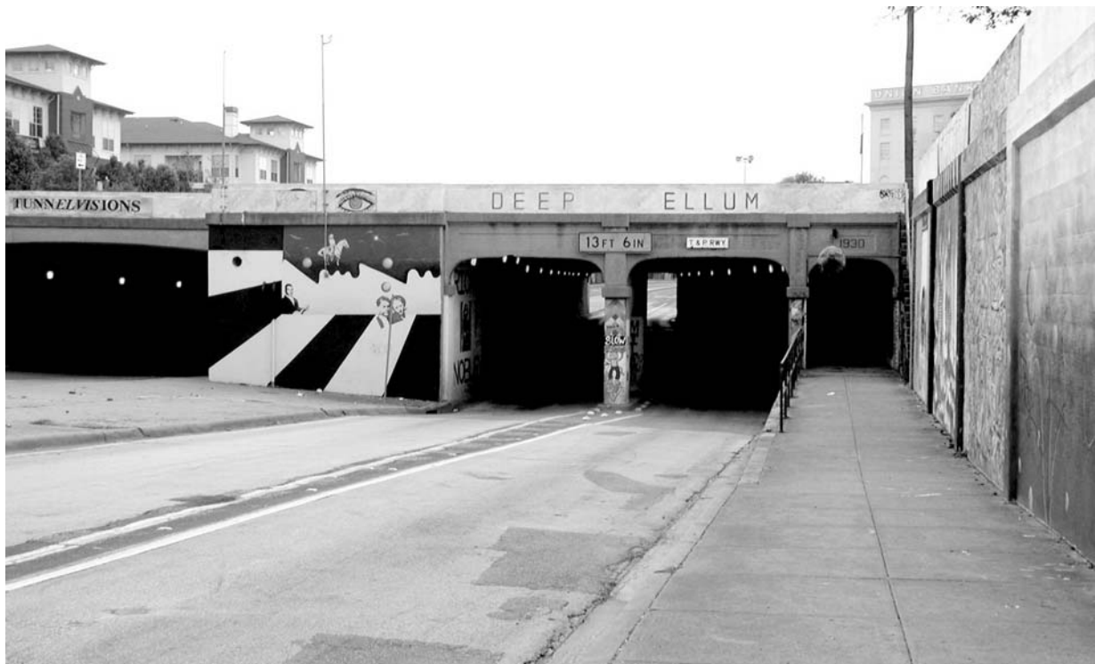
Figure E.5 View of Good-Latimer Tunnel Looking South
