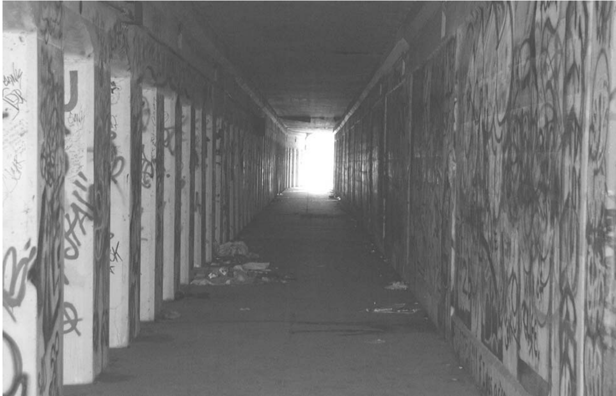
Figure E.6 View of Pedestrian Tunnel in the West Tunnel Section
