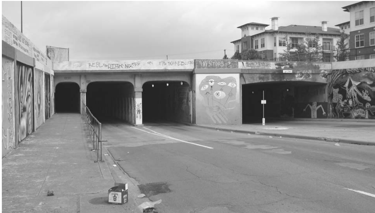
Figure E.4 View of Good-Latimer Tunnel Looking North
