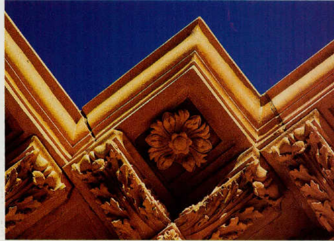
Detail on the Hutchings-Sealy building in Galveston. As a practitioner of “High Victorian” architectural style, Clayton loved to add lavish and colorful detail to his buildings. Perhaps his early years as a carver helped him design elaborate scrollwork and floral designs in three dimensions.
