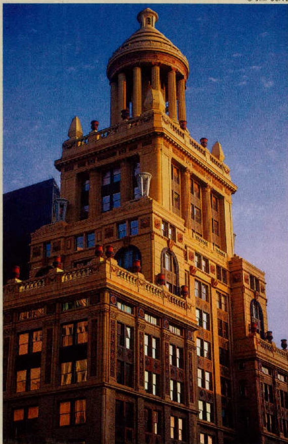
The Niels Esperson Building, at 808 Travis Street in downtown Houston, stands as a testament to Mellie Esperson’s undying devotion to her late husband, Niels.
