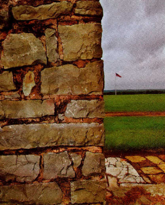
Buildings of locally quarried limestone define the edge of the Fort Griffin parade ground, where the solitary flagpole emphasizes the site's quiet remoteness.
