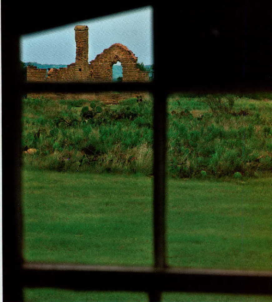
A glimpse of the Fort Griffin administration building ruins from a window of the Army post's bakery. A few fort structures are slated for restoration, or at least stabilization.
