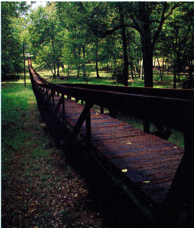
Footbridge Garden Park in Rusk
