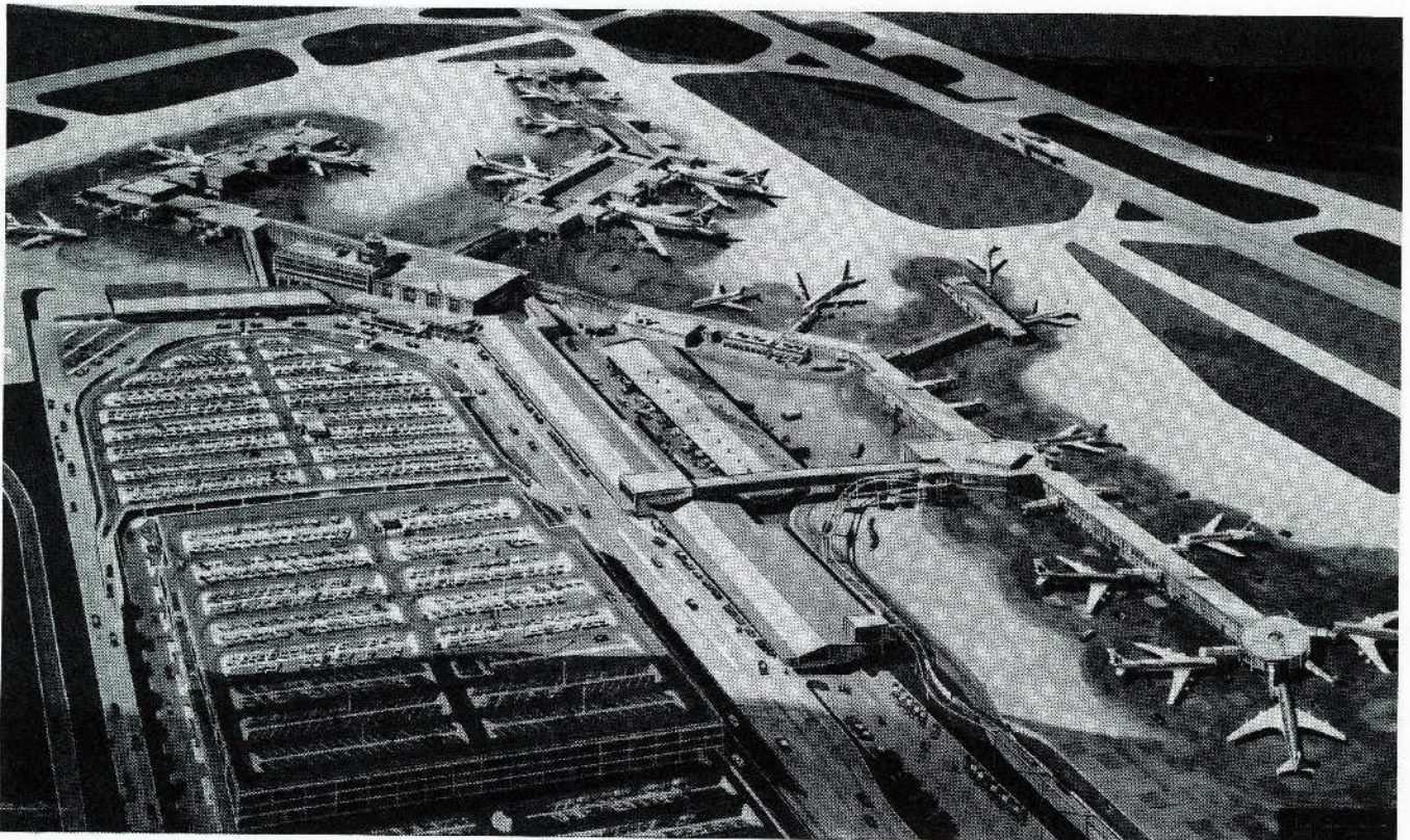
Problems of success. Additional passenger loading gates nearing completion, upper left and lower right, just keep pace with increased traffic at Dallas Love Field. Additional auto parking spaces, left foreground, are not yet under construction. (Rendition by Jack Corgan & Associates)
