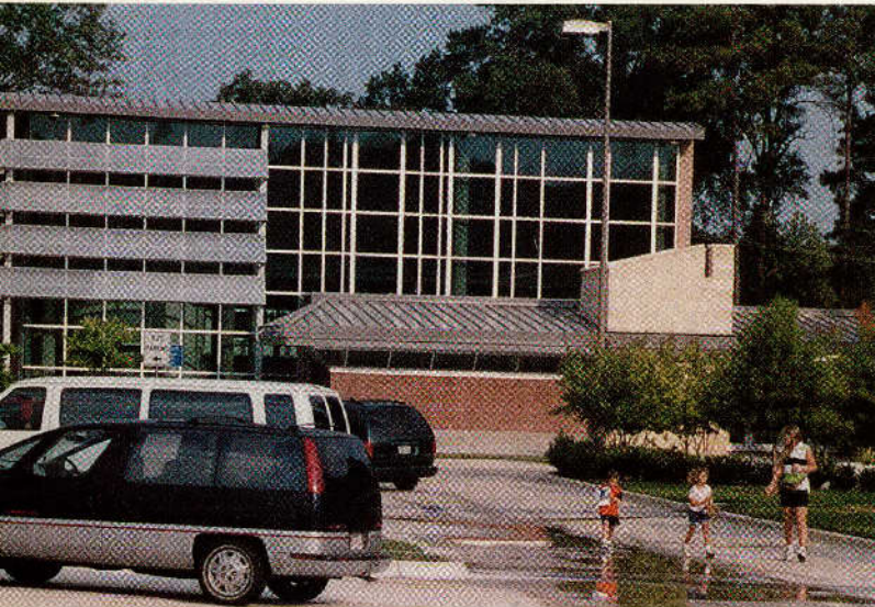
Texas Travel Information Center on I-30 at Texarkana
