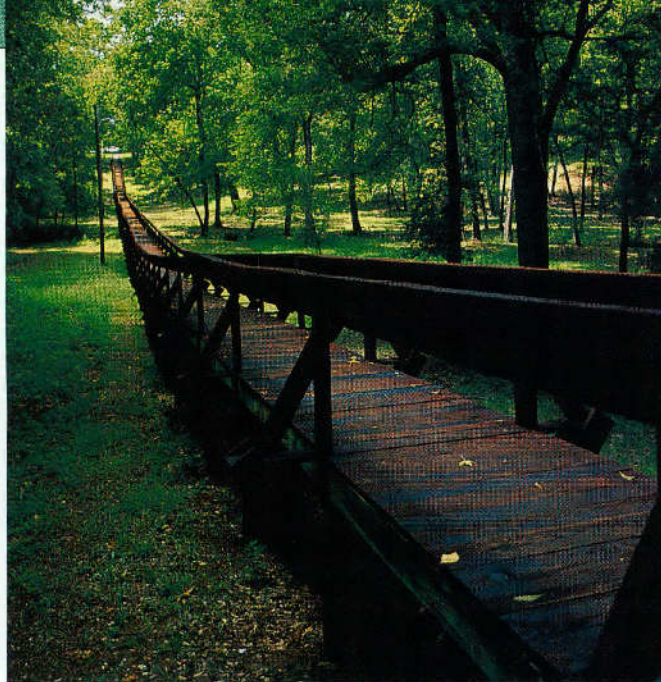
Footbridge Garden Park in Rusk
