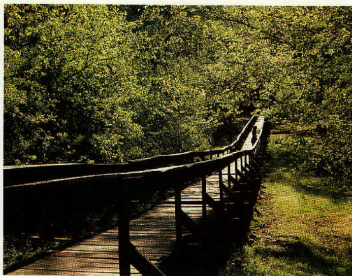
Footbridge Garden Park in Rusk
