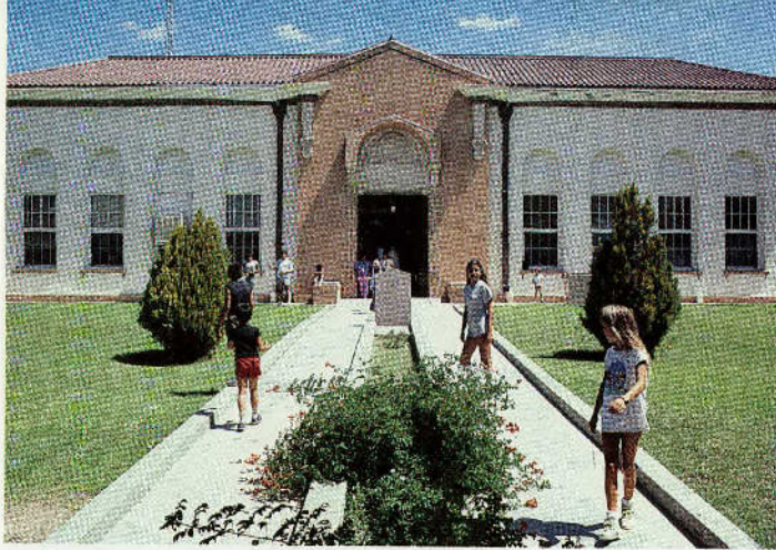
Hudspeth County Courthouse in Sierra Blanca is Southwest's only in-use government adobe structure
