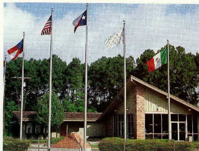
Texas Travel Information Center on I-10 in Orange
