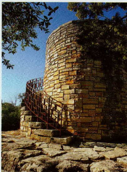
The water tower at Mother Neff State Park was built in the 1930s by the Civilian Conservation Corps.
