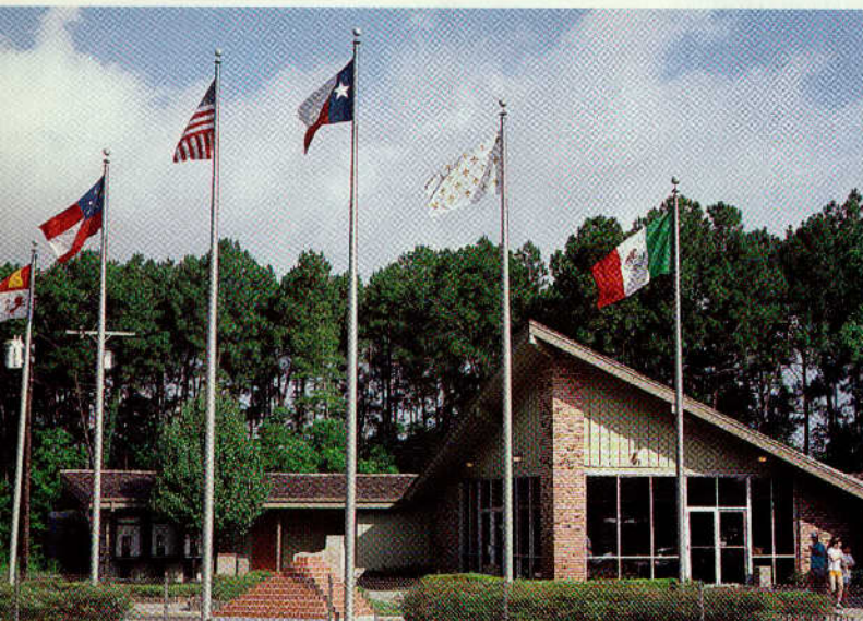
Texas Travel Information Center on I-10 in Orange
