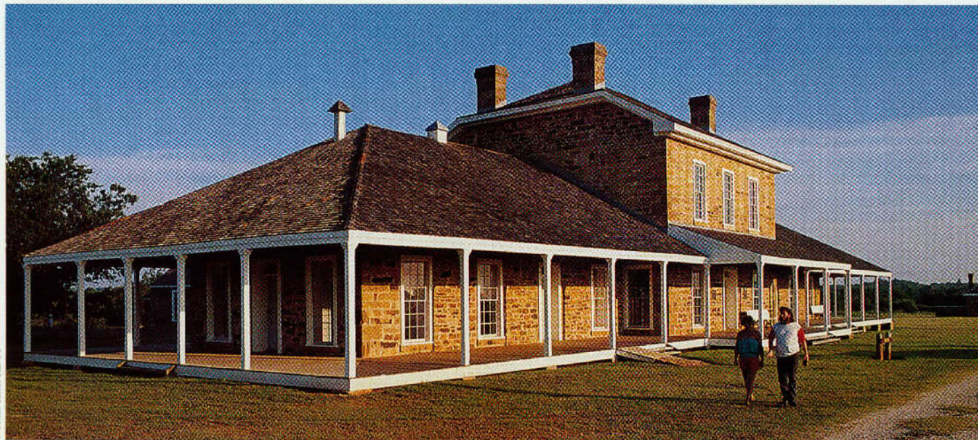
Restored Fort Richardson near Jacksboro
