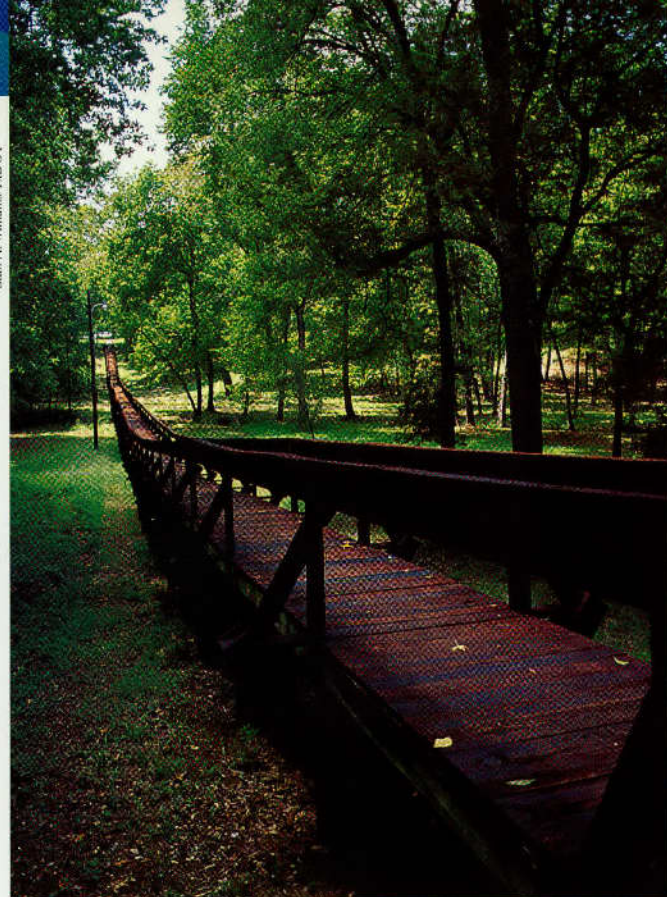
Footbridge Garden Park in Rusk
