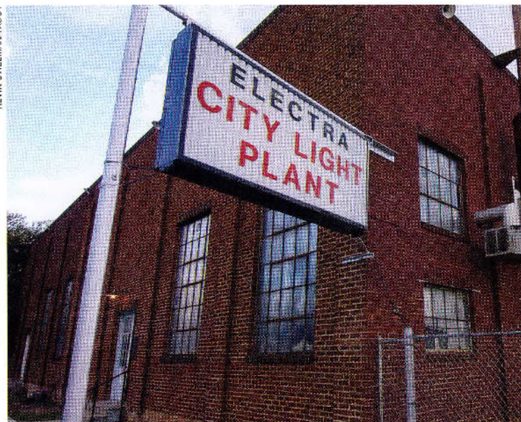
Old City Light Plant in Electra
