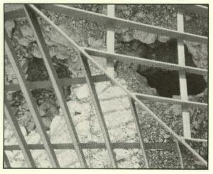
The EUWD has placed a grate over a sinkbole located in the flood pool of the San Antonio River Authority's dam site #10. The grate was installed to protect curious explorers and to keep the recharge feature intact. The sinkbole was acquired last summer as part of the Edwards Aquifer Preservation Program, and is located within a 51 acre conservation easement.
