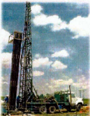
SAWS Saline Zone Drilling
