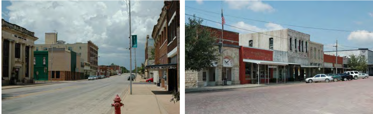
Figure 5-5 (left). 100 - 200 blocks of W. Main Street (RR 101), Ranger. The majority of buildings in downtown Ranger date to the oil-boom era of the late 1910s and 1920s and represent the community's most prosperous period of development.
