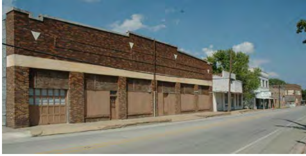
Figure B-19 (left). 100 block of W. College Street (SH 36), Rising Star.
