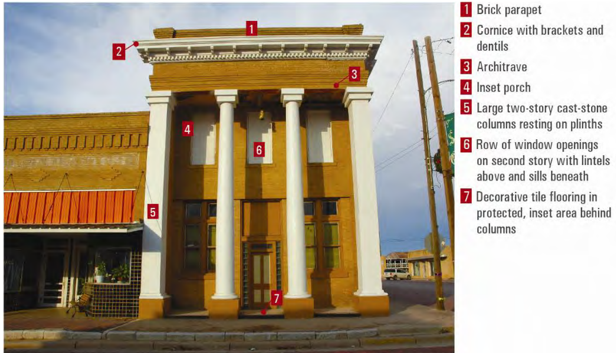
Figure 3-12. Temple Front building at the southwest corner of Edwards Street and N. Second Street, Merkel. This former bank is a good example of Temple Front building and features Classical Revival detailing.
