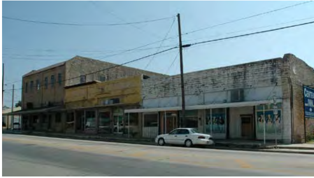
Figure B-5 (left). 100 block of N. Patrick Street (US 377 and US 67), Dublin.
