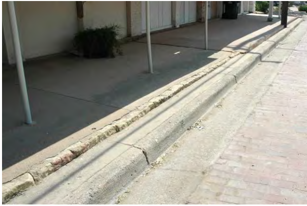
Figure 3-33 (top left). Stone and concrete curbing in Miles.
