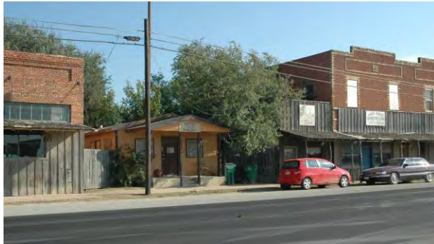
Figure 4-38. 100 block E. Dempsey Street (US 380), Bryson.
