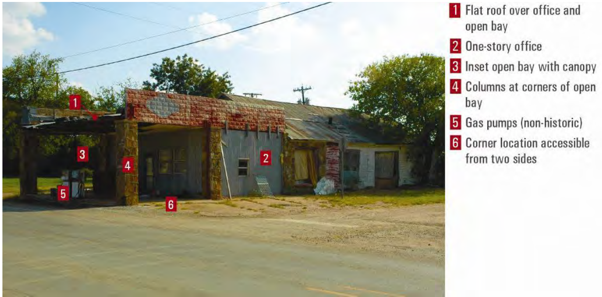
Figure 3-28. Box with Canopy building in 400 block of Ground Street, Moran.
