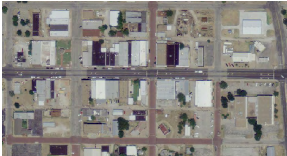
Figure C-6. Aerial view of downtown Olney. Commercial area without street names. Source: Bing.com
