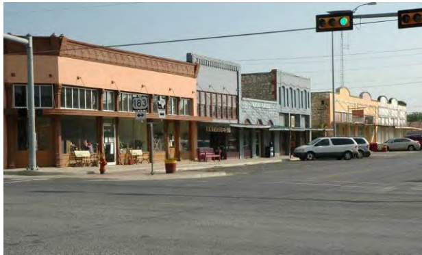
Figure B-9 (left). 100 block of W. Main Street, Lometa. North side of the block looking northeast.
