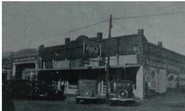
Figure C-9. Streetscape of 100 block of Edwards Street. Date ca. 1925–1930. Source: A Merkel Area History .
