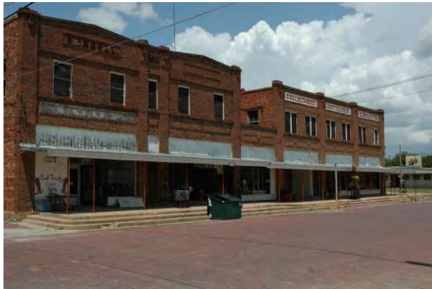
Figure 4-20 (left). Buildings with significance under Criterion C, 100 block of N. Rusk, Ranger.
