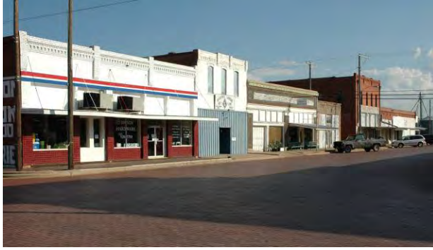
Figure B-11 (left). 100 block of Edwards Street, Merkel.
