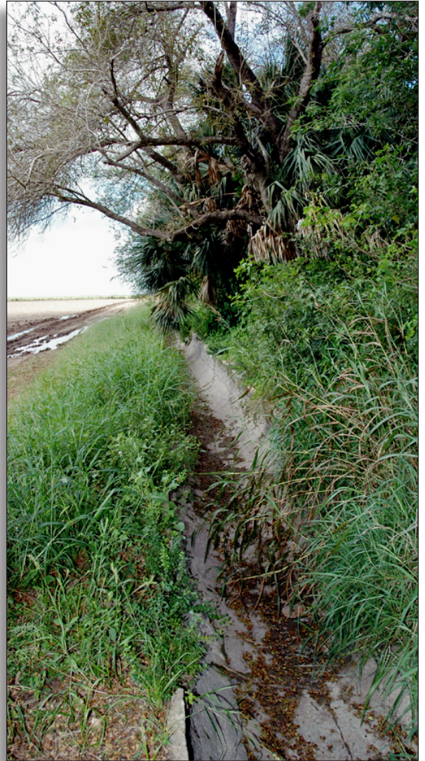
Figure 109: Brick lined lateral canal (1937), Cameron County Irrigation District No. 6.
