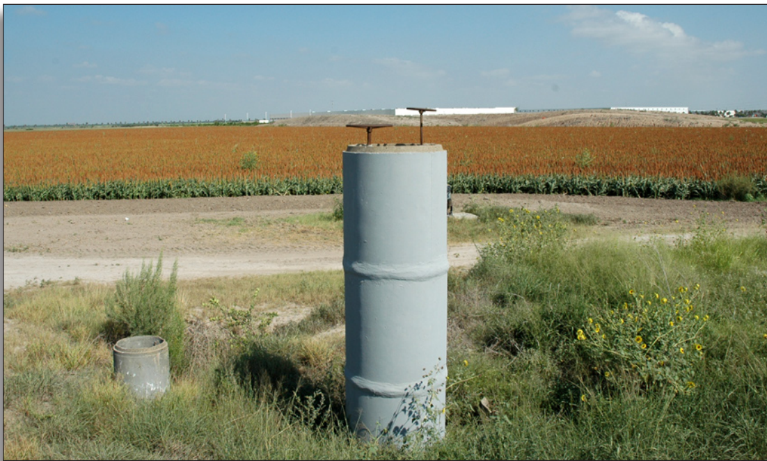
Figure 169: Mortar joint standpipe (1957) near levee on Bentsen Road, Hidalgo County Irrigation District No. 19.
