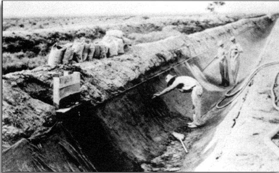
Figure 51: Lining canals in Hidalgo County Water Improvement District No. 2. Source: Brochu, Getting Up Steam
