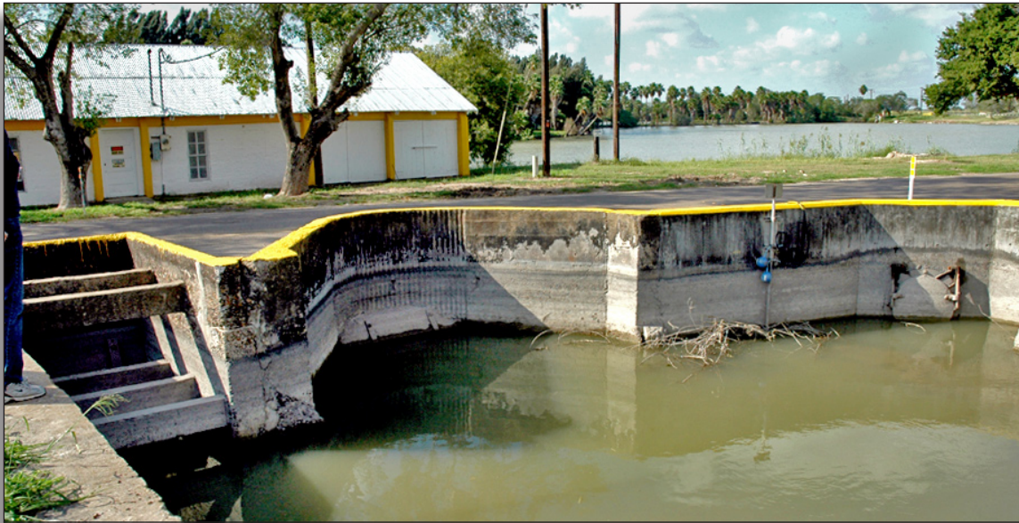
Figure 91: Main headworks, second lift pumphouse (1922), Cameron County Irrigation District No. 6.
