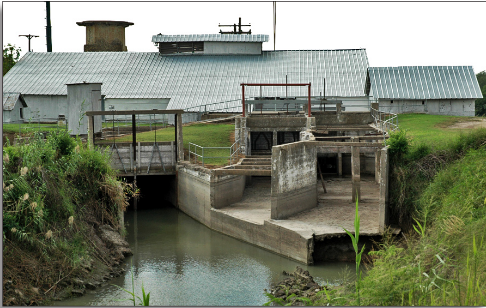
Figure 90: Main headworks, first lift pumphouse, Cameron County Irrigation District No. 6 (1929).
