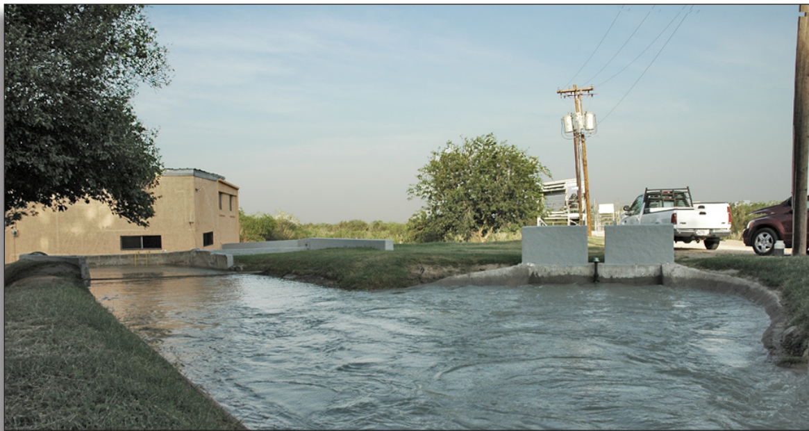
Figure 291: The intersection of old (left) and new (right) headworks provides contrasting examples of historic and contemporary materials, first lift pumping plant, Hidalgo County Irrigation District No. 3.
