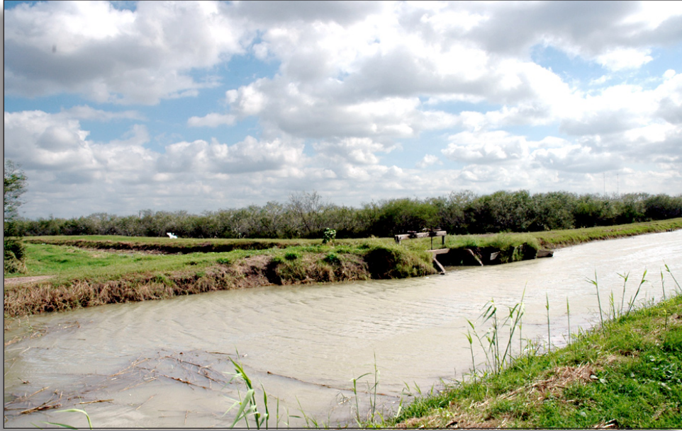
Figure 317: The rural setting contributes to the integrity of association of this canal, Cameron County Irrigation District No. 6.
