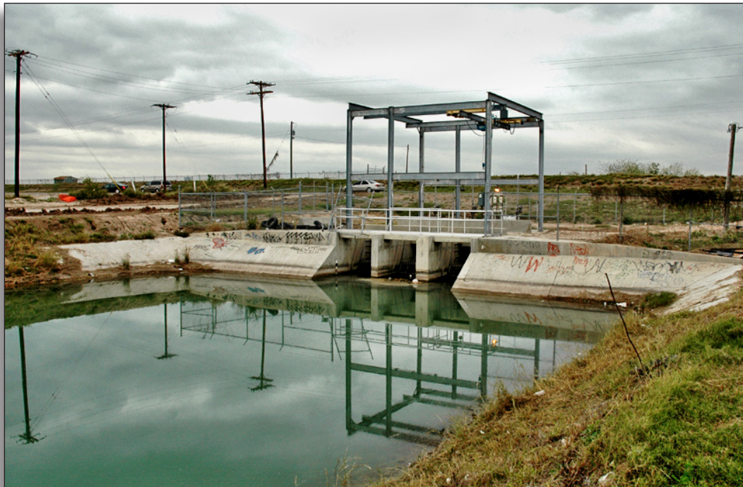
Figure 148: Electronic checkgate (2004) on Edinburg Main Canal, Los Ebanos Road, Hidalgo County Irrigation District No. 1.
