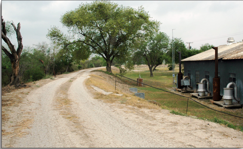
Figure 222: View of levee behind first lift pumping plant, United Irrigation District.
