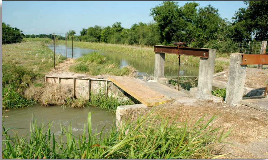
Figure 164: Division gate, Cameron County Irrigation District No. 2.
