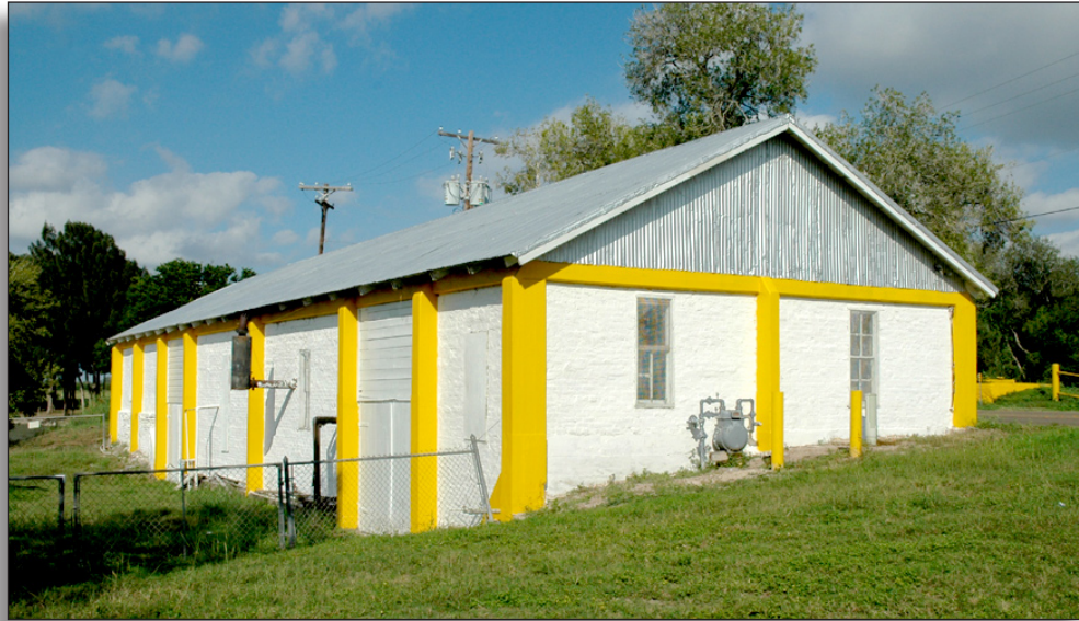
Figure 84: Second lift pumphouse (1922), Cameron County Irrigation District No. 6.
