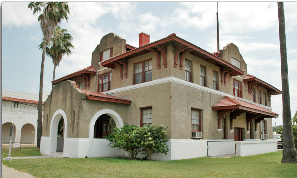
Figure 272: Former offices of the Cameron County Irrigation District No. 2, San Benito.
