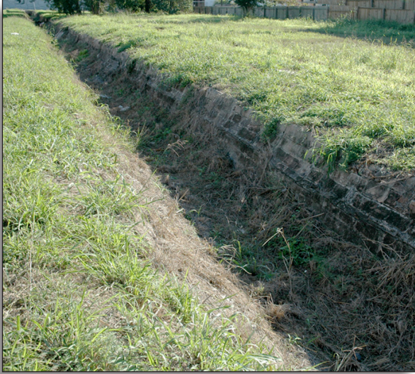
Figure 107: Brick lined canal (1938), Cameron County Irrigation District No. 6.
