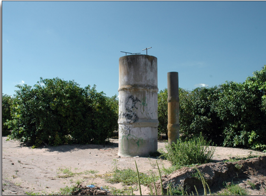
Figure 168: Mortar joint standpipes (1947) in citrus orchard along Ingle Road, Santa Cruz Irrigation District No. 15.
