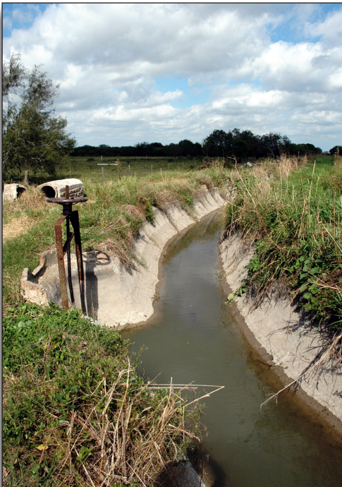
Figure 105: Concrete lined lateral canal (1937), Cameron County Irrigation District No. 6.
