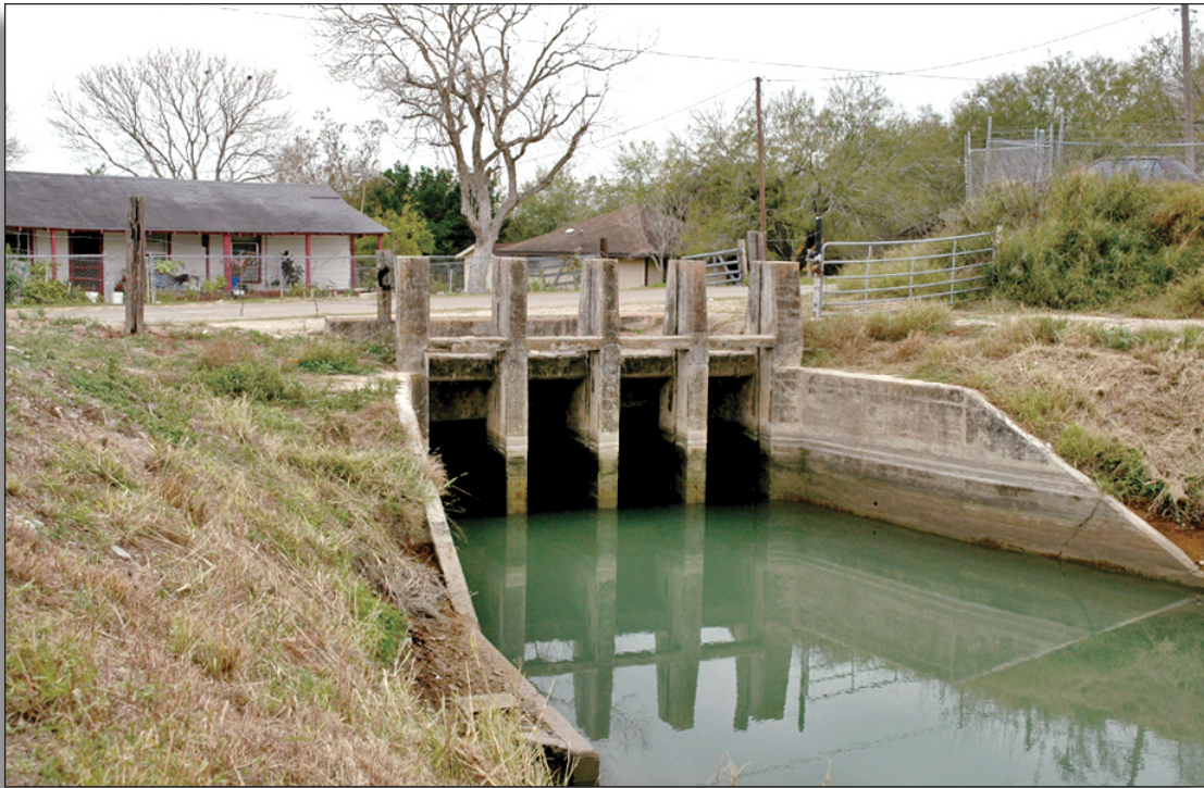
Figure 67: Headworks at beginning of Edinburg Main Canal, Hidalgo County Irrigation District No. 1.
