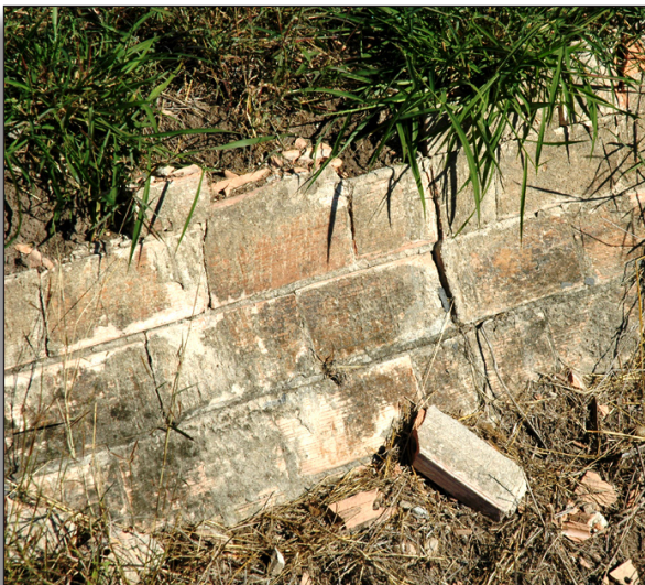
Figure 108: Detail of brick lined canal (1938), Cameron County Irrigation District No. 6.
