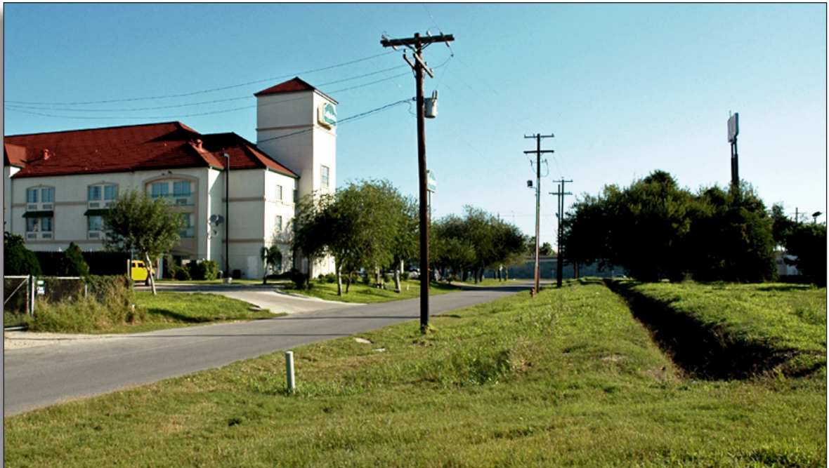
Figure 309: Stub Lateral at Tandy Road (near US 77/83) presents a loss of integrity of feeling due to urban intrusions, Cameron County Irrigation District No. 6.
