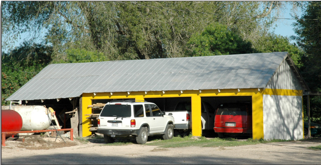
Figure 233: Shed and garage, Cameron County Irrigation District No. 6.
