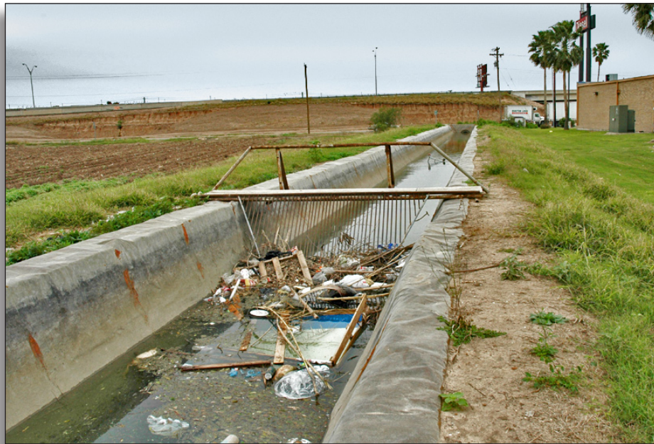
Figure 120: Geo-membrane lined lateral canal (2005) off FM 2128, Hidalgo County Irrigation District No. 1.
