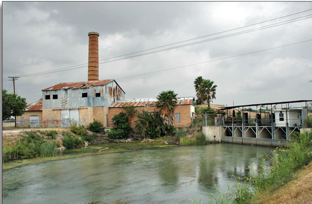
Figure 85: Old second lift pumping plant (1910), on left (NRHP, 2002), and new second lift pumping plant (1984), on right, United Irrigation District.
