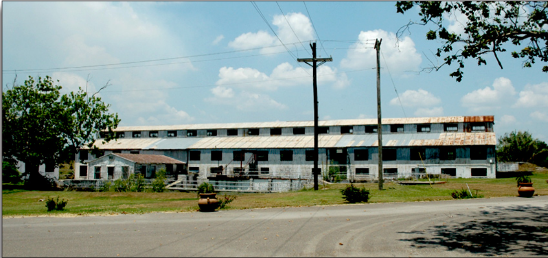
Figure 278: The old pumping plant at Los Indios, Cameron County Irrigation District No. 2, houses five non-historic pumps.
