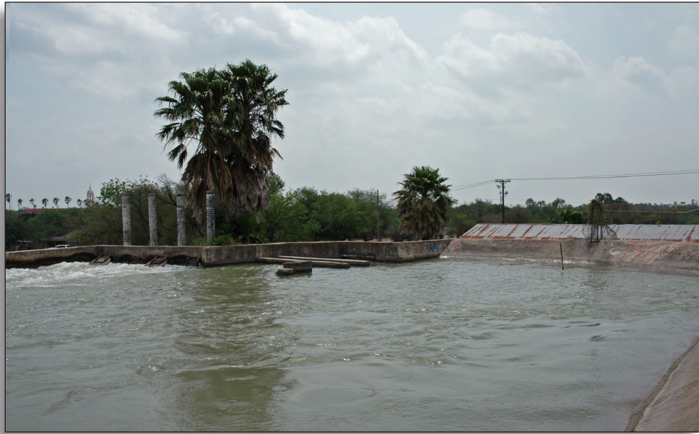
Figure 92: Intersection of new and old main headworks (1910/1984), second lift pumping plant, United Irrigation District.
