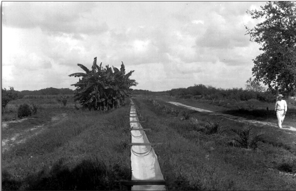
Figure 184: Early example of a concrete lined sub-lateral canal (c.1910). Source: Runyon Photograph Collection
