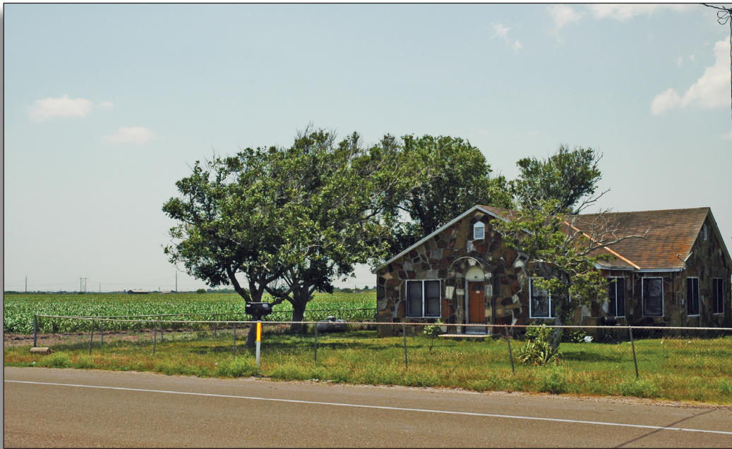
Figure 273: Farmstead in Cameron County Irrigation District No. 2.
