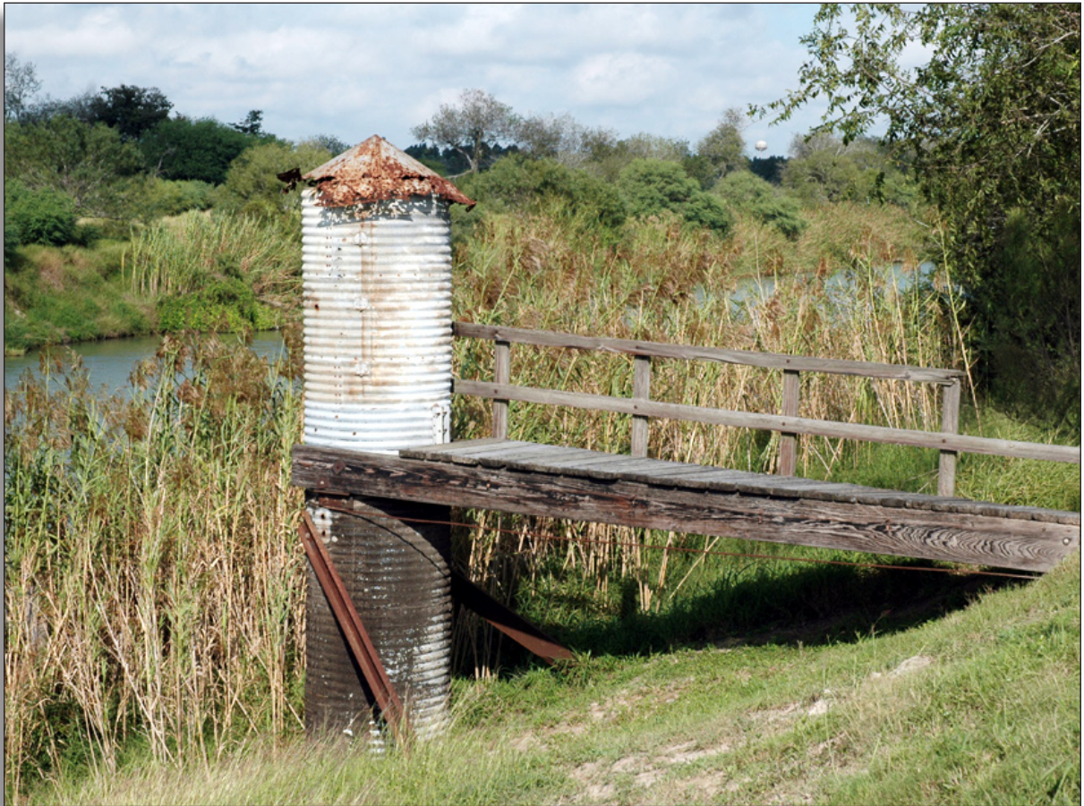
Figure 246: Gauging station, International Boundary & Water Commission, first lift pump house, Cameron County Irrigation District No. 6.
