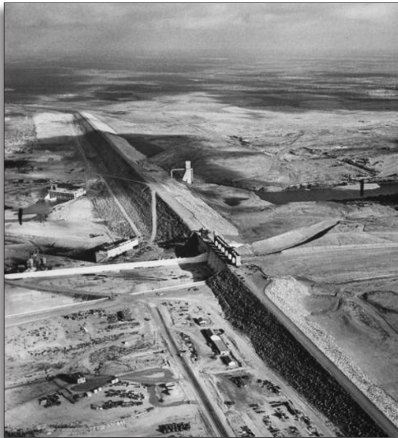
Figure 247: Falcon Dam under construction. Source: Life Magazine , June, 1953
