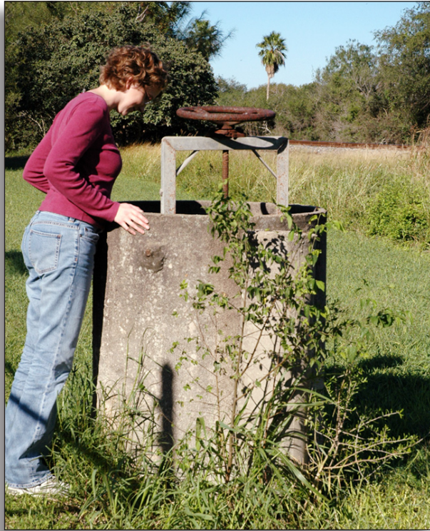
Figure 178: Diversion stand, Cameron County Irrigation District No. 6.
