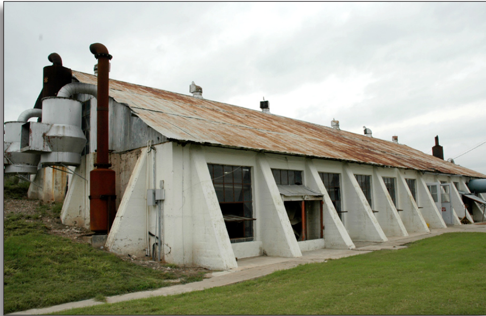
Figure 79: First lift pumphouse (1927), Hidalgo County Irrigation District No. 1.
