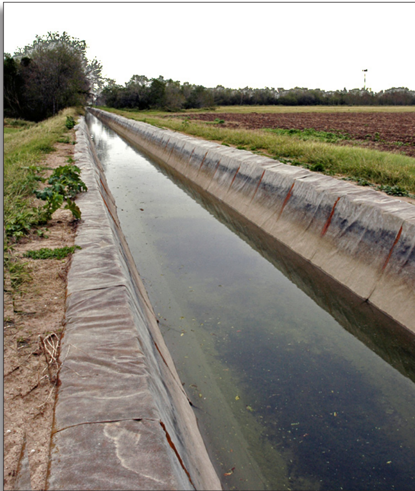
Figure 289: Modern geomembrane lining material of this lateral canal did not exist during the historic period, Hidalgo County Irrigation District No. 1.
