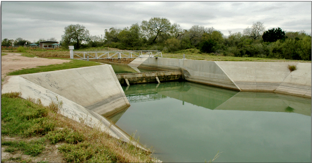
Figure 288: This electronic weir, designed by engineers Meldon and Hunt, is an example of alteration to the design of earthen Edinburg Main Canal.
