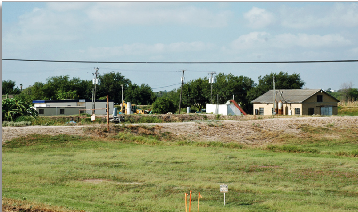
Figure 280: Pumping plant, right, with new manufactured buildings moved on site, Hidalgo County Irrigation District No. 19.
