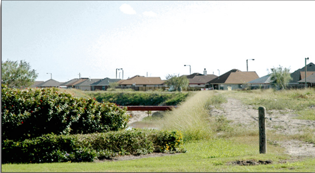
Figure 218: Drainage ditch off Curve Road, Hidalgo County Irrigation District No. 1.
