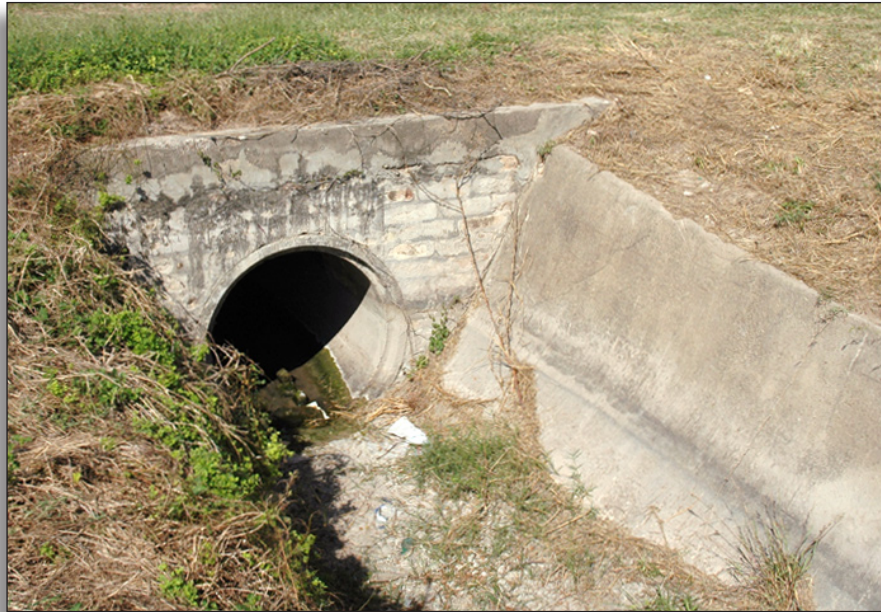
Figure 132: Concrete pipe culvert, Cameron County Irrigation District No. 6.
