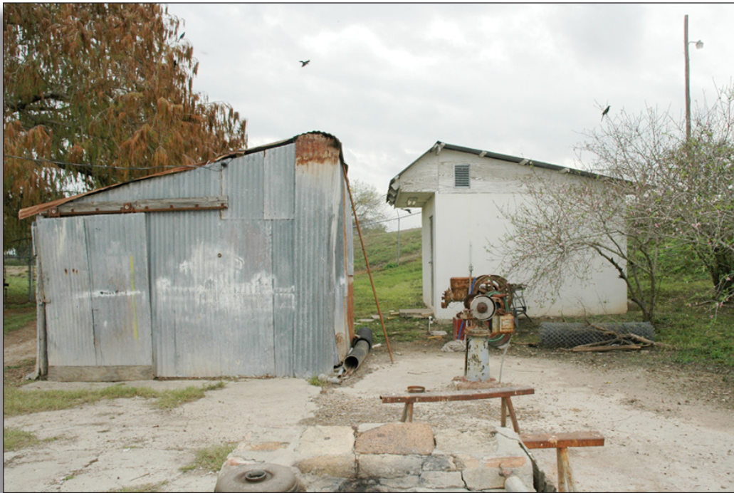
Figure 236: Sheds at first lift pumping plant, Hidalgo County Irrigation District No. 1.
