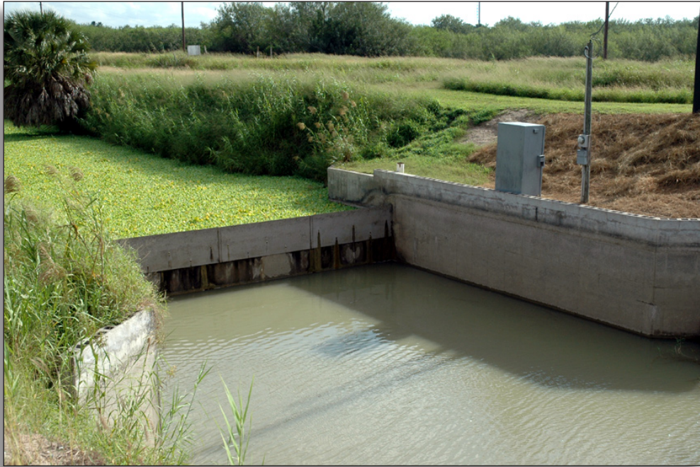
Figure 158: Weir on main canal, Cameron County Irrigation District No. 6
