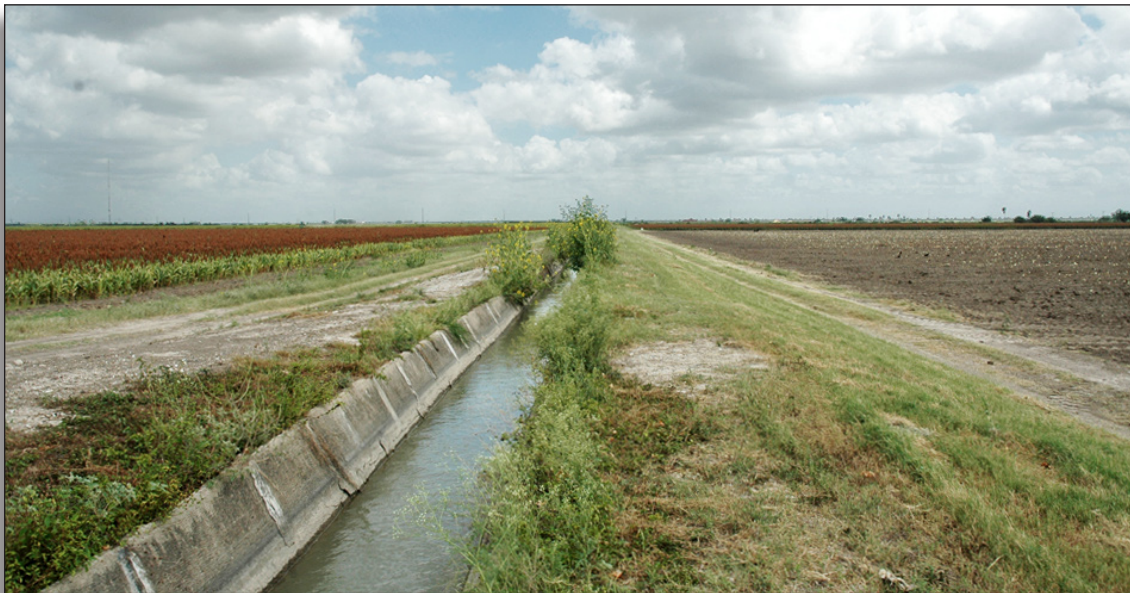
Figure 118: Bodine Lateral, Hidalgo County Irrigation District No. 19.
