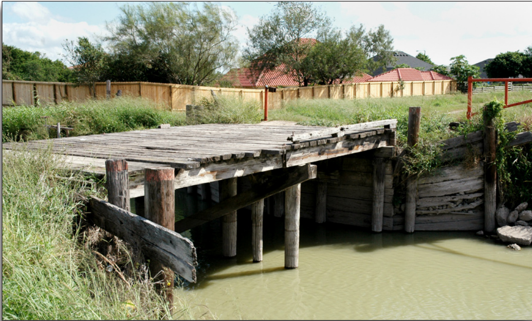
Figure 211: Canal bridge (c.1925) near reservoir, Cameron County Irrigation District No. 6.
