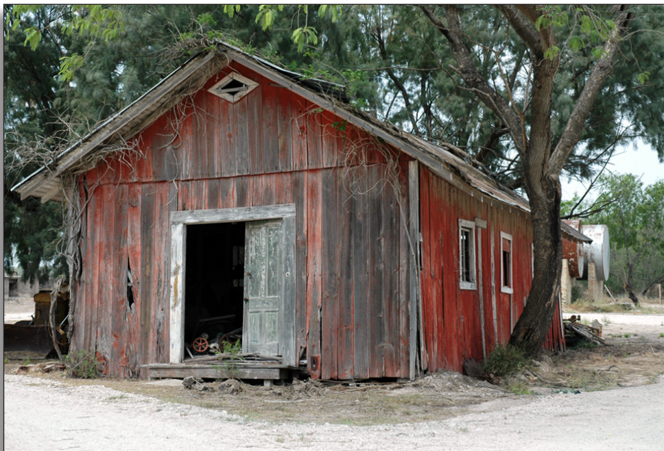
Figure 234: Barn (c.1921), Old Third Lift Pumping Plant, United Irrigation District.
