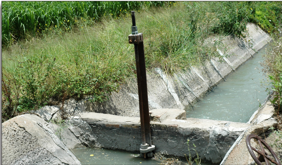
Figure 271: Small check gate in Samuelson Lateral Canal, Hidalgo County Irrigation District No. 19.
