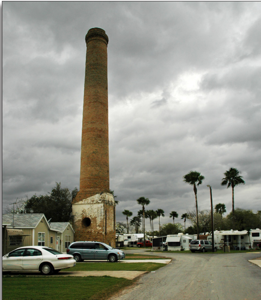
Figure 314: The surviving chimney stack of the original First Lift Pumping Plant, located in a trailer park at Chimney Park, has lost all integrity of association, formerly part of United Irrigation District.
