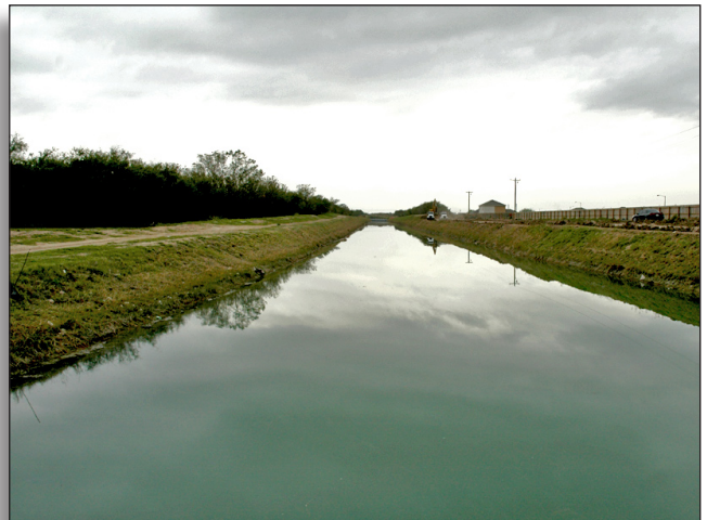
Figure 103: Earthen Edinburg Main Canal (1912/1926), Hidalgo County Irrigation District No. 1.
