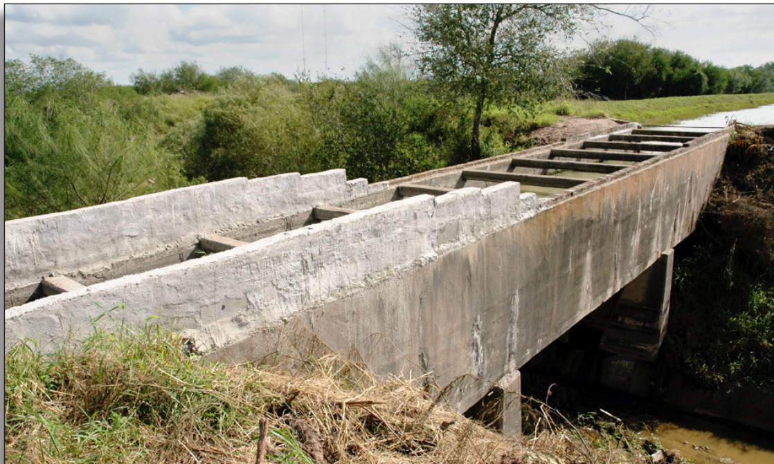
Figure 127: Box flume (1936/1998), Cameron County Irrigation District No. 6.
