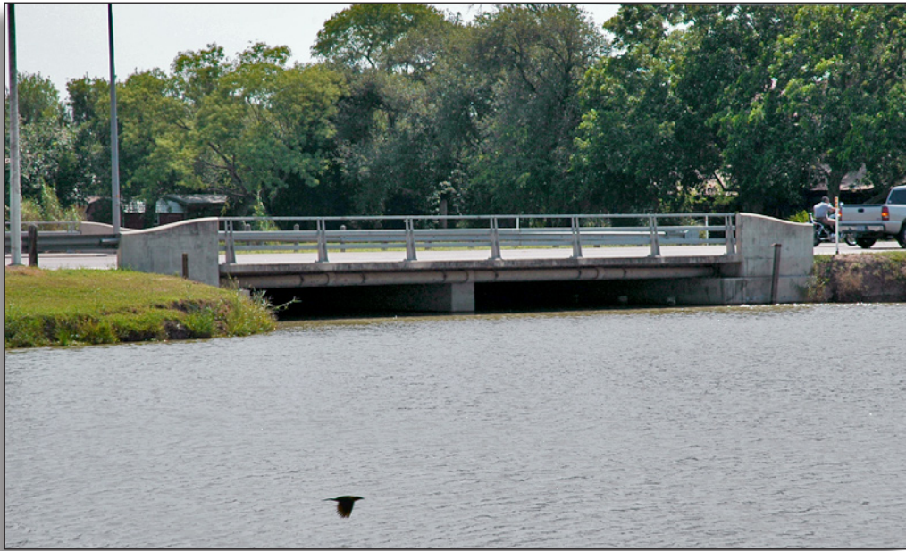
Figure 210: Bridge across Resaca de Los Fresnos, Business US 77 in Los Fresnos, Cameron County Irrigation District No. 2.
