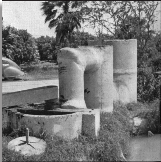
Figure 166: Early concrete standpipe (c.1935). Source: Loving, Concrete Pipe for Irrigation and Drainage
