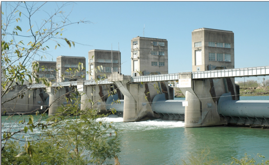
Figure 249: Construction of Anzalduas Dam was completed in 1960.
