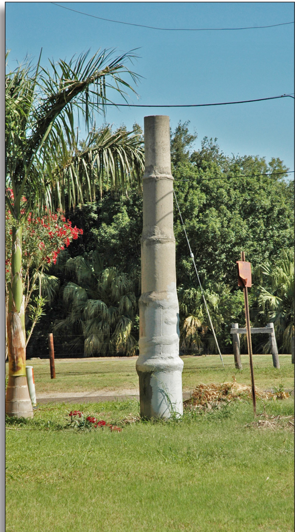
Figure 172: Mortar joint standpipe (1960s) on Glasscock at Fair Oaks, United Irrigation District.
