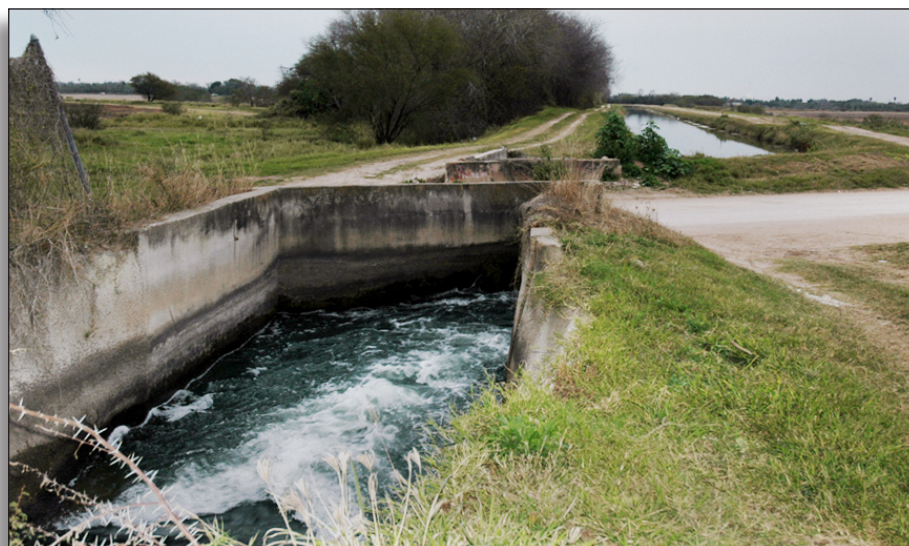
Figure 131: Siphon (c.1930) under road, Hidalgo County Irrigation District No. 1.
