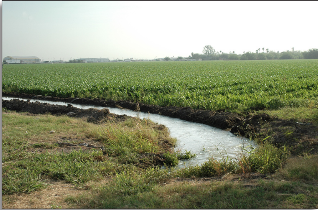
Figure 185: View of sub-lateral, Hidalgo County Irrigation District No. 3.
