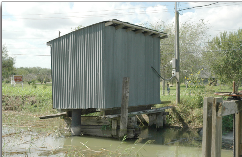
Figure 88: Pumping shed, Cameron County Irrigation District No. 6.
