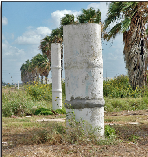
Figure 170: Row of mortar joint standpipes (1994), FM 494, Hidalgo County Irrigation District No. 19.
