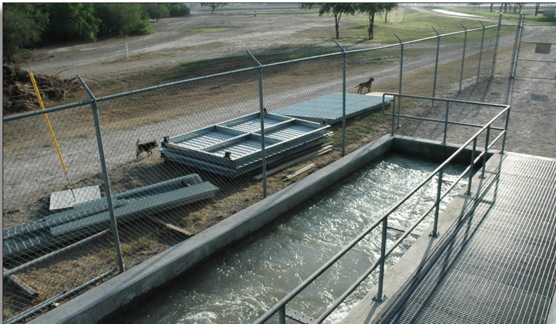
Figure 93: Detail of new headworks (2005), Hidalgo County Irrigation District No. 3.
