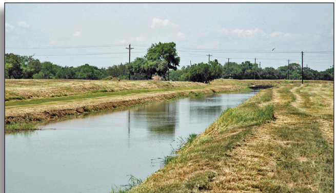
Figure 111: High Line Canal, Cameron County Irrigation District No. 2.
