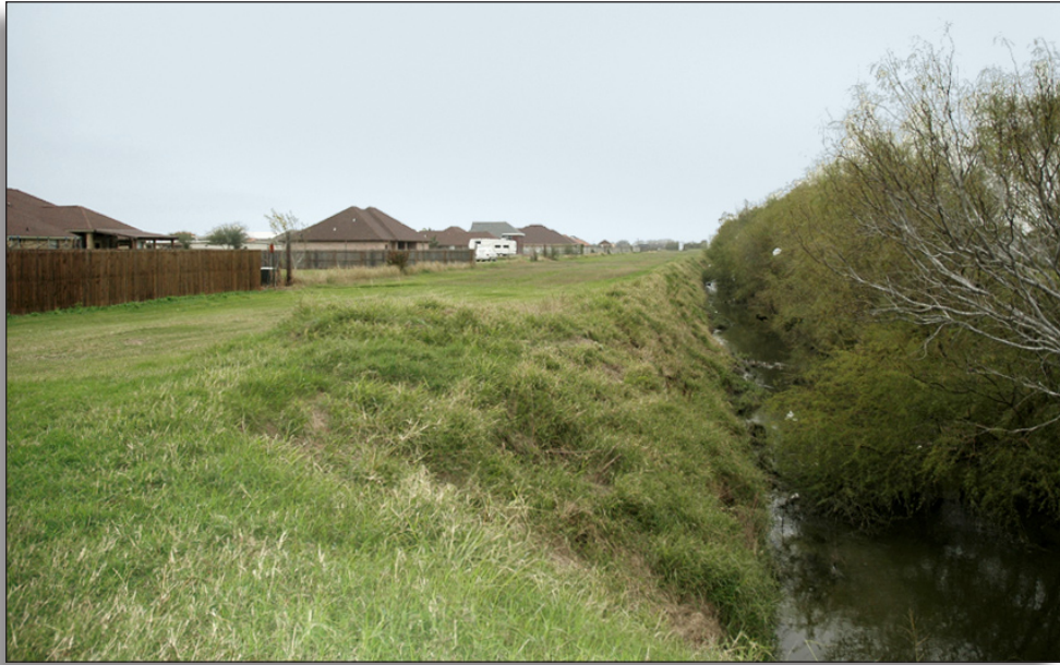
Figure 138: Curry Main Canal (underground pipeline) adjacent to drainage ditch, south of Curry Avenue, Hidalgo County Irrigation District No. 1.
