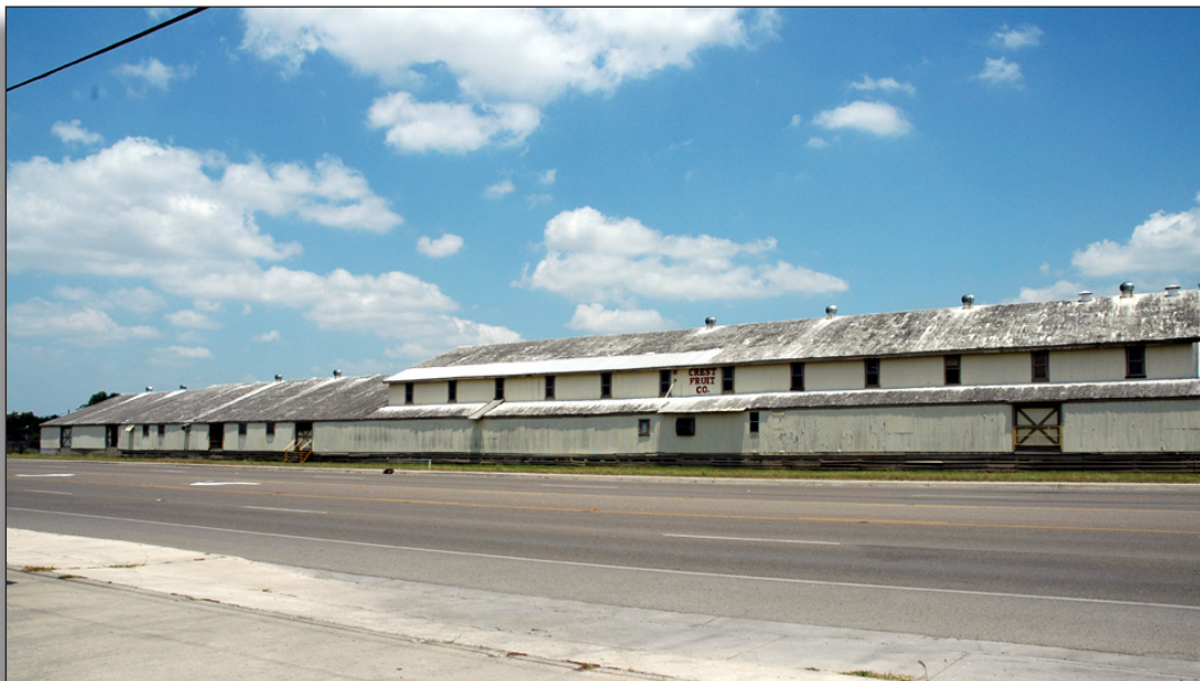
Figure 263: View of Crest Fruit Company looking northwest across Business 83 and railroad tracks.
