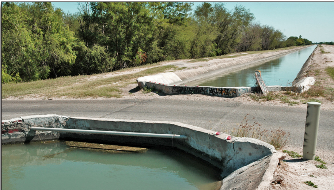
Figure 133: Siphon on Bryan Canal Main Canal, United Irrigation District.
