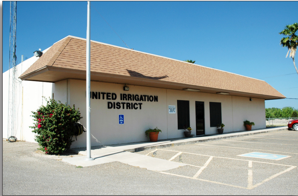
Figure 227: United Irrigation District offices located north of Mission on Mile 2 North Road.
