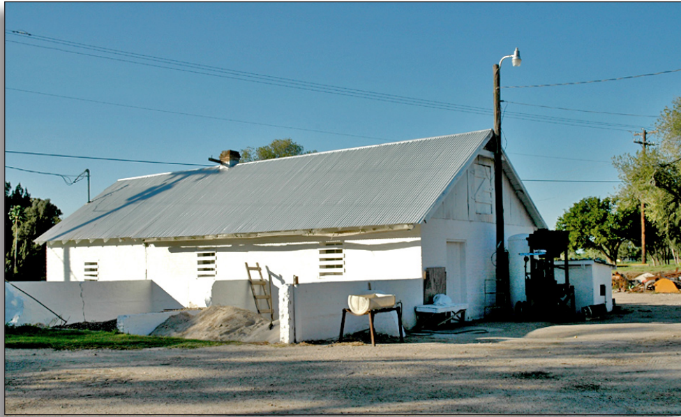
Figure 229: Warehouse (1925) at second lift, Cameron County Irrigation District No. 6.
