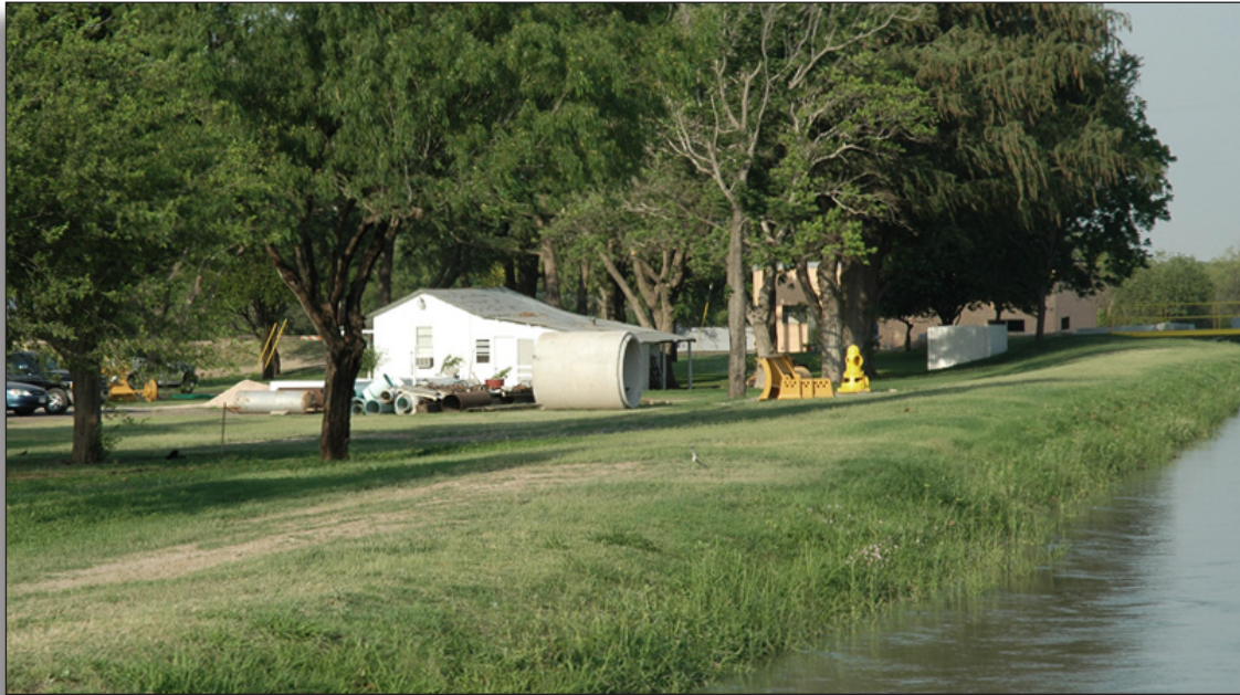
Figure 242: Employee housing (c.1935) at first lift pumping station, Hidalgo County Irrigation District No. 3.
