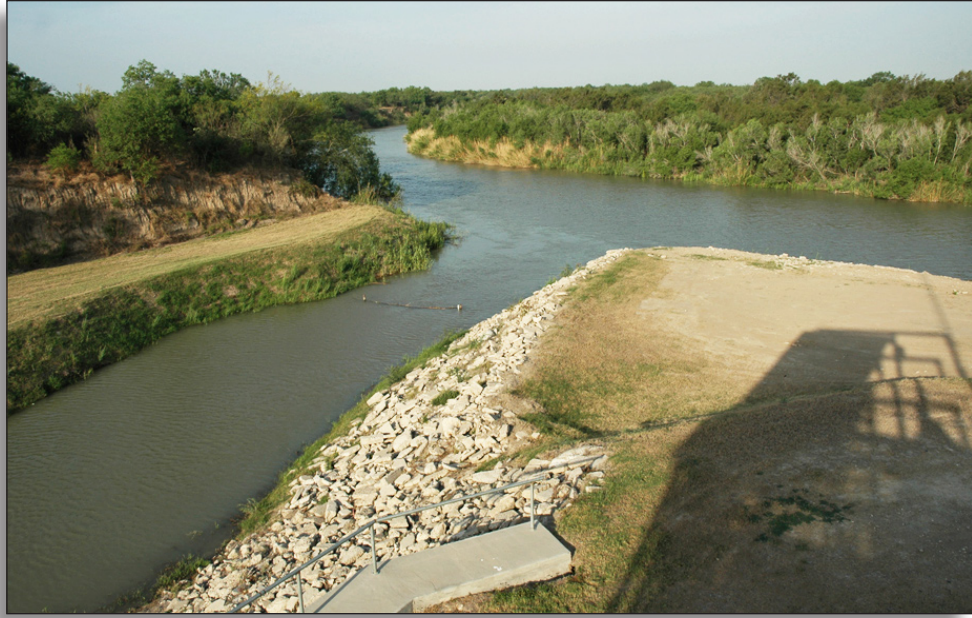
Figure 68: View of inlet channel at Rio Grande River, looking west from first lift pumping station, Hidalgo County Irrigation District No. 3.
