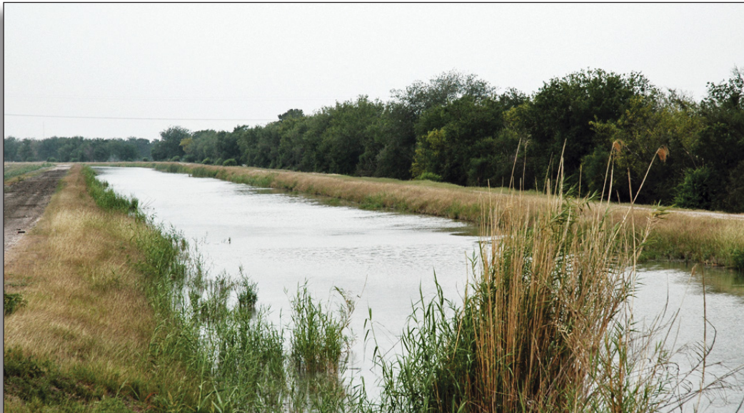
Figure 223: Levee on main canal at IBWC floodgate, United Irrigation District.
