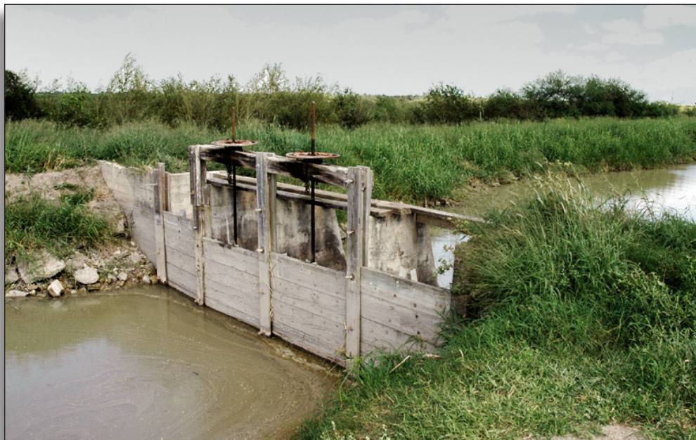
Figure 144: Check gate (1931) near State Fish Hatchery, Cameron County Irrigation District No. 6.
