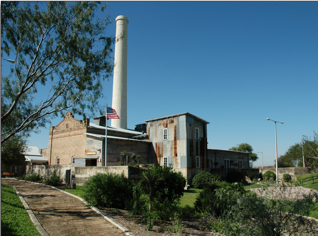
Figure 270: Old Hidalgo Pumphouse, listed in the National Register of Historic Places in 1995.
