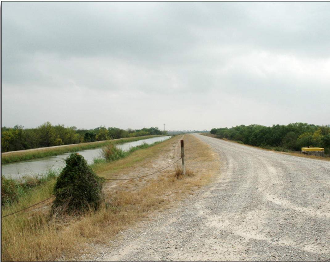
Figure 214: Road atop levee at floodgate, United Irrigation District.
