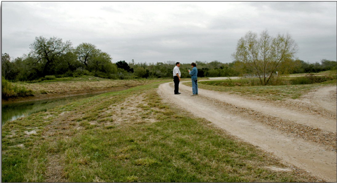
Figure 215: Road adjacent to Edinburg Main Canal, Hidalgo County Irrigation District No. 1.
