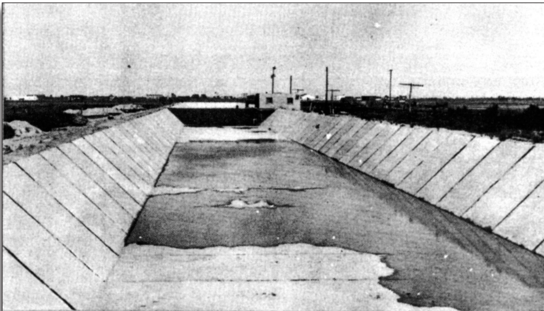
Figure 52: Concrete lining of an unidentified main canal (c.1930). Source: Watson, Lower Rio Grande Valley and Its Builders
