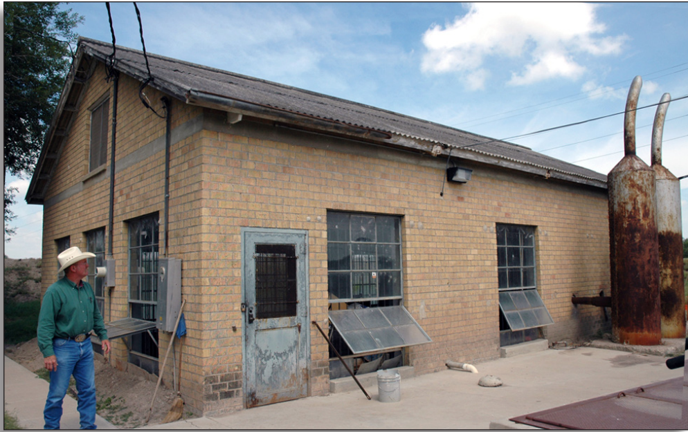
Figure 71: First lift pumphouse (1953), Hidalgo County Irrigation District No. 19.
