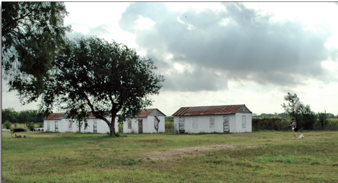
Figure 244: Employee housing (c.1945) behind district office, Santa Cruz Irrigation District No. 15.
