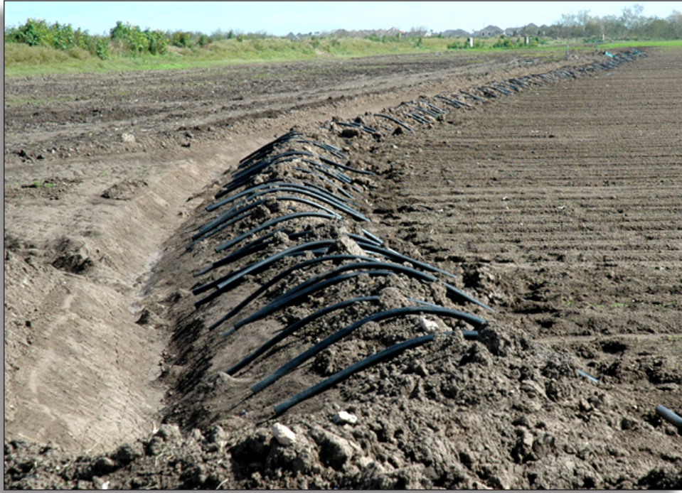
Figure 192: Surface siphon pipes, Hidalgo County Irrigation District No. 1.
