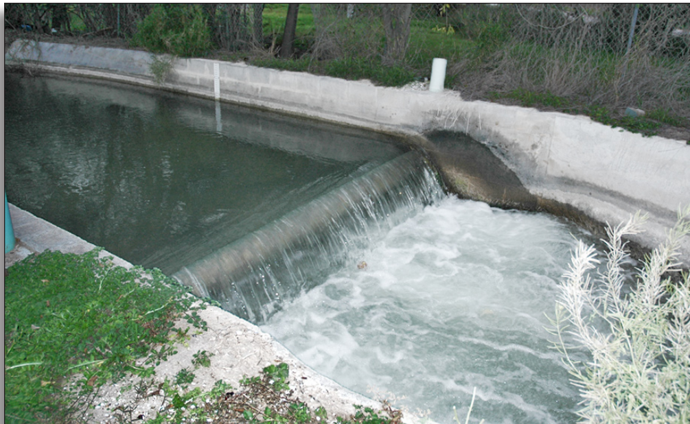
Figure 159: Drop weir, Hidalgo County Irrigation District No. 1.
