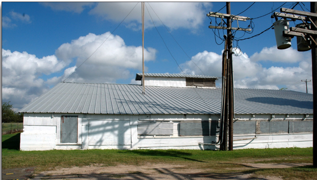
Figure 80: First lift pumphouse (1922), Cameron County Irrigation District No. 6.
