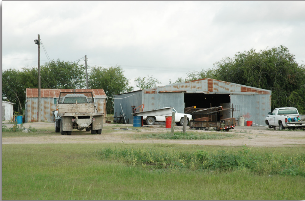
Figure 231: Warehouses (c.1945) at district office, Santa Cruz Irrigation District No. 15.
