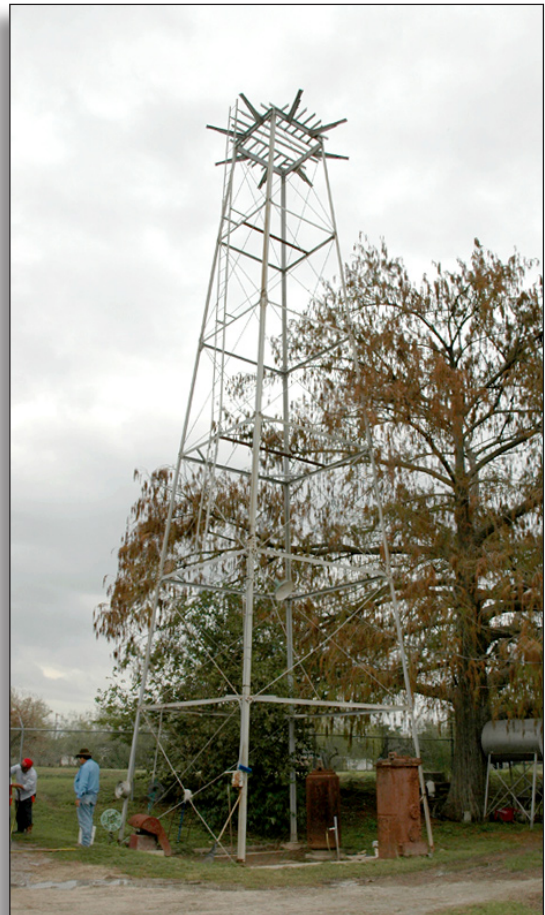
Figure 239: Remains of water tower, first lift station, Hidalgo County Irrigation District No. 1.
