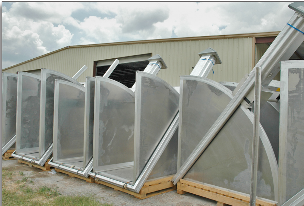
Figure 151: Solar powered, radial head gates (2007) awaiting installation in Cameron County Irrigation District No. 2.
