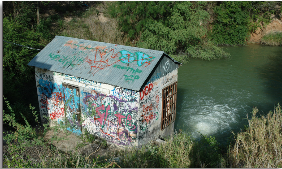
Figure 87: Pump No. 3 (1948), Hidalgo County Irrigation District No. 15.
