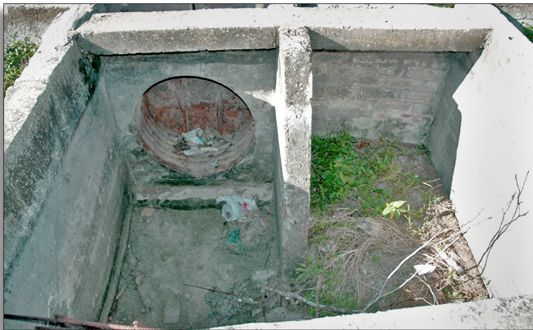
Figure 163: Concrete division box, Cameron County Irrigation District No. 6.
