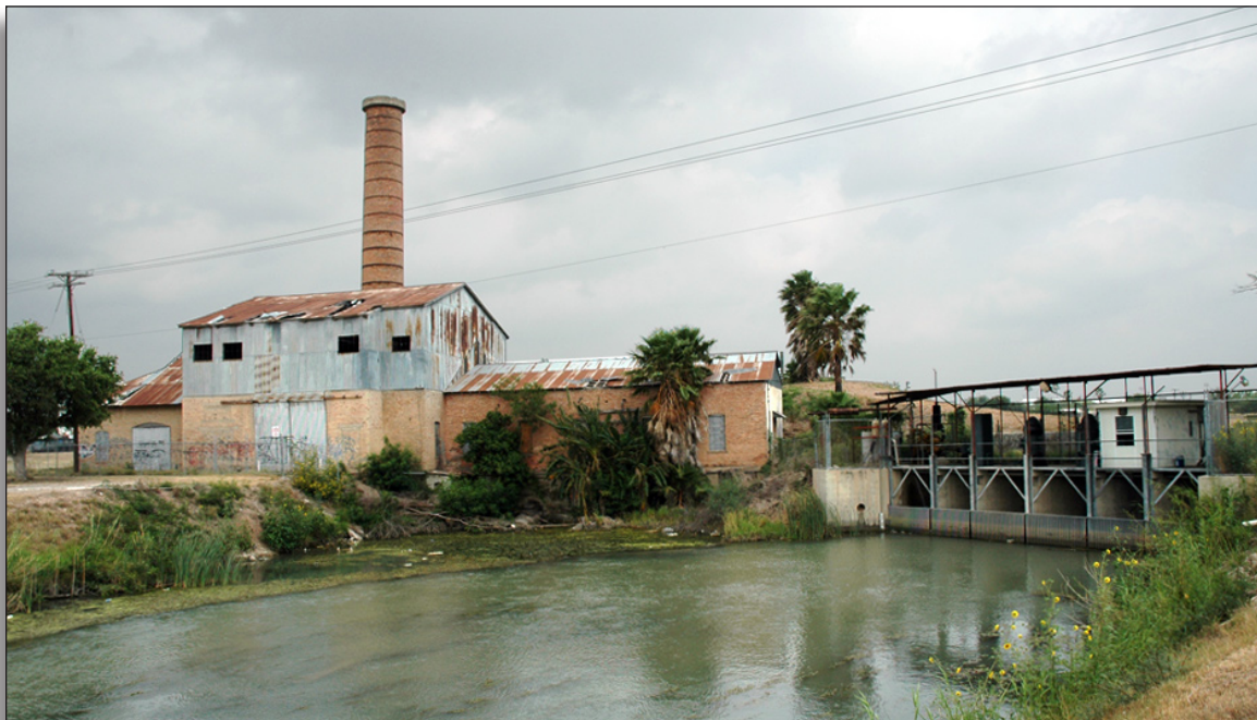
Figure 283: Integrity of design impacted by the new second pumping plant (right) next to the old second pumping plant (left, no longer in service), United Irrigation District.
