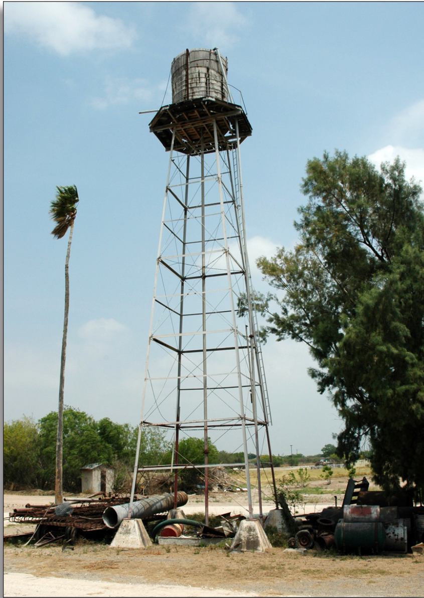
Figure 237: Water tower, old third lift pumping plant, United Irrigation District.
