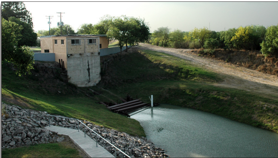
Figure 72: Old first lift pump house (1921) and inlet channel, Hidalgo County Irrigation District No. 3.
