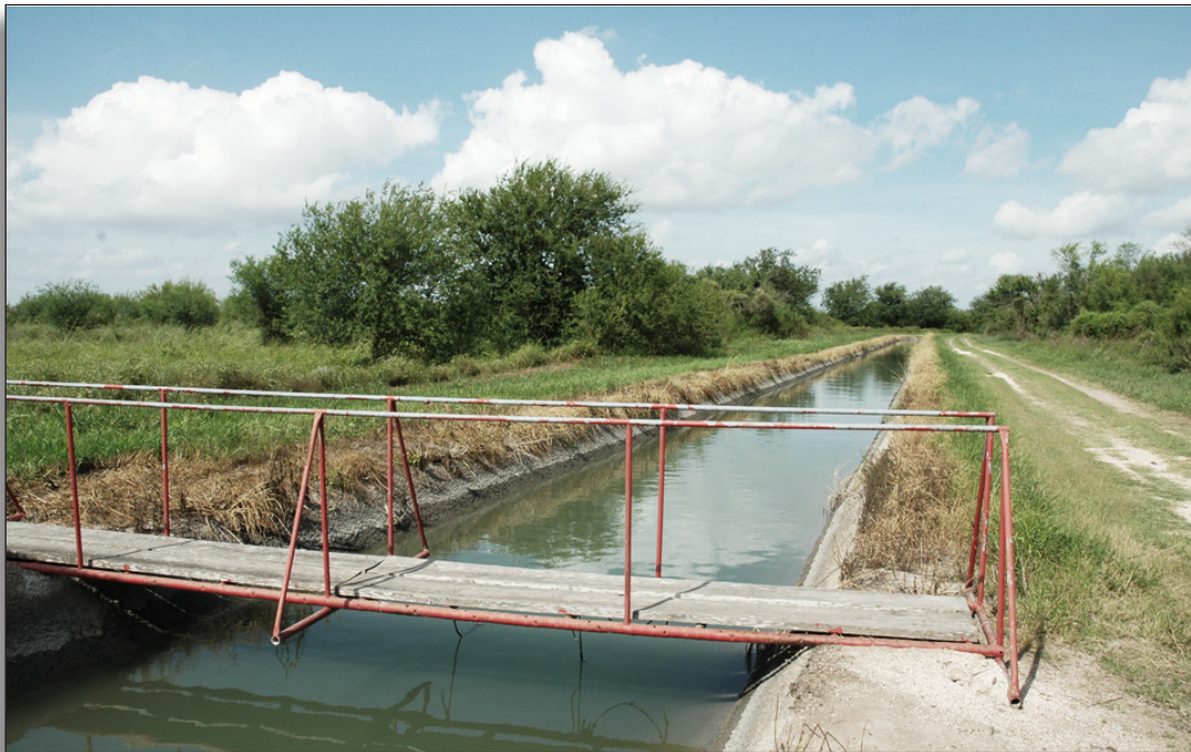
Figure 213: Pedestrian bridge (c.1956) at Pump No. 16, Santa Cruz Irrigation District No. 15.
