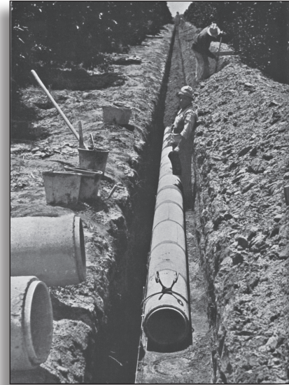
Figure 136: Laying concrete pipe. Source: Loving, Concrete Pipe for Irrigation and Drainage
