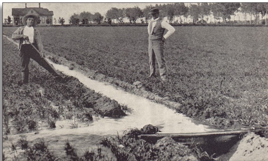
Figure 204: Water distribution from ditch to field employing temporary dam (1902). Source: Newell, Irrigation in the United States
