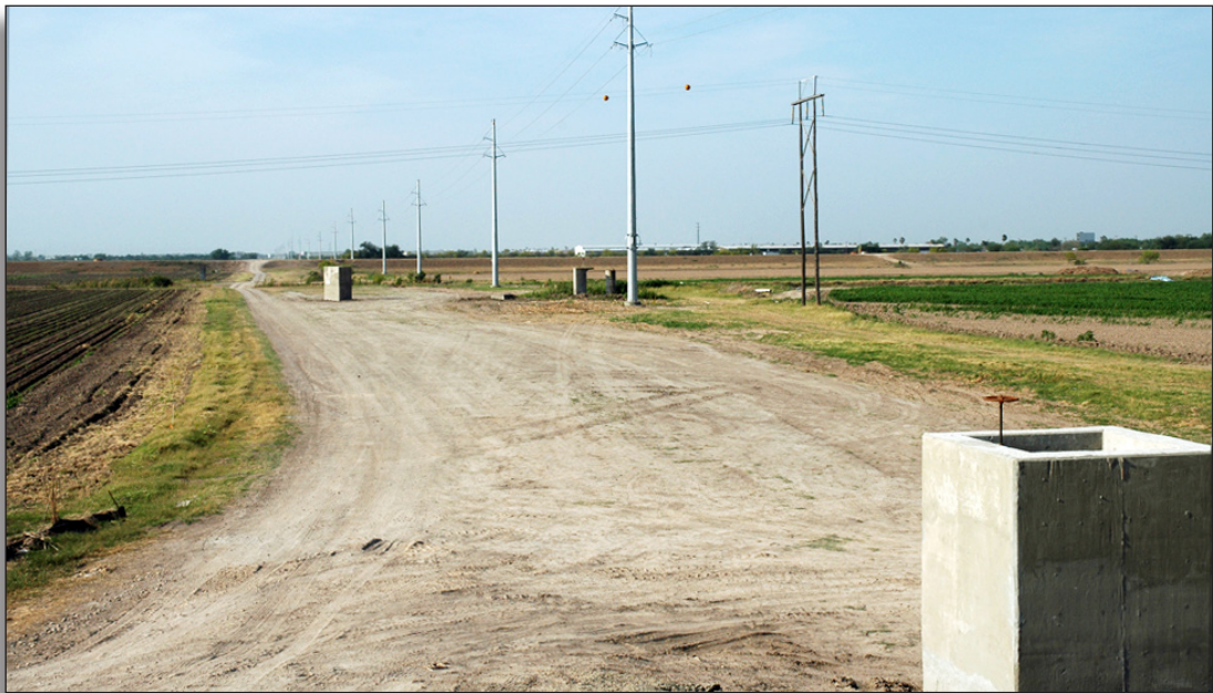
Figure 216: Service road adjacent to new underground siphon across floodway, Hidalgo County Irrigation District No. 3.
