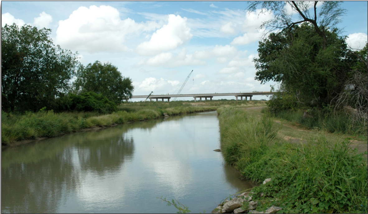
Figure 277: New alignment (1974) of the main canal for Hidalgo County Irrigation District No. 19.
