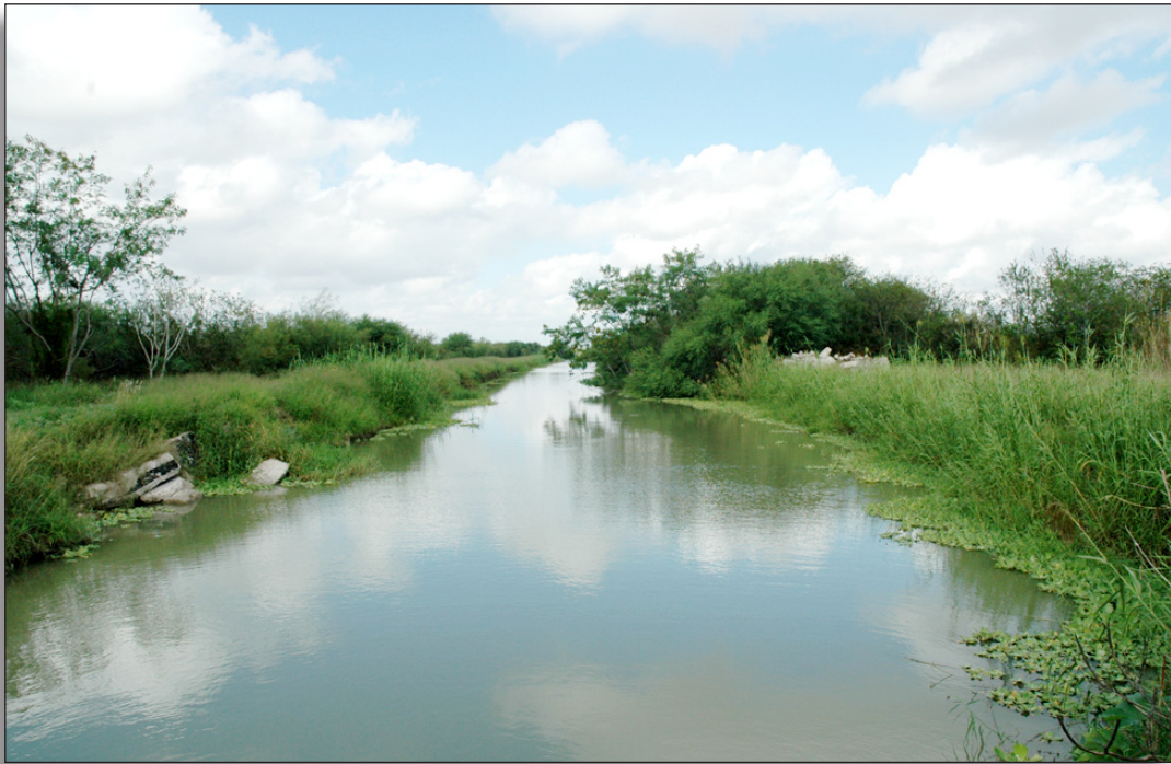
Figure 269: Main canal, Cameron County Irrigation District No. 6.
