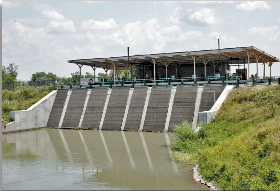
Figure 81: New pumping plant, Cameron County Irrigation District No. 2 (2005).
