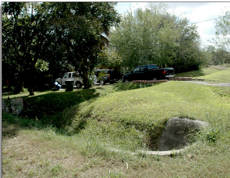
Figure 188: Sub-lateral of Stub-Tandy Lateral Canal, Cameron County Irrigation District No. 6.
