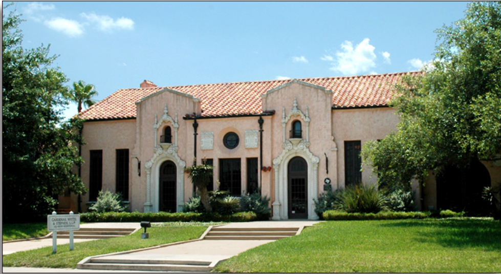
Figure 258: The old Southern Pacific Railroad Depot in McAllen opened for service in August 1927.
