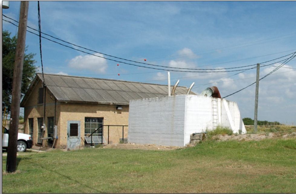
Figure 94: Surge box (1953) at river pumping plant, Hidalgo County Irrigation District No. 19.
