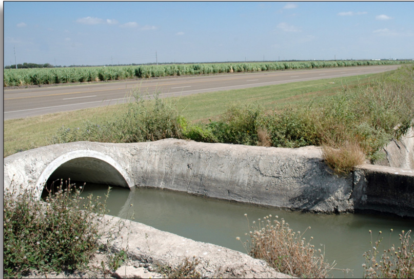
Figure 130: Siphon at Samuelson Canal (c.1985), Hidalgo County Irrigation District No. 19.
