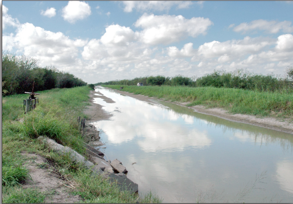
Figure 112: Northwest view of main canal (c.1914), Cameron County Irrigation District No. 6.
