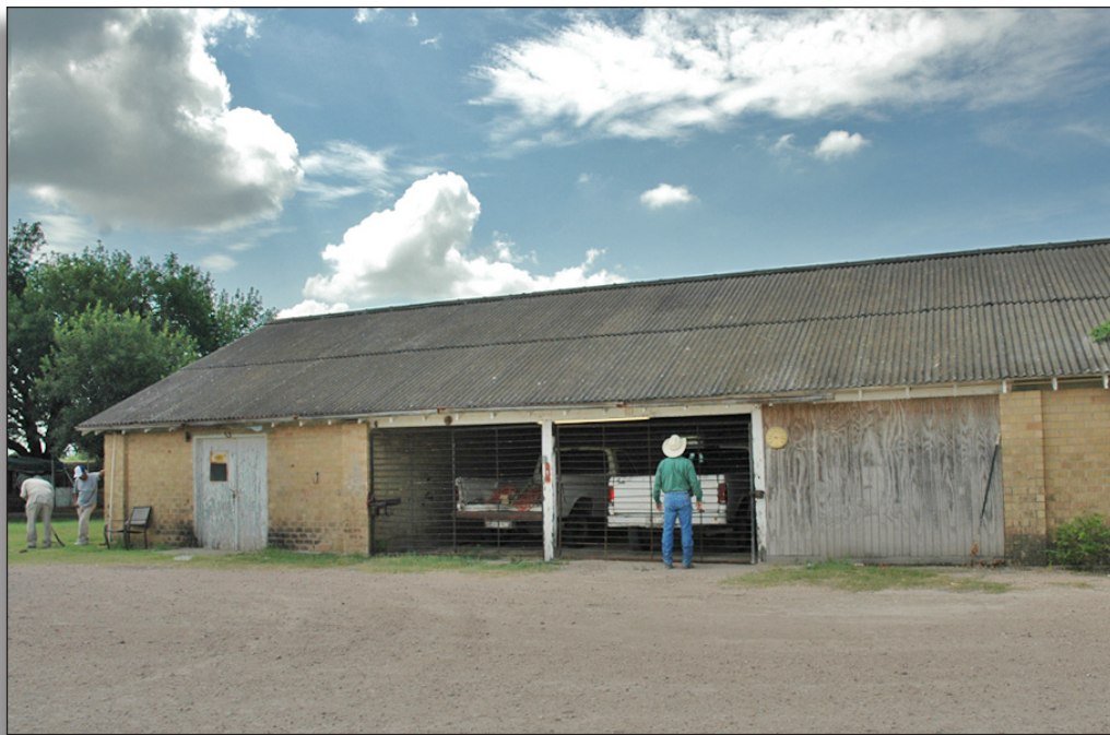
Figure 232: Warehouse (1953) at pumping plant, Hidalgo County Irrigation District No. 19.
