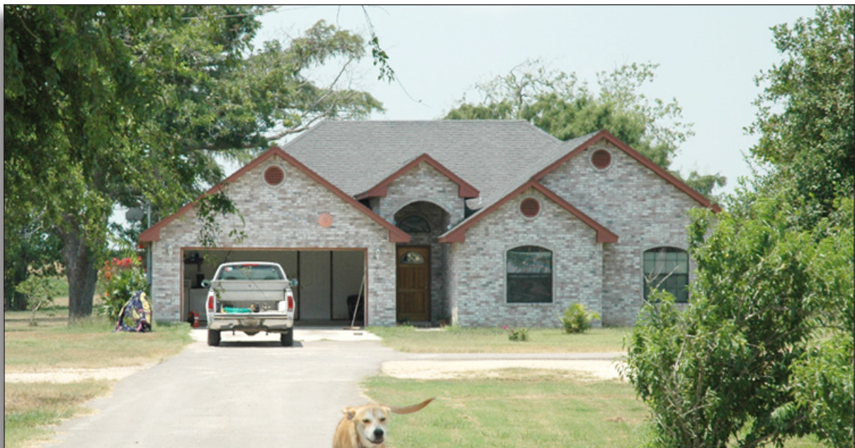
Figure 241: New employee housing at new pumping plant, Los Indios, Cameron County Irrigation District No. 2.
