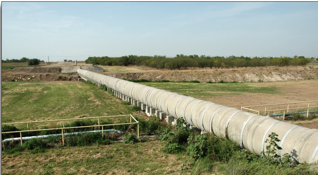
Figure 129: Flume over main floodway channel (1984), Hidalgo County Irrigation District No. 3.
