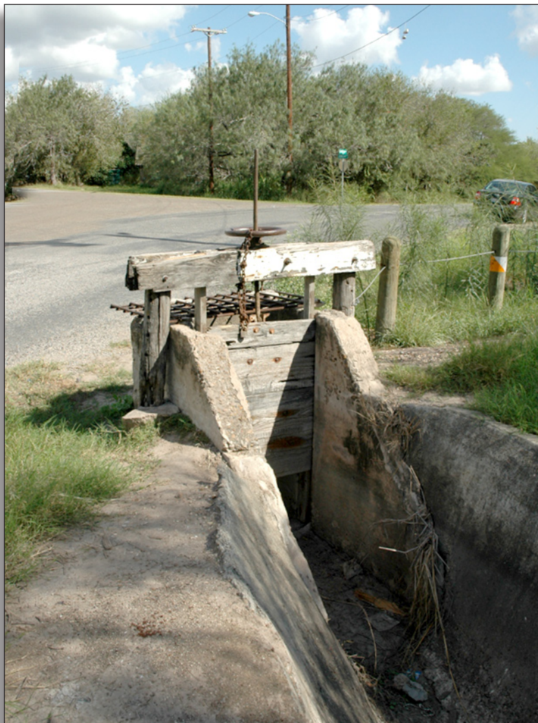
Figure 149: Head gate on Stub Canal, Cameron County Irrigation District No. 6.
