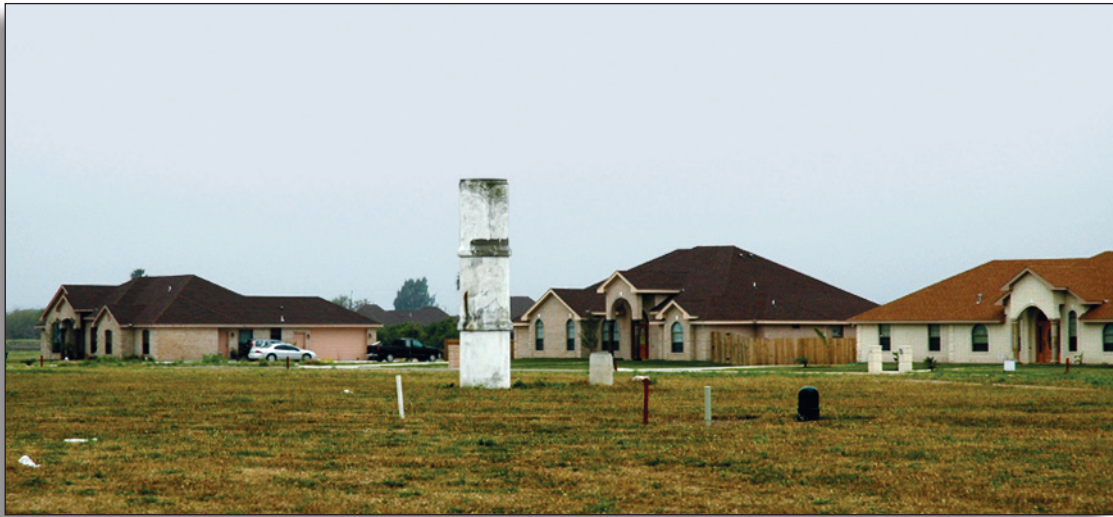
Figure 308: This stand pipe in new subdivision demonstrates a loss of feeling due to its loss setting and association, Hidalgo County Irrigation District No. 1.
