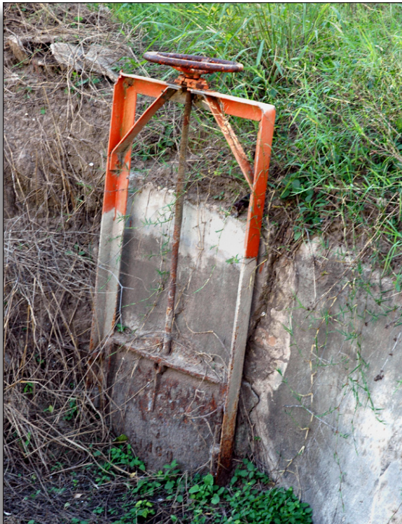
Figure 153: Modern slide gate (c.1950), Cameron County Irrigation District No. 6.
