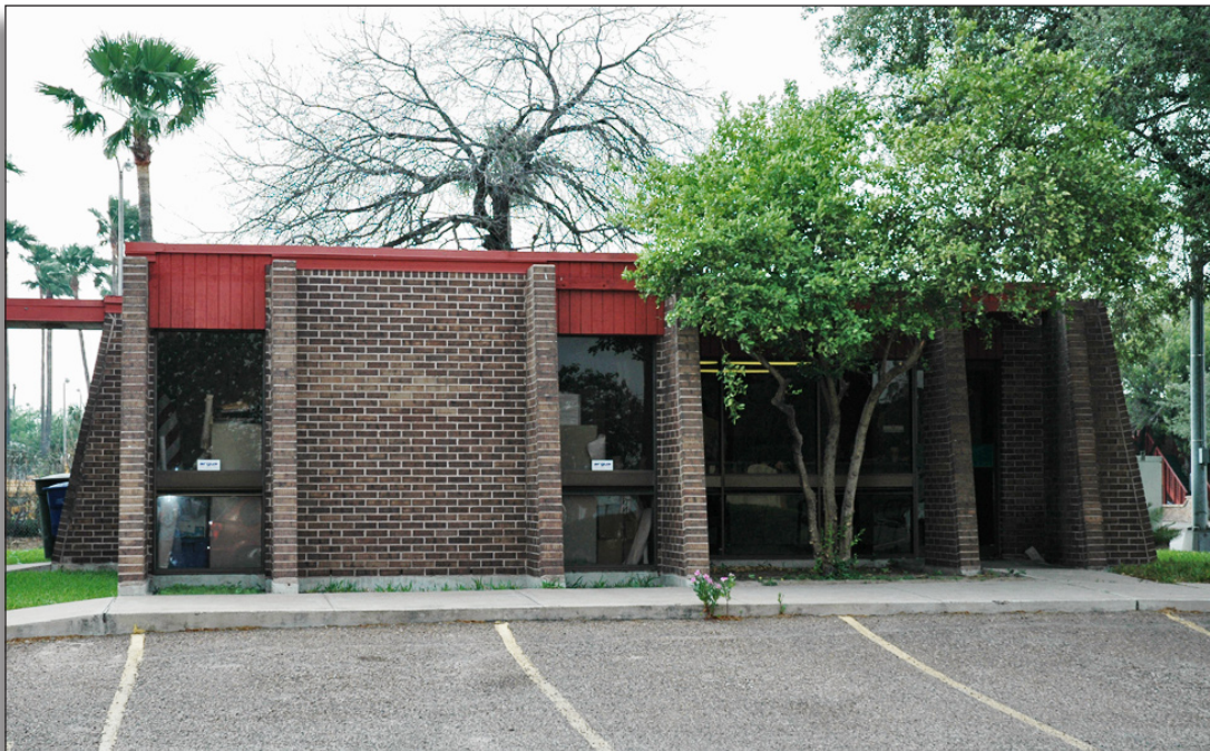
Figure 224: Offices (1974) of Hidalgo County Irrigation District No. 3, 1325 Pecan Street, McAllen.
