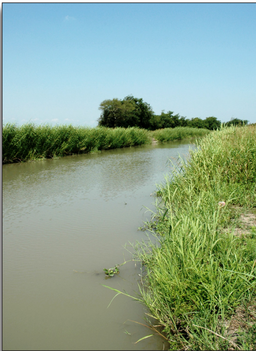
Figure 102: Earthen main canal, Cameron County Irrigation District No. 2.
