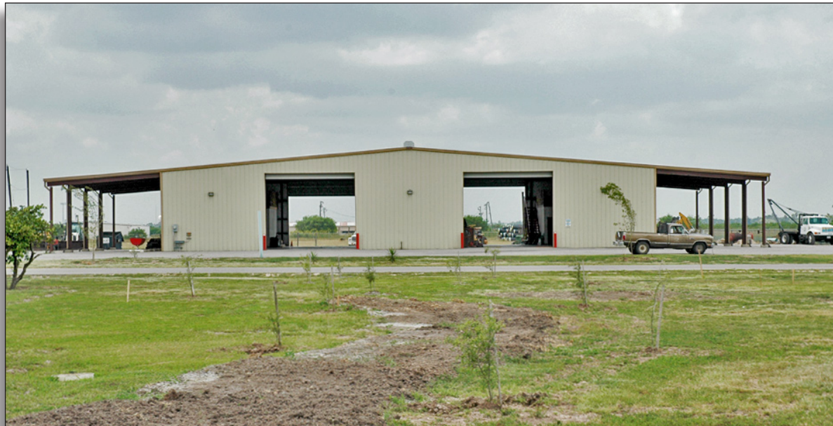
Figure 230: Warehouse at district office located off FM 510, San Benito, Cameron County Irrigation District No. 2.
