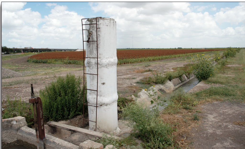
Figure 177: Diversion stand (1962) to Bodine Lateral along FM 494, Hidalgo County Irrigation District No. 19.
