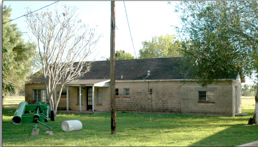
Figure 240: Employee residence at second lift plant, Cameron County Irrigation District No. 6.
