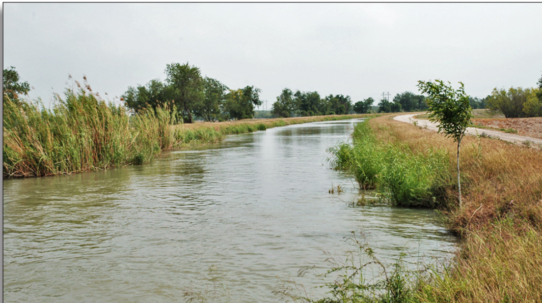
Figure 113: Main canal (1960) at first lift pumping plant, United Irrigation District.
