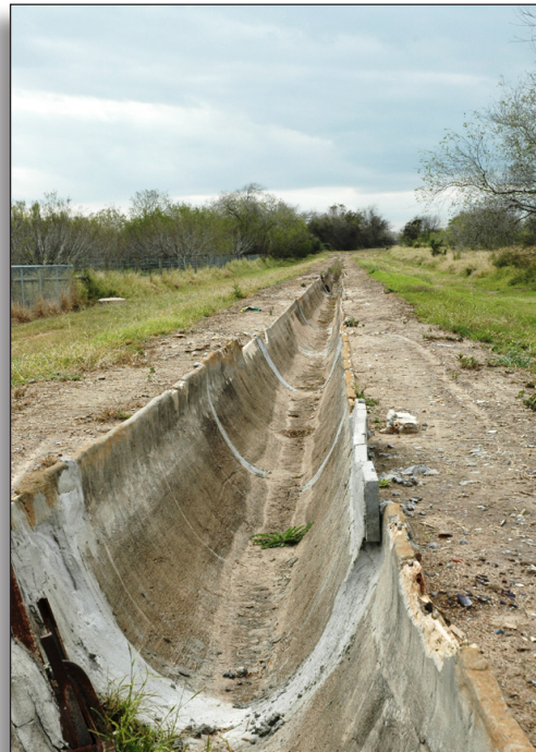
Figure 106: Concrete lined canal (1927), Hidalgo County Irrigation District No. 1.
