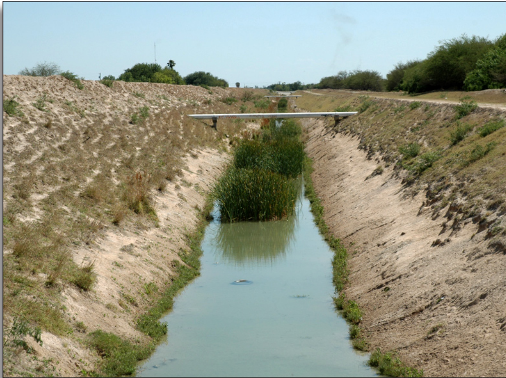
Figure 219: Drainage ditch along Main Canal, Mile 6 North Road, United Irrigation District.
