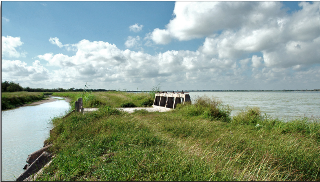
Figure 313: The reservoir and diversion gate retain integrity of both feeling and setting, Cameron County Irrigation District No. 6.
