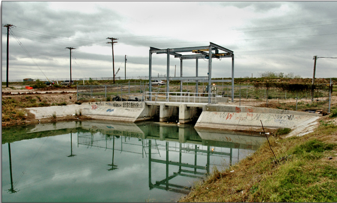
Figure 287: Design of the first check gate on Edinburg Main Canal is a state-of-the-art example of modern irrigation technology that impacts the overall design, Hidalgo County Irrigation District No. 1.
