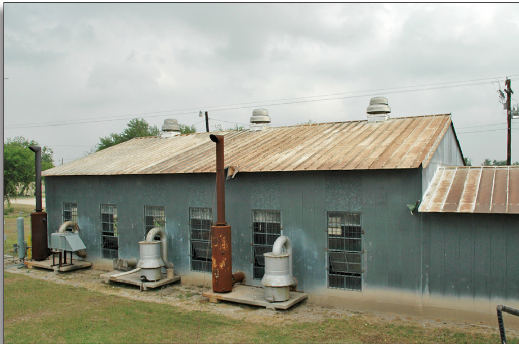
Figure 70: First lift pump station, United Irrigation District.
