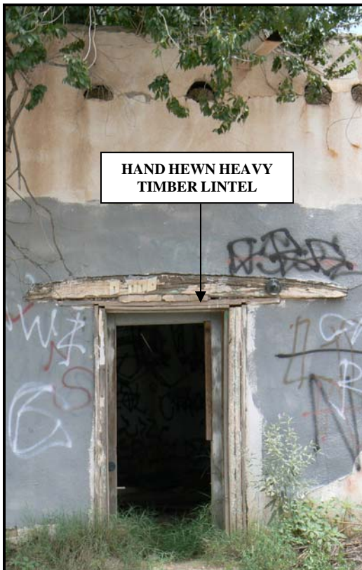
San Elizario, circa 1870. Hand-hewn window and door frame materials suggest that the building is adobe. Source: Baker, 2008.
