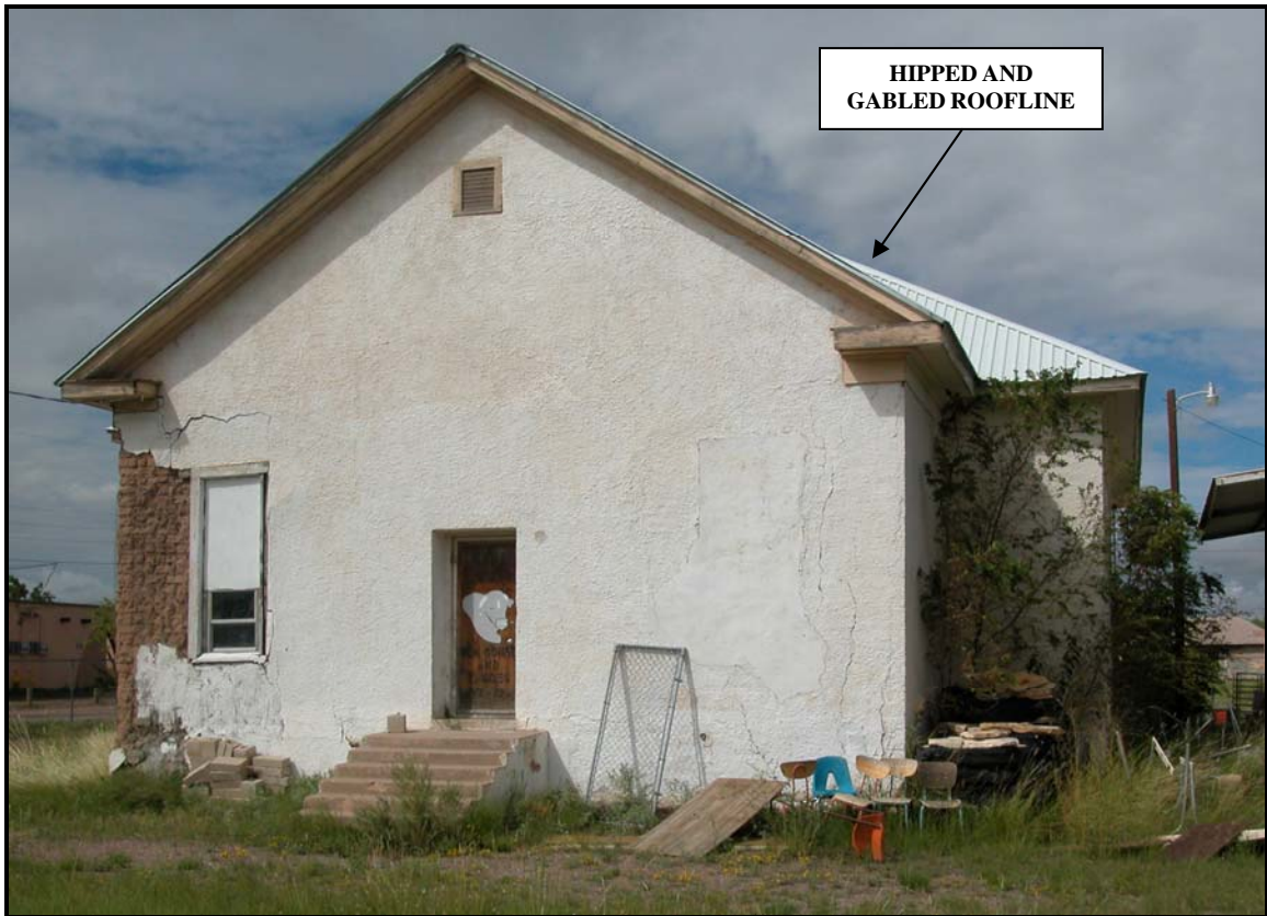
Circa 1910 adobe school in Marfa. Pitched rooflines were not commonly used on adobe buildings before the early 20 th century. Source: Preservation Central, Inc., 2007.
