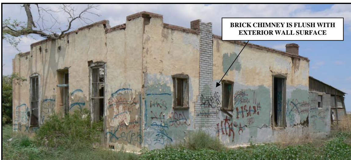
Circa 1900 dwelling in Socorro, Texas. The brick chimney is flush with exterior wall surface. Source: Baker, 2008.
