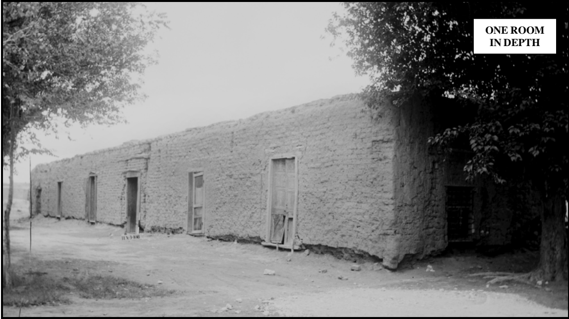
Jesus Lujan House, erected in San Elizario, Texas circa 1850. The building demonstrates the linear, single-file floor plan typical of early adobe architecture. Source: Library of Congress, Prints & Photographs Division, HABS TEX, 71-SANEL, 3- 1936.
