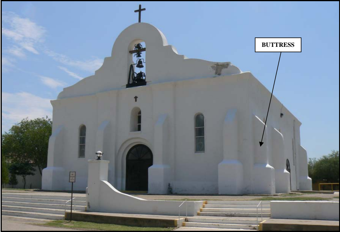
San Elizario Chapel, San Elizario, Texas. This circa 1870 adobe chapel has massive buttressing. Source: Baker, 2008.
