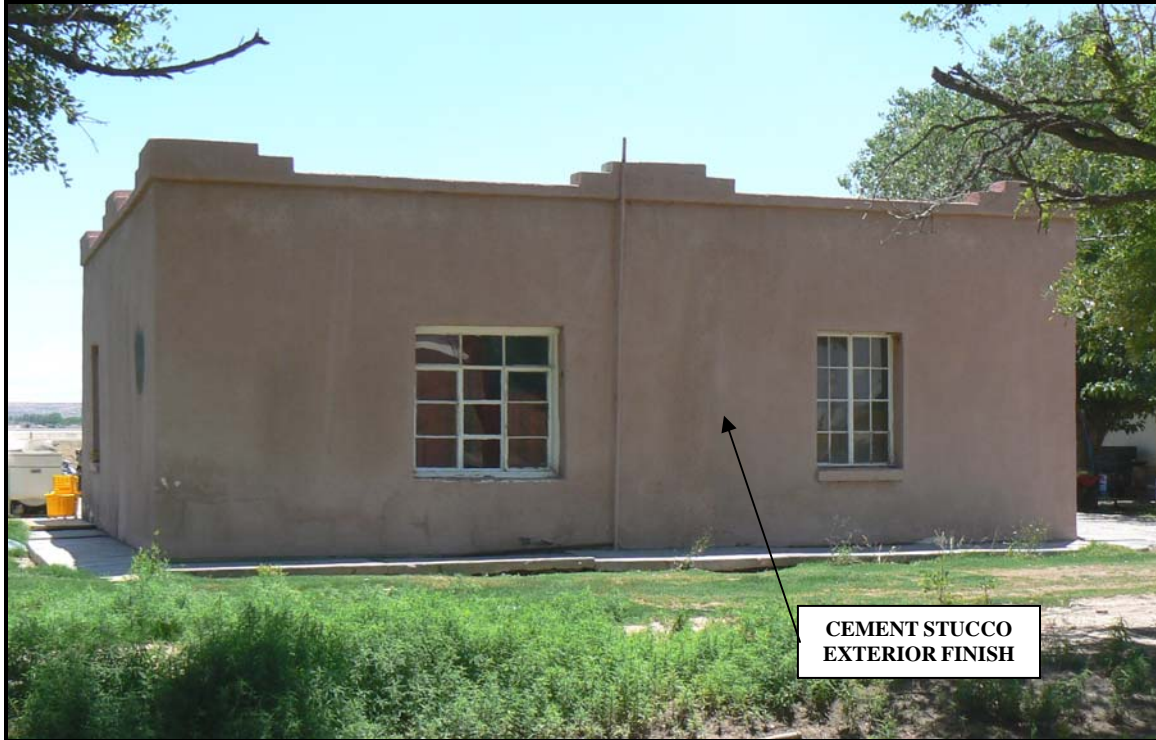
El Paso, Texas. A circa 1940 adobe building is covered with cementitious stucco. Source: Baker, 2008.
