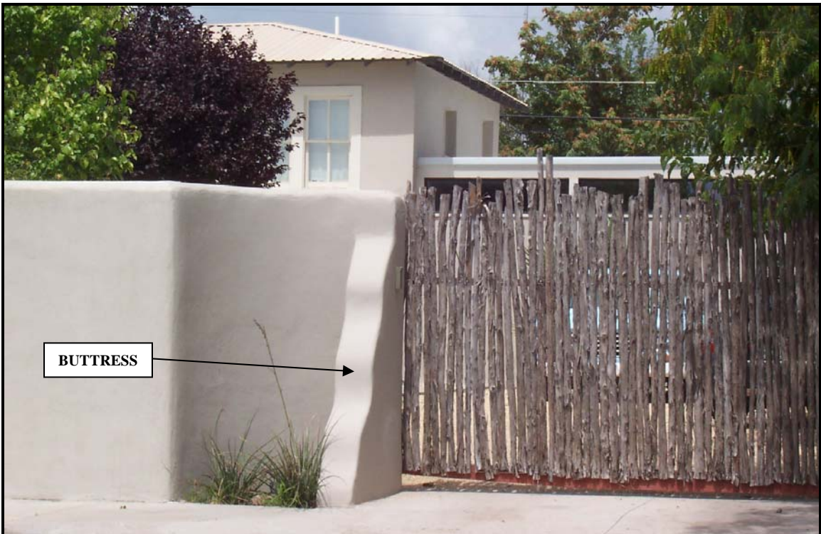
Newly constructed free-standing adobe wall in Marfa, Texas, with buttressing. Source: Preservation Central, Inc., 2007.
