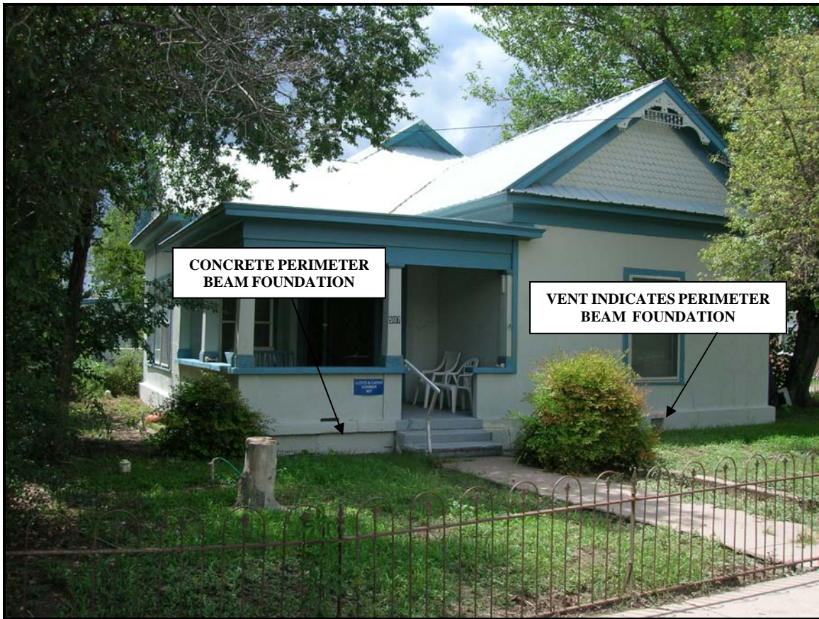
Circa 1915 adobe house in Marfa, Texas. Concrete perimeter beam foundation. Source: Preservation Central, Inc., 2007.
