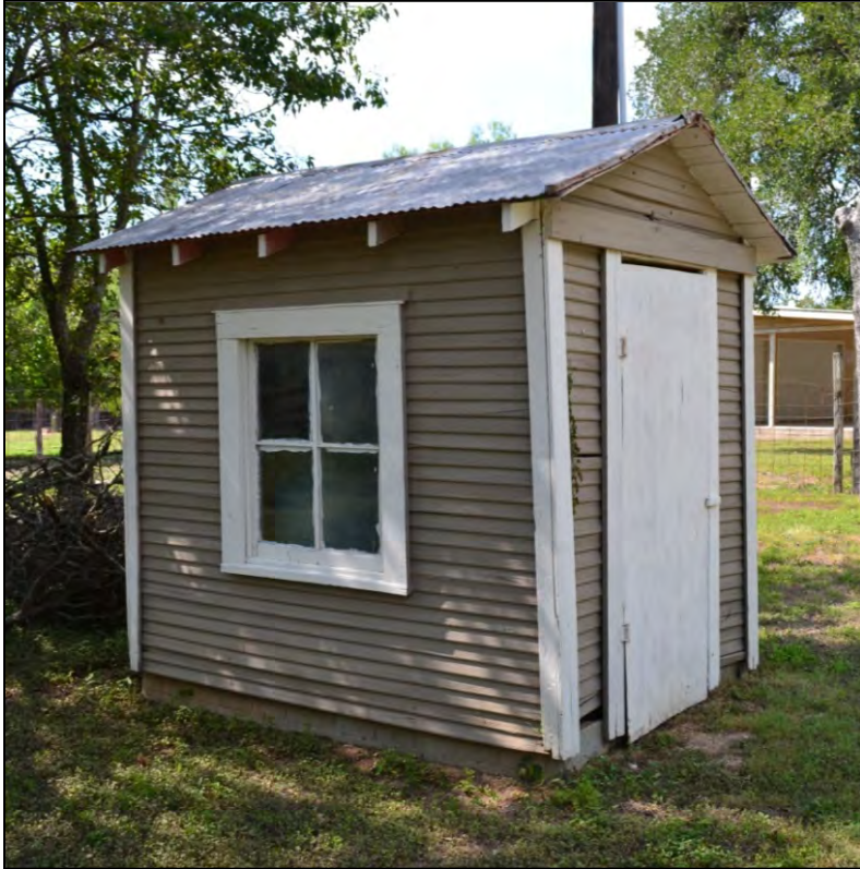
Figure 5-11. Ca. 1920 timber-frame domestic shed. It consists of horizontal wood siding, a fixed-sash multi-glazed window, gabled metal roof with exposed eaves, and a plywood door.
