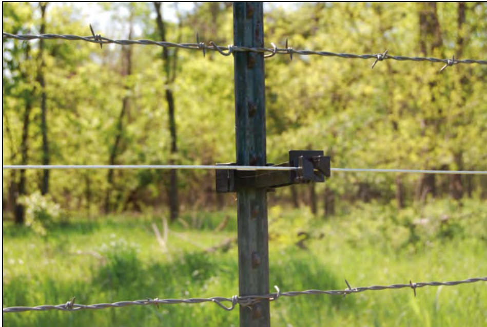
Figure 5-69. Detail of electric fence with electrified wiring in the middle between the barbed wire strands. Source: www.patriotglobal.com .
