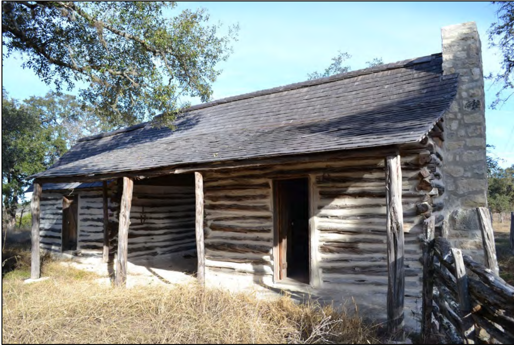
Figure 6-34. Photo of a ca. 1850 house in Comal County. This house exhibits the use of indigenous materials, including native wood and locally quarried stone that is typical from the pre-railroad area in Central Texas. (Source: Comal County Historical Commission.)
