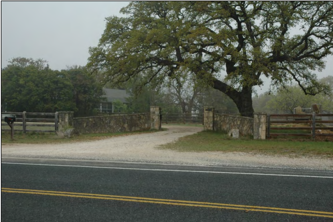
Figure 5-33. Main entrance gate with masonry walls and piers and wooden fencing.
