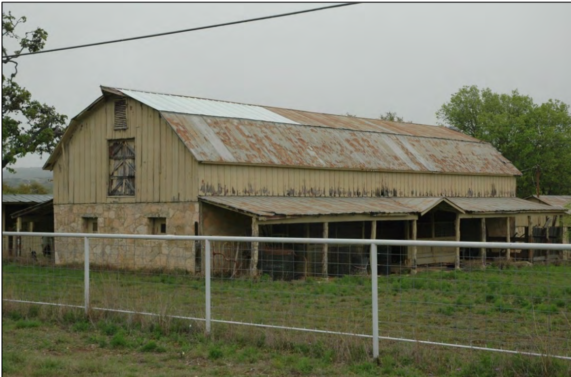
Figure 5-42. Gambrel roof side-entry dairy barn. The barn exhibits masonry and wood construction, a hay door with hay roof, small square windows for light and ventilation, and a timber frame shed roof side room.
