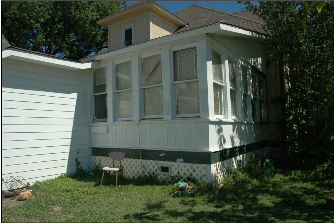
Figure 7-24. Sunroom addition on southwest façade of main house (ID a), constructed ca. 1940.
