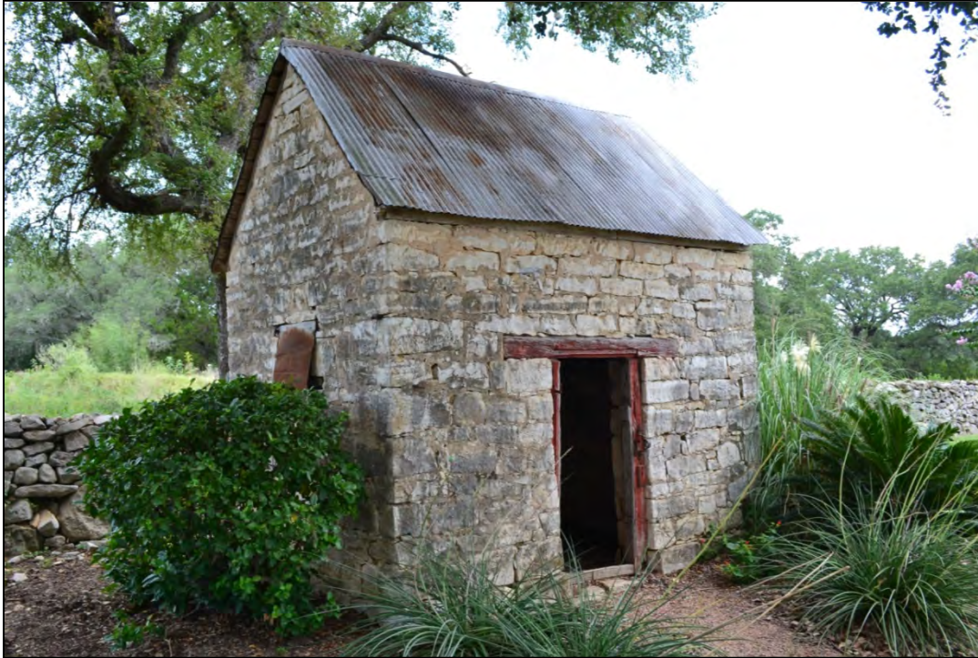
Figure 5-25. Ca. 1880 smokehouse. The building exhibits masonry construction with a corrugated metal roof and a small opening on the gable-end for ventilation.
