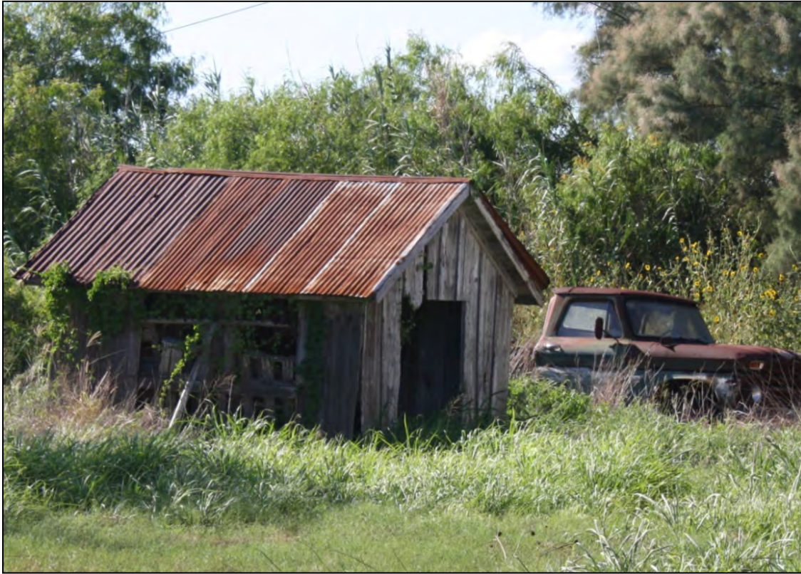
Figure 5-12. Ca. 1920 domestic work shed with gable roof and wood siding.
