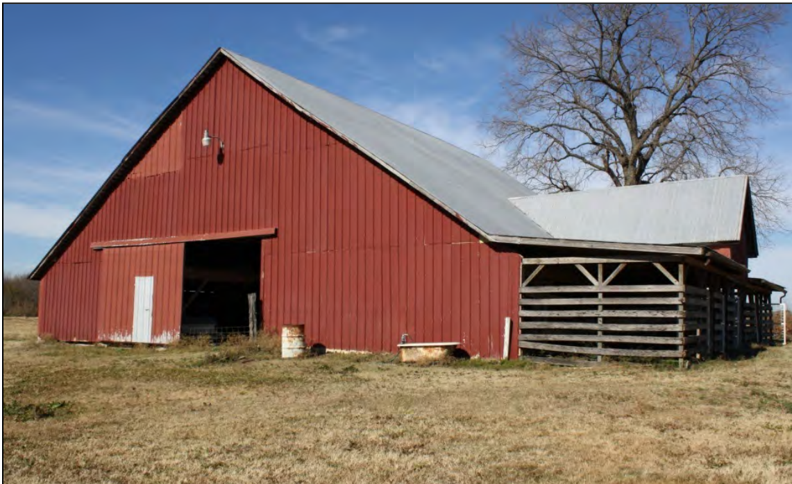
Figure 5-40. Transverse general purpose barn with attached livestock pens. Barn exhibits vertical wood siding with a sliding door and capped with a gabled metal roof.
