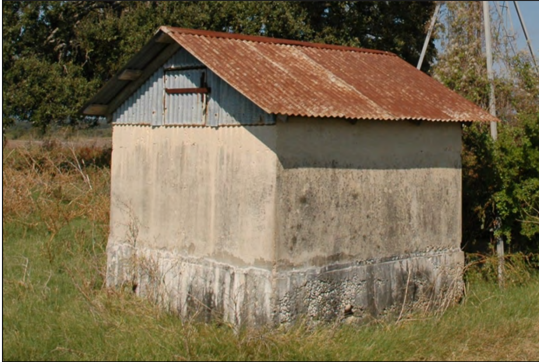
Figure 5-19. This well house is located adjacent to a windmill. The concrete well house was built ca. 1925 and is topped with a gable corrugated sheet metal roof.
