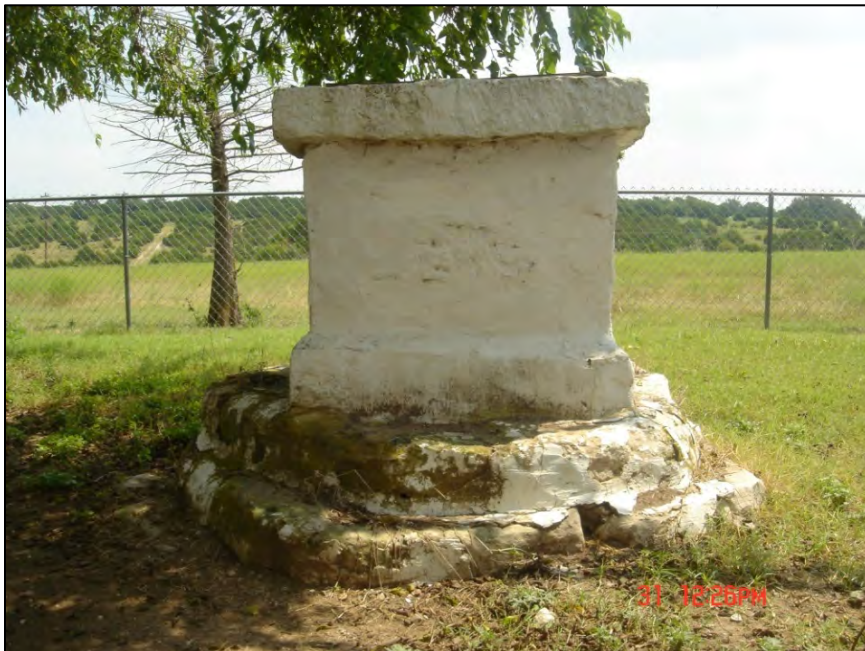
Figure 6-6. View of the cistern on the Bryson farmstead. It is located at the southeast corner of the main house and is considered contributing to the historic farmstead. According to Section 5, Property Types, cisterns are commonly located near the main house and early examples are usually of masonry construction. In later years, many agriculturalists constructed raised cisterns that rested on wooden supports. (Source: TxDOT.)
