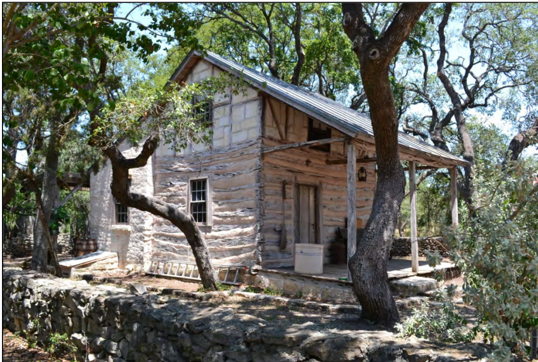
Figure 5-5. Ca. 1850 one-and-a-half side-gable residence with stone rear-shed addition. Fachwerk is on the upper-half of the gable section with its timber framing and vertical and diagonal bracing.
