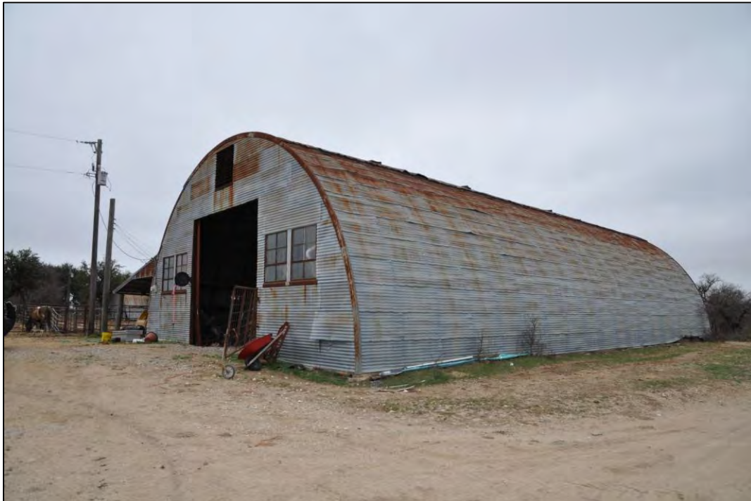
Figure 5-44. Ca. 1950 Quonset hut. Source: TxDOT Environmental Affairs Division.
