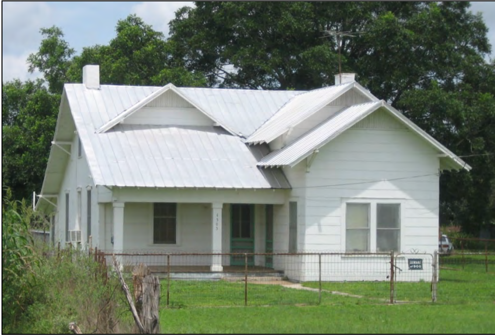
Figure 5-6. Ca. 1920 two-story, cross-gable residence with modest Folk Victorian and Craftsman style influences, indicating that the house may have been remodeled after its initial construction. Folk Victorian features include window hoods and six-over-six double-hung windows on the porch and side-gable end. Craftsman features include low-pitched roof, exposed eaves, and square columns supporting a wide unornamented entablature.
