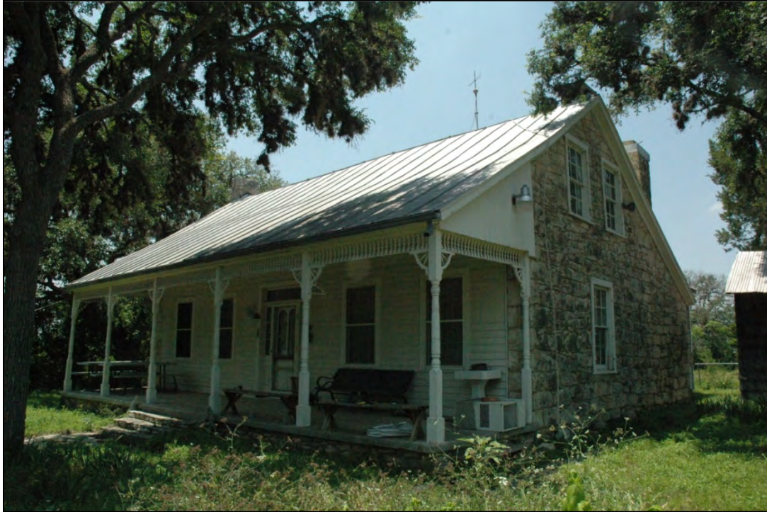
Figure 5-4. This main house is a two-story, side-gable Folk Victorian residence located in Central Texas. Built ca. 1890, the main house exhibits stone and timber construction topped with a metal roof. Distinctive features include spindlework detailing on the full-width porch, six-over-six double-hung windows, and glazed paneled front door with sidelights and transom.
