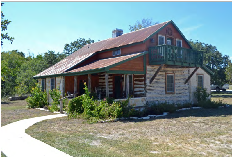
Figure 6-14. View of single-family dwelling in Comal County. This building has been modified with the addition of a second story, second floor balcony, multiple additions, and replacement windows. As such, it does not retain sufficient integrity of materials and design to illustrate the craftsman's skills and talents, and, therefore, has lost its integrity of workmanship. (Source: Comal County Historical Commission.)
