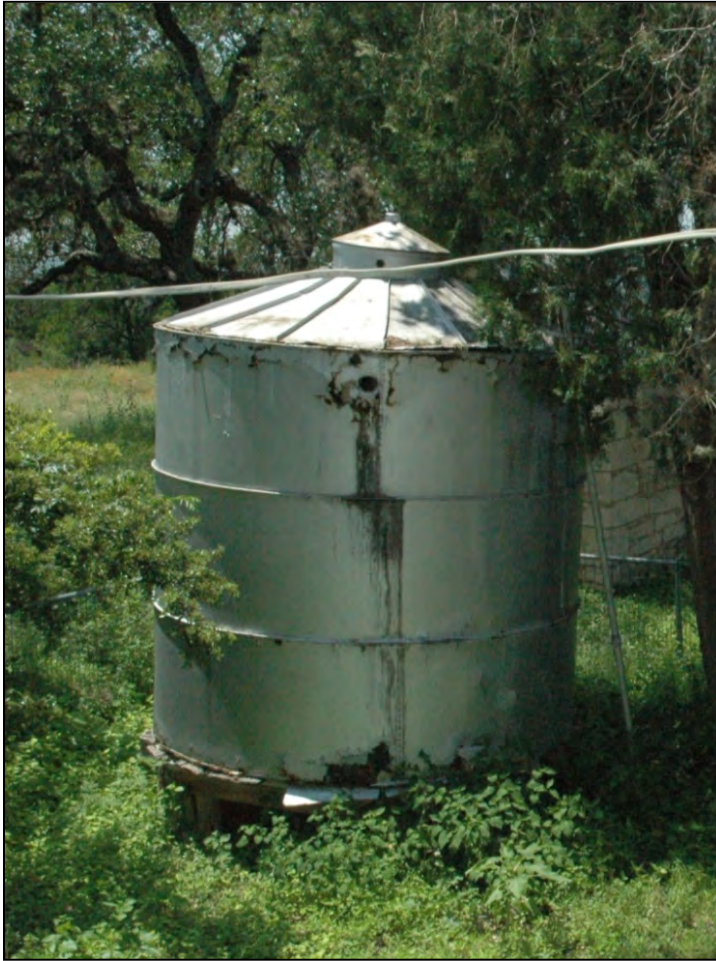
Figure 5-14. Ca. 1925 metal cistern elevated off the ground by wooden supports.
