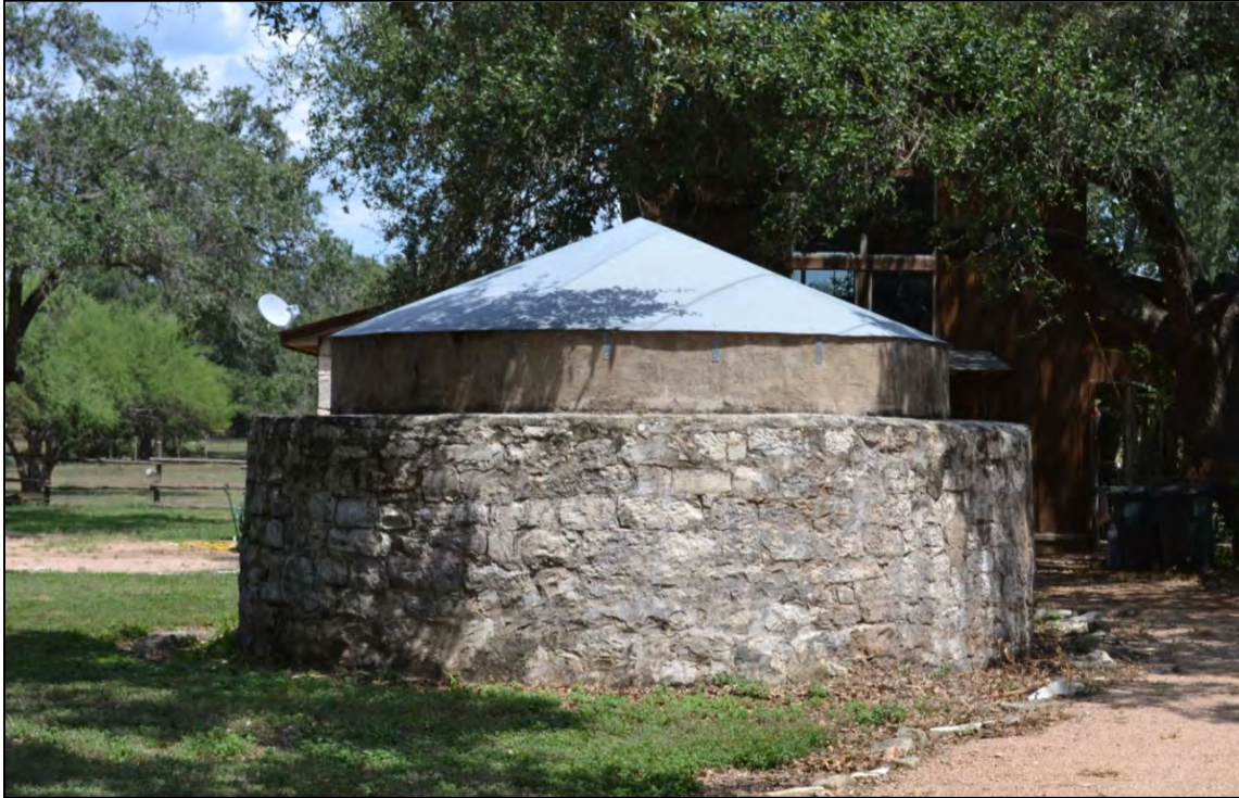
Figure 5-13. Above-ground stone cistern.
