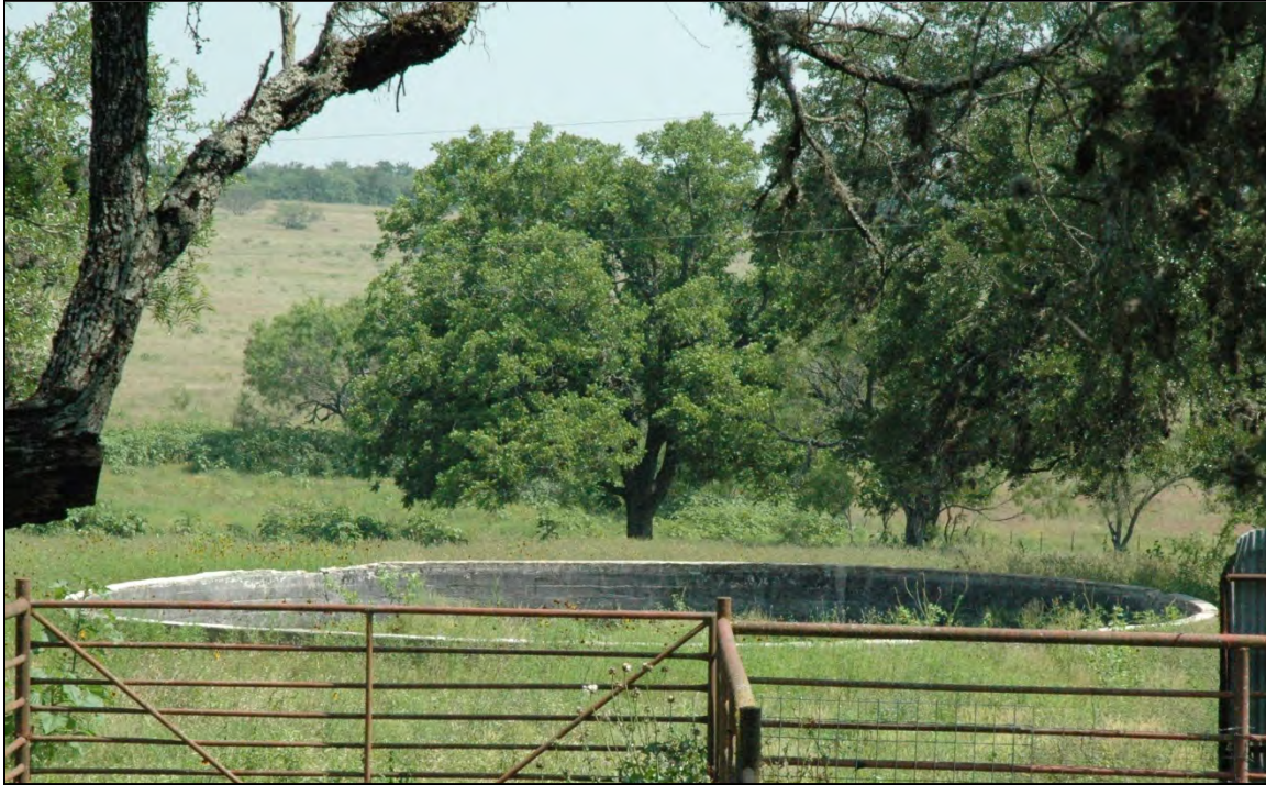
Figure 5-55. Concrete stock tank adjacent to corrals.
