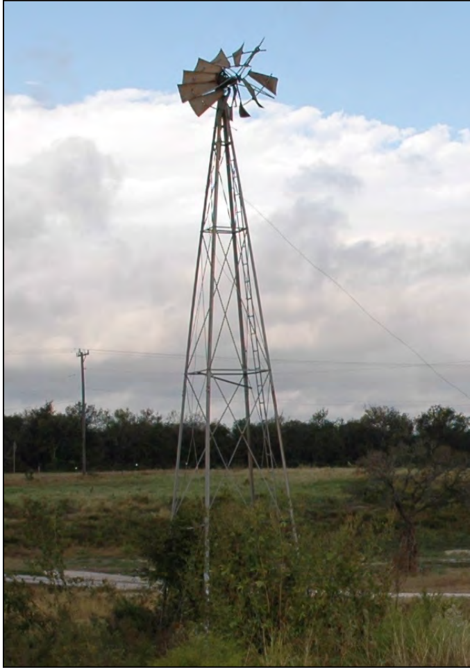
Figure 5-17. This photo shows a windmill with damaged metal rotating vanes and metal tower.
