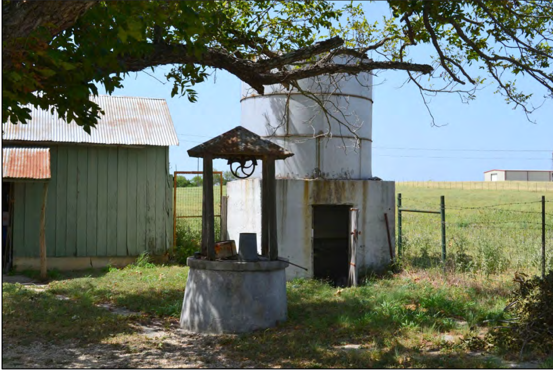
Figure 5-16. This well has a pyramidal covering with a pulley system to retrieve water; note the cistern adjacent to it.
