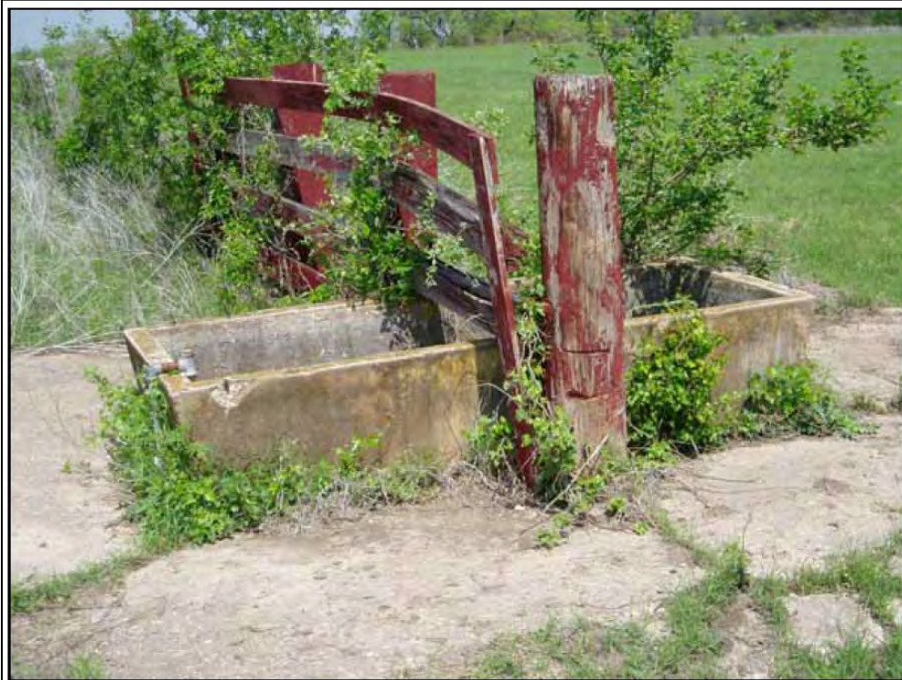
Figure 7-10. Resource ID No. 23j was one of two concrete water troughs recorded on the agricultural property. The portion of fencing that remained allowed livestock to have access to water from two adjacent enclosed pastures.
