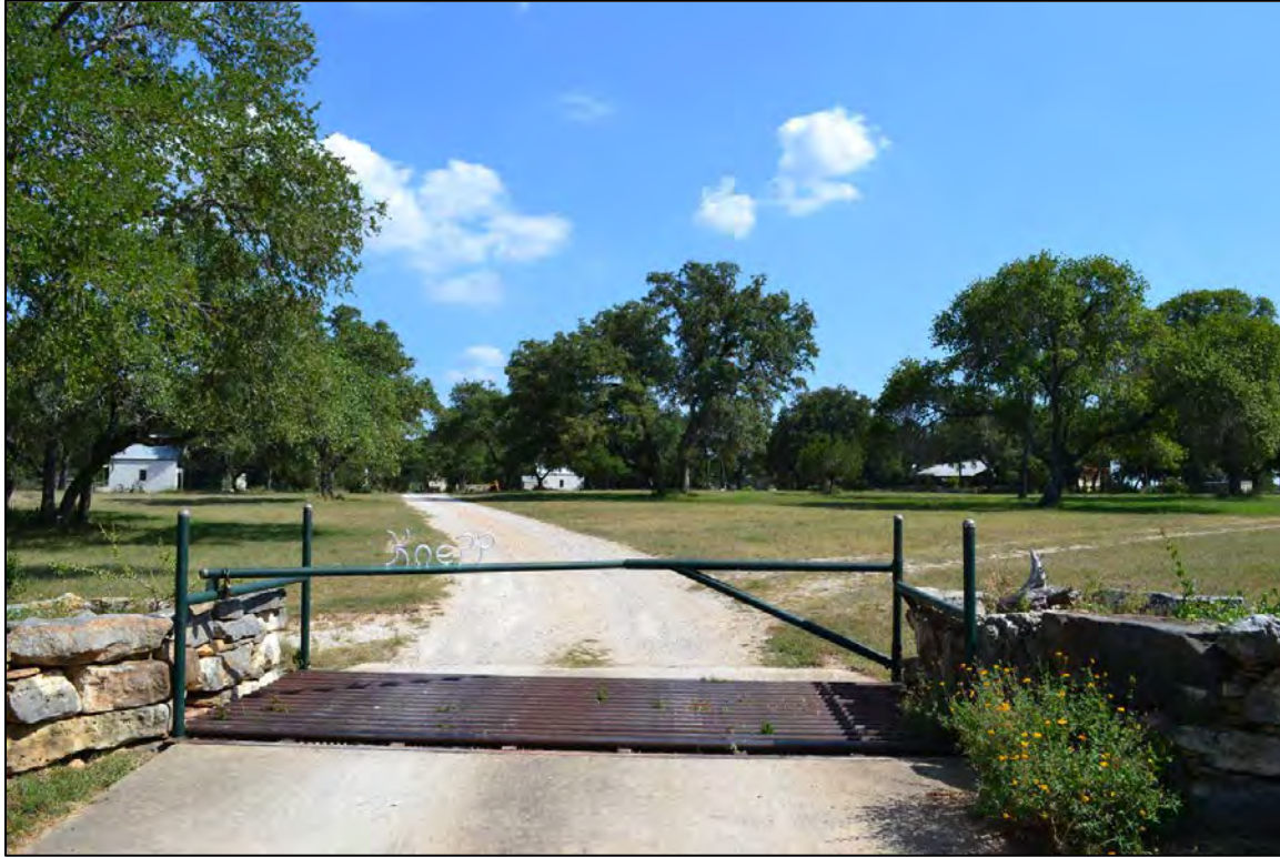
Figure 5-70. Cattle guard at the entrance to a property.
