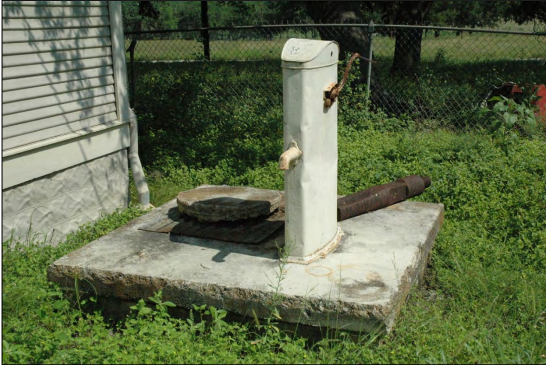
Figure 5-15. This concrete well was constructed ca. 1920 and is topped with a concrete cap and metal hand crank.
