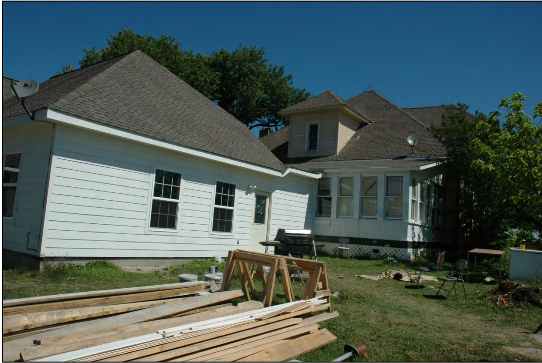
Figure 7-26. Rear addition, constructed in 2008.
