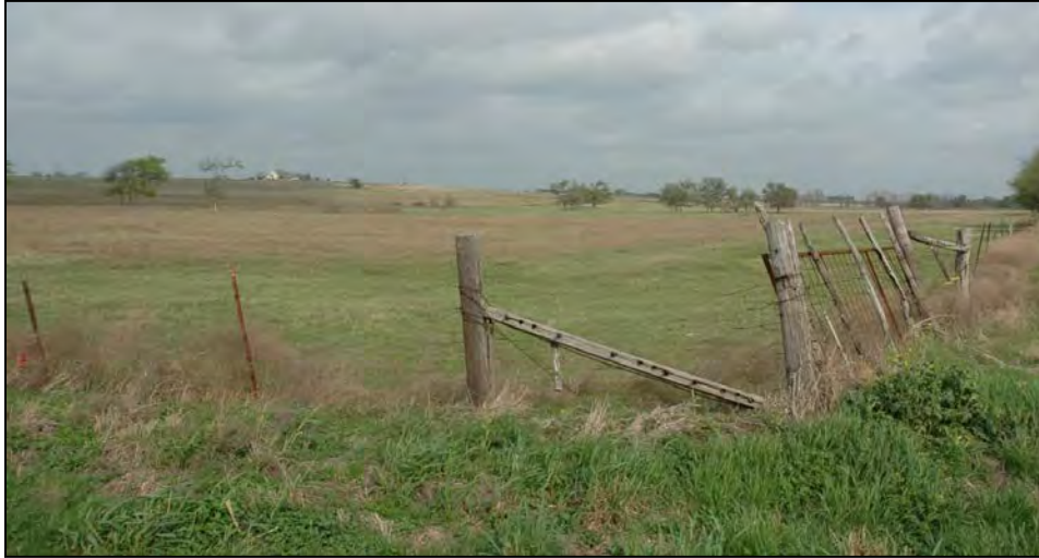
Figure 5-68. Barbed wire fencing between cedar and metal posts.
