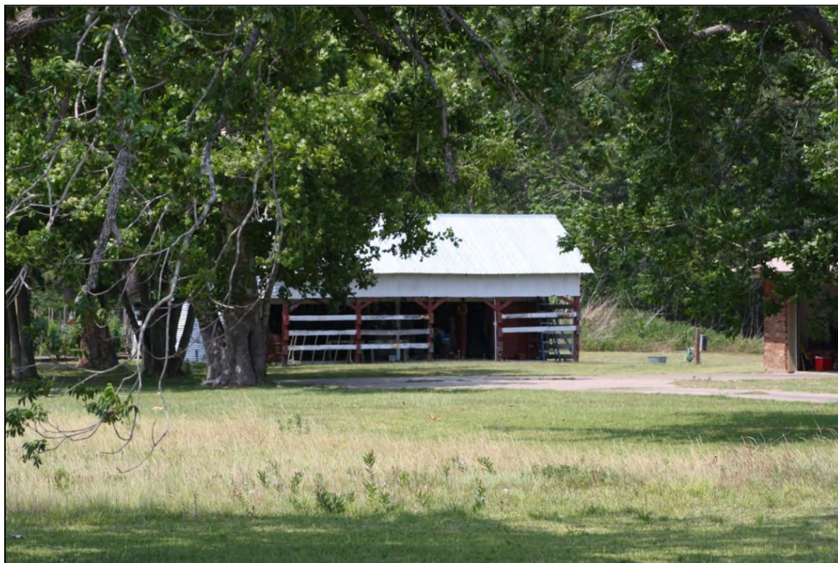
Figure 5-45. Ca. 1930 hay barn with open stalls.
