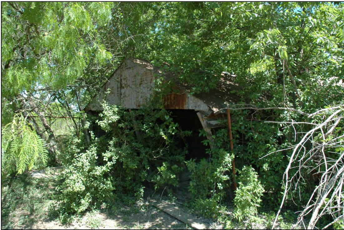
Figure 7-18. Storage structure (ID f).
