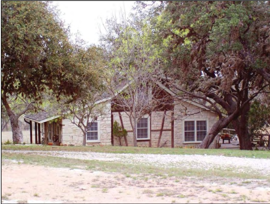
Figure 6-21. Photograph of a fachwerk house on a historic farmstead. Many German immigrants who settled in Central Texas during the mid-nineteenth century used this type of construction to build their residences. Fachwerk, which features a half-timbering framing system with brick, stone, or other materials as infill, was a popular vernacular building form of these early pioneers and reflected the cultural traditions of these German-speaking settlers.
