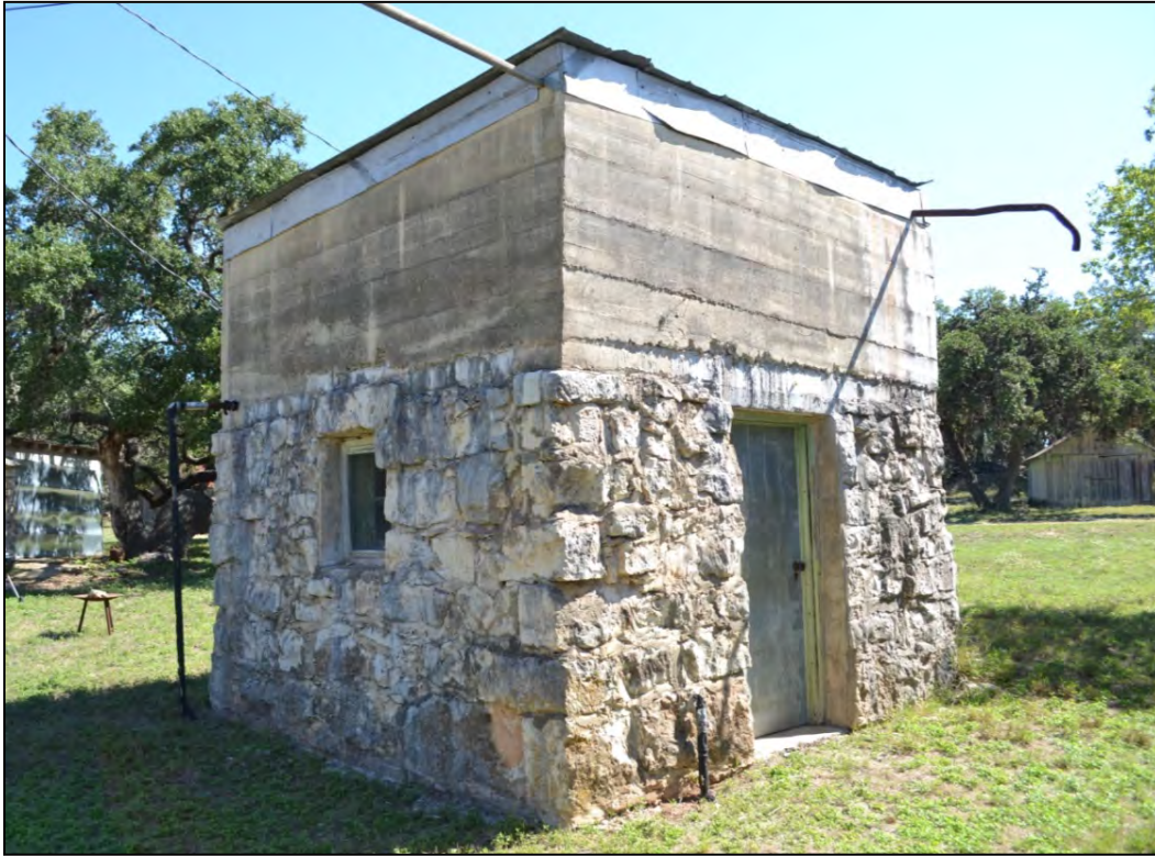
Figure 5-20. Ca. 1900 pump house. Exhibits thick stone walls with a small square window and entrance. Since its initial construction, concrete placed on top of the stone walls has raised the height of the pump house.
