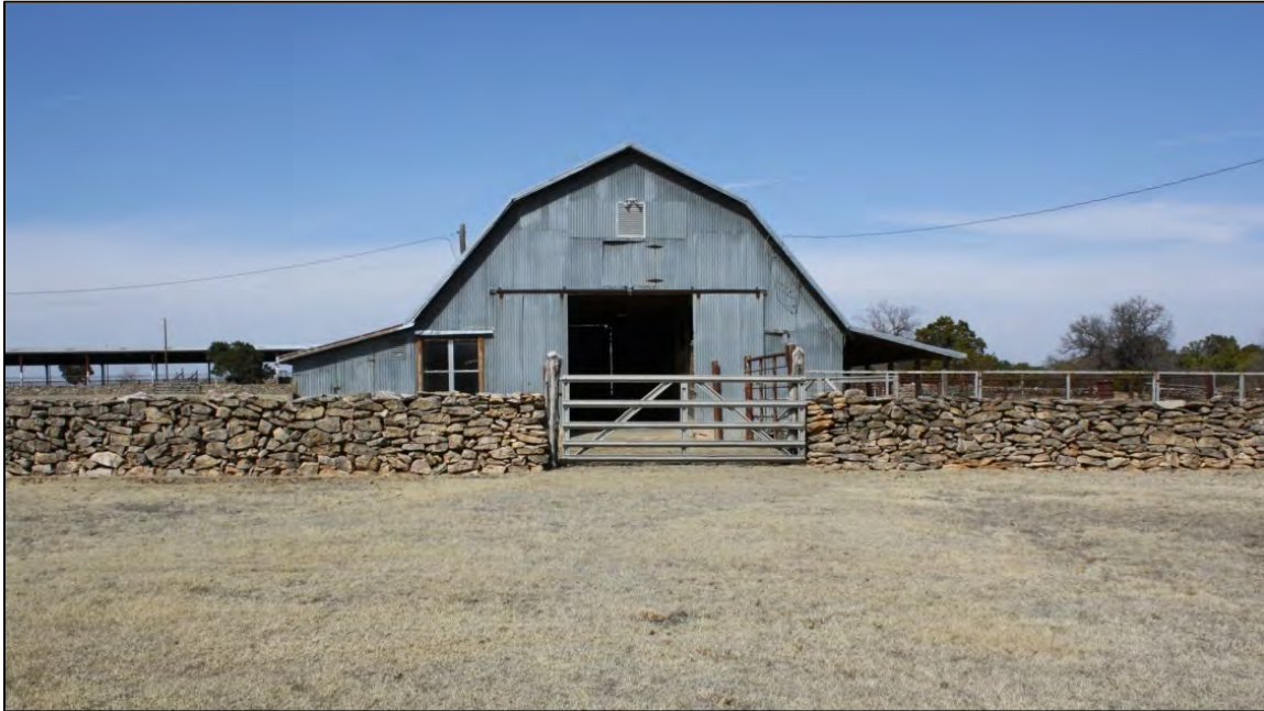
Figure 5-41. Gambrel roof transverse barn with attached livestock pens and a side room on a ranching property.
