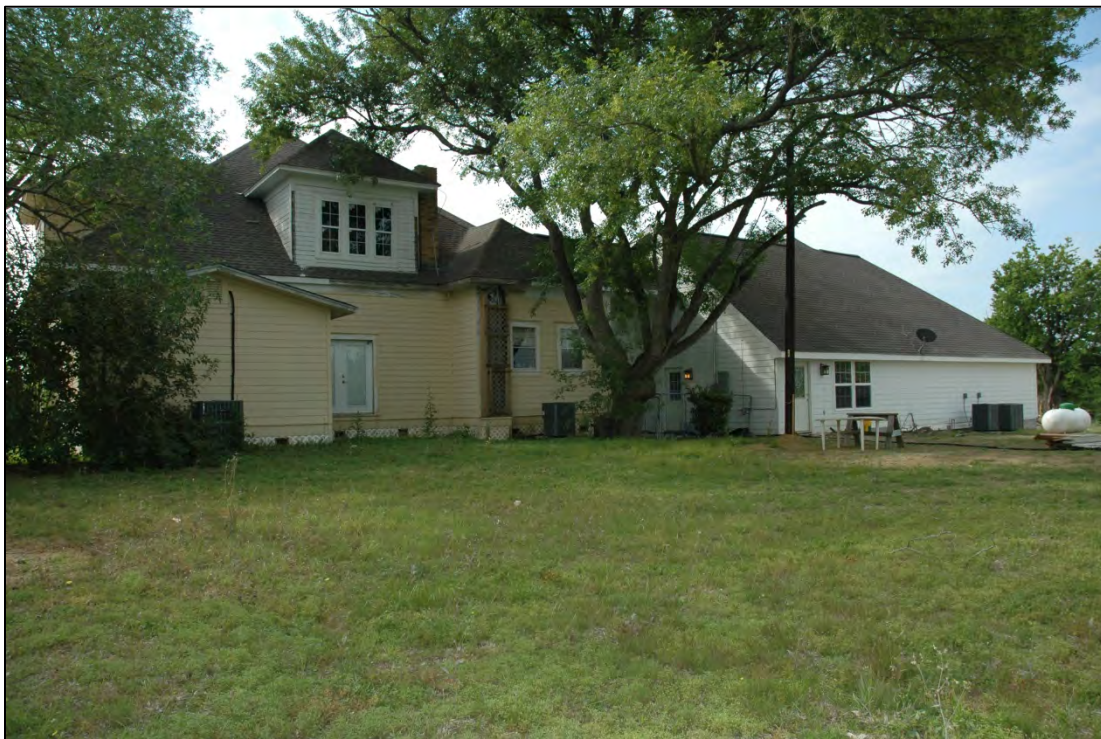
Figure 7-25. Photo of northwest façade of main house (ID a), showing restroom addition constructed ca. 1960 at the middle of the original façade and rear addition constructed in 2008 at the rear of the original façade.
