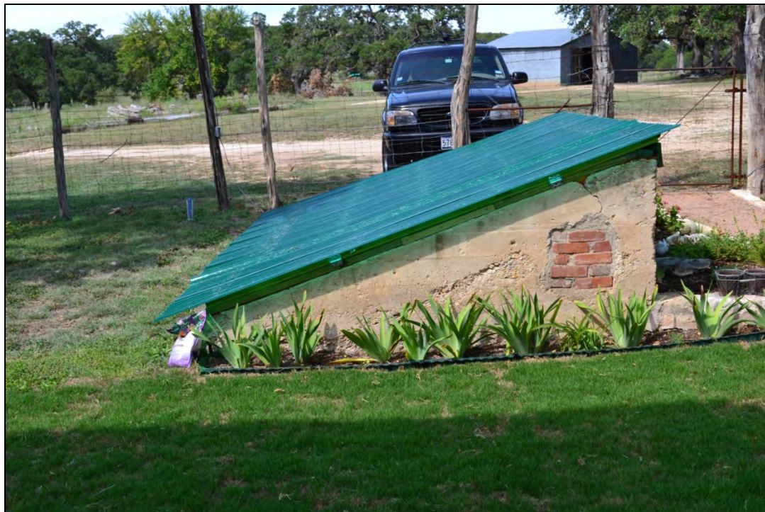
Figure 5-34. Detached root cellar.
