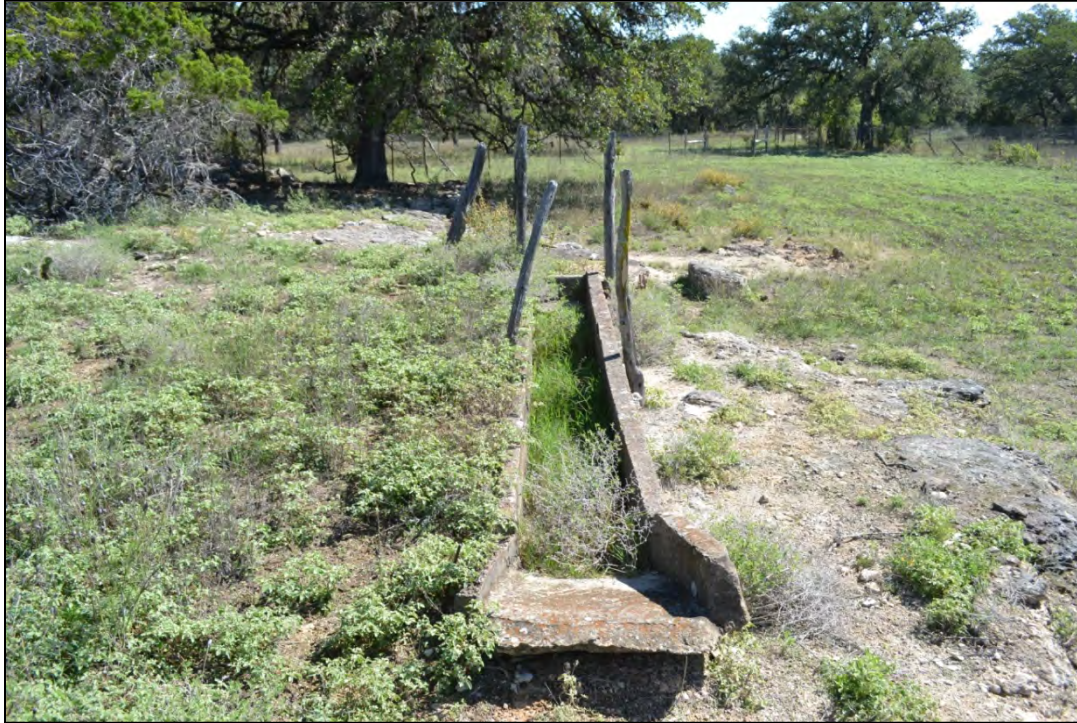
Figure 5-54. Concrete dipping vat.
