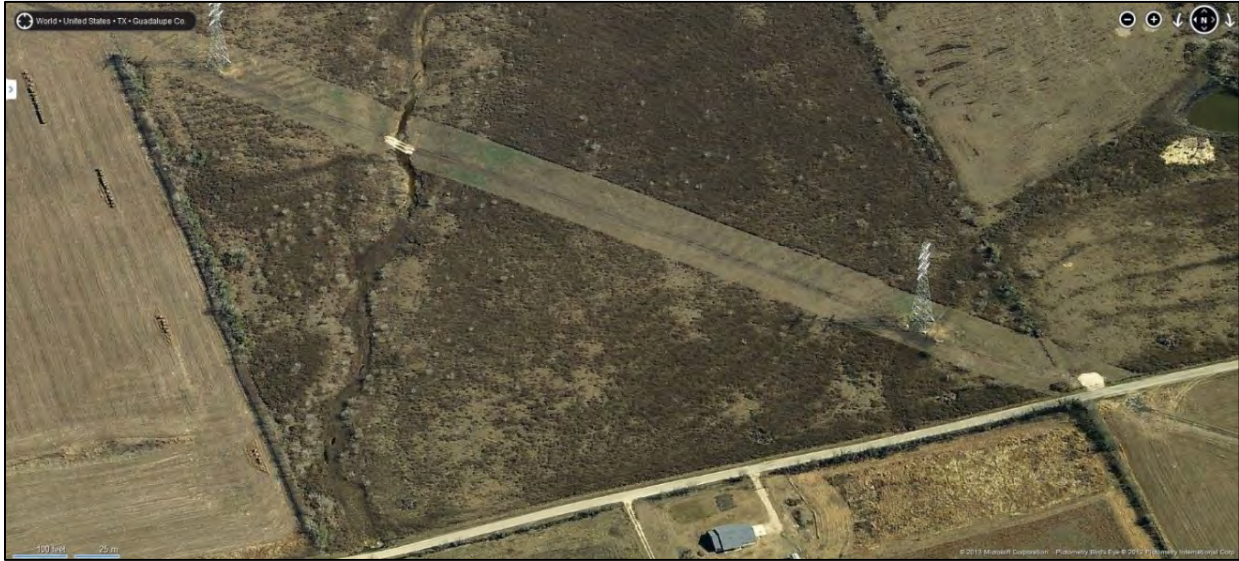
Figure 6-19. Aerial photograph showing power lines running through an agricultural field, disrupting historic patterns of spatial organization and detracting from the property's integrity of setting, feeling, and association. (Source: Google Earth.)
