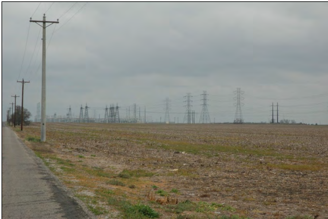
Figure 3-20. Rural Landscape in Guadalupe County. This image shows the visual effect of power transmission lines to an agricultural property near Geronimo, off SH 123. The land continues to be used for crop cultivation, but the introduction of high-power transmission lines disrupts the historic character of the landscape and diminishes the area's ability to convey a sense of the past.
