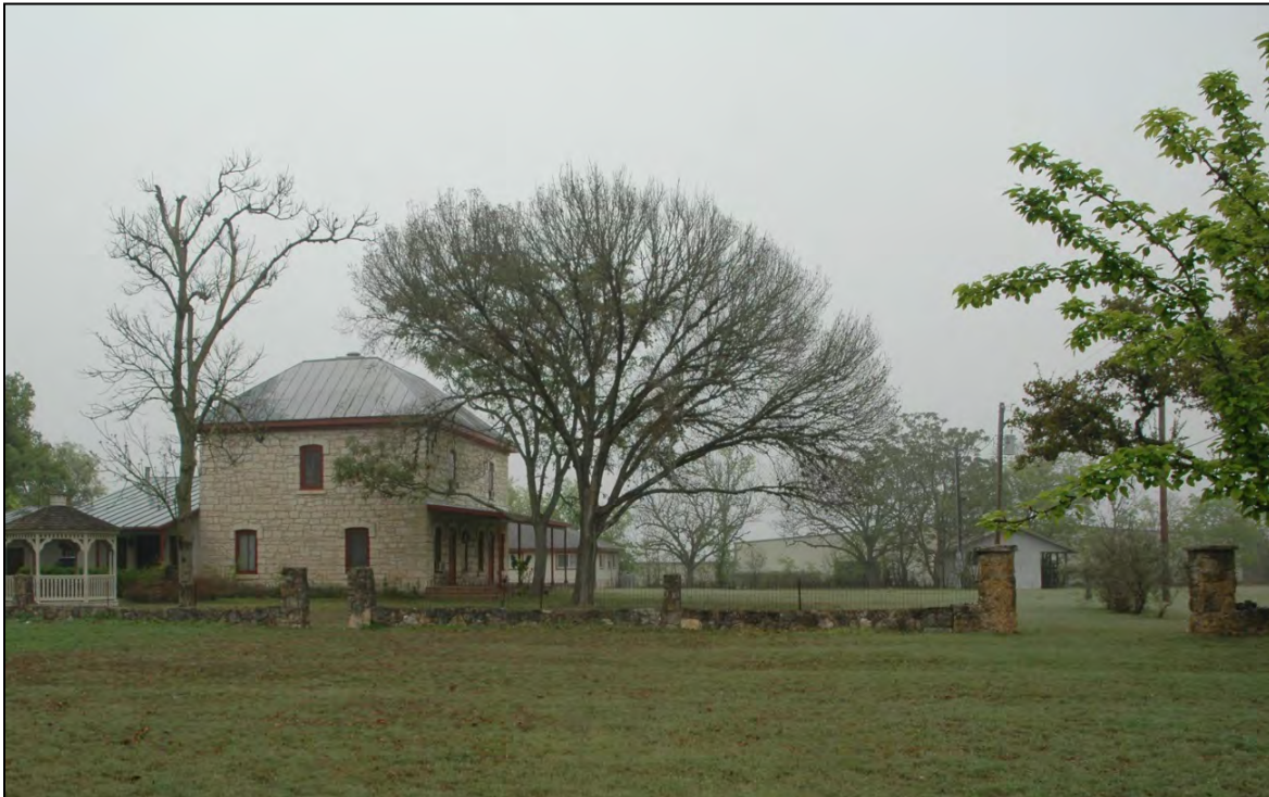
Figure 5-29. Stone fence with stone piers separating the domestic work zone from the public road (not shown).
