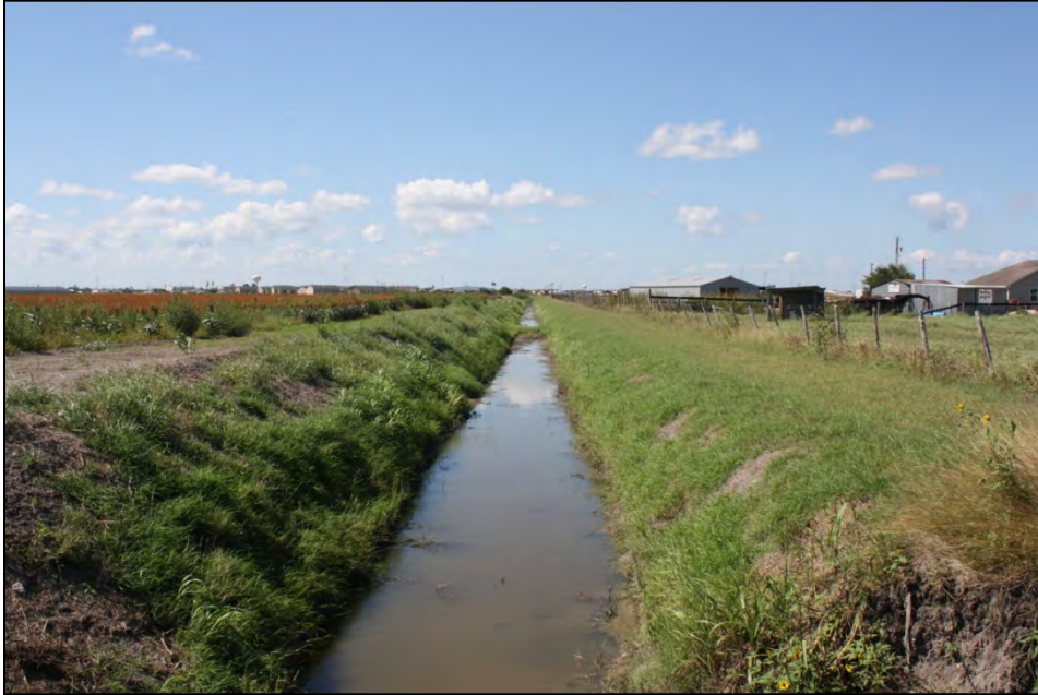
Figure 5-65. Drainage ditch adjacent to cultivated fields; note how much lower the elevation of the drainage ditch is compared to the fields.
