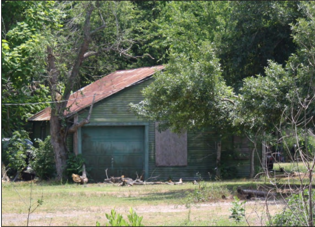
Figure 5-9. Ca. 1940 detached garage with metal siding and roofing.
