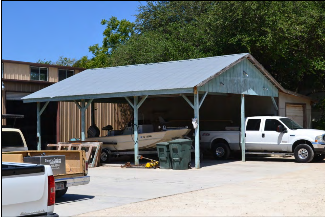
Figure 5-10. Timber-frame carport with gabled roof. The carport is attached to a single-stall garage.
