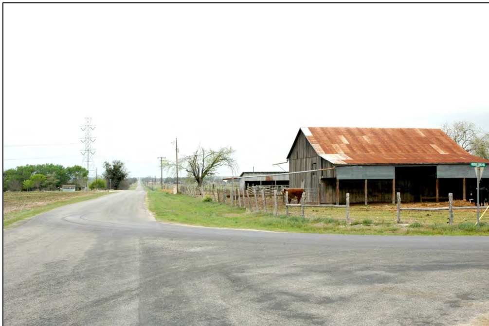
Figure 3-25. View of Spatial Relationships between the Agricultural Work Zone and the Existing Road. This is an important aspect to document in order to assess potential effects to the property.
