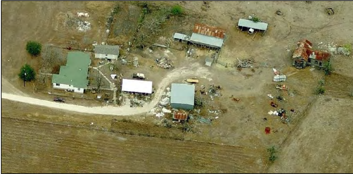
Figure 6-32. Aerial view of a farmstead in Guadalupe County. The introduction of modern buildings on the landscape, combined with the deterioration of historic-age buildings, negatively affects the farmstead's integrity of design. (Source: Bing Maps.)
