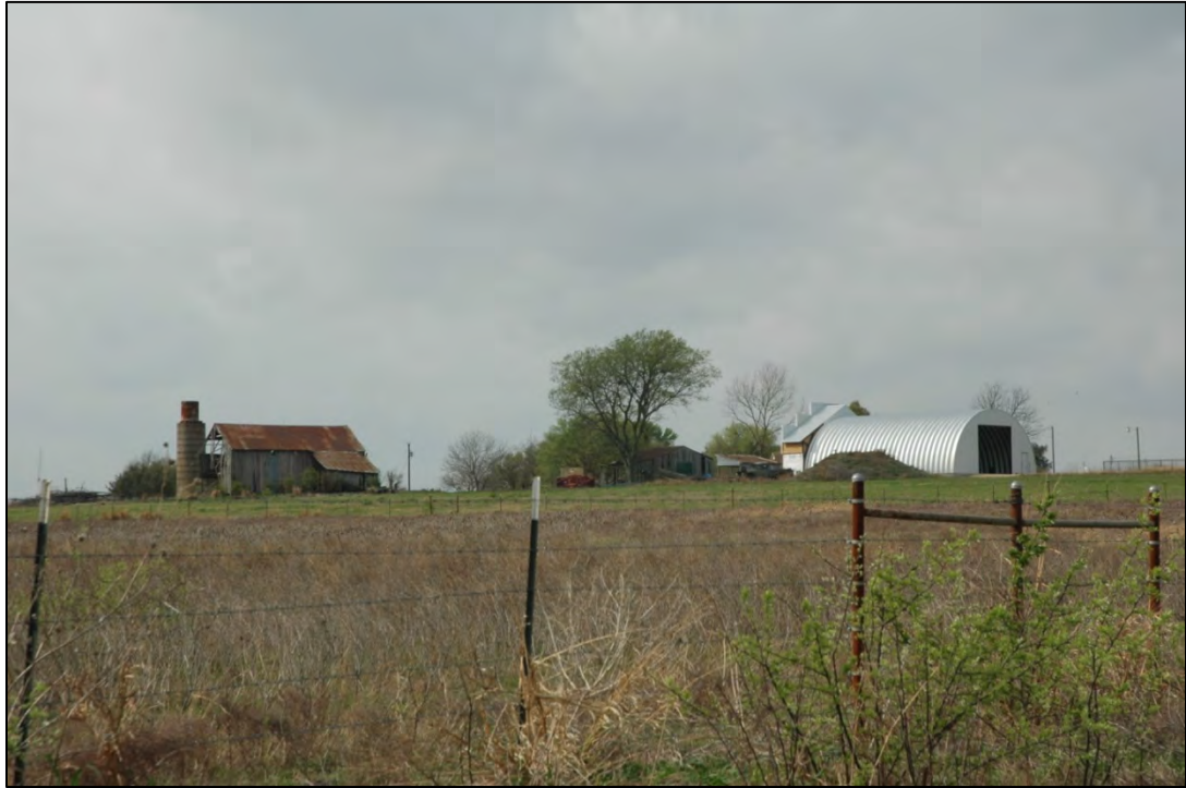
Figure 3-19. Agricultural Complex in Falls County. The metal-clad building is an intrusive element that detracts from the historic character of this agricultural property.
