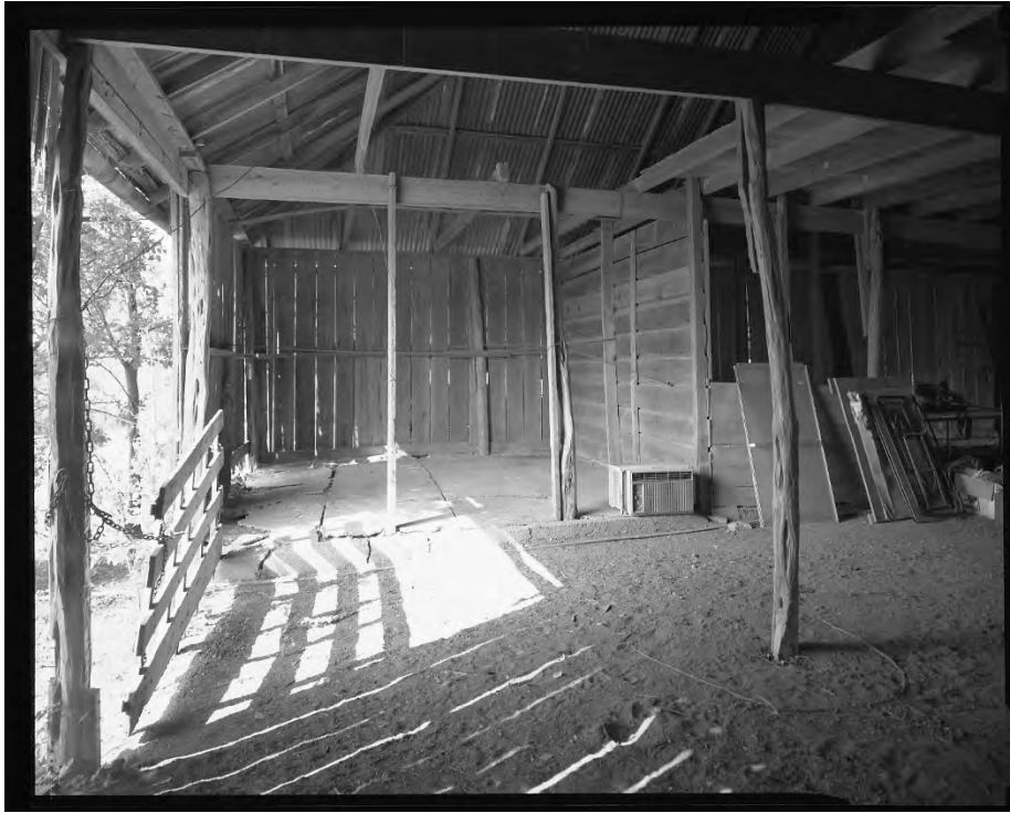
Figure 6-9. An interior view of a barn located on the E. W. Raney Farmstead in Caldwell County. This view, one of a series of photographs taken from HABS documentation prepared for the property, highlights the presence of a crib, a feature that is characteristic to the layout of a side-entry barn.
