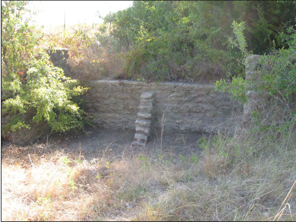
Figure 5-66. Cut stone dam. Source: TxDOT Environmental Affairs Division.
