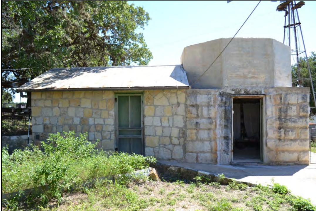
Figure 5-50. Ca. 1890 stone and concrete milk house. The room on the right with the open door most likely dates to ca. 1890, while the gabled room to the left is an addition that may date to ca. 1925. The cast concrete topping the ca. 1890 section appears to be a non-historic-age addition and may function as a cistern, given the close proximity of the windmill in the background.
