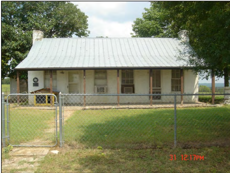
Figure 6-5. View of the front façade of the 1872 Bryson homestead in Williamson County. The house is significant architecturally because the form and plan is indicative of vernacular building traditions in Texas of the mid-to-late nineteenth century and because of the fine detail in the hand-hewn native limestone used in its construction. (Source: TxDOT.)
