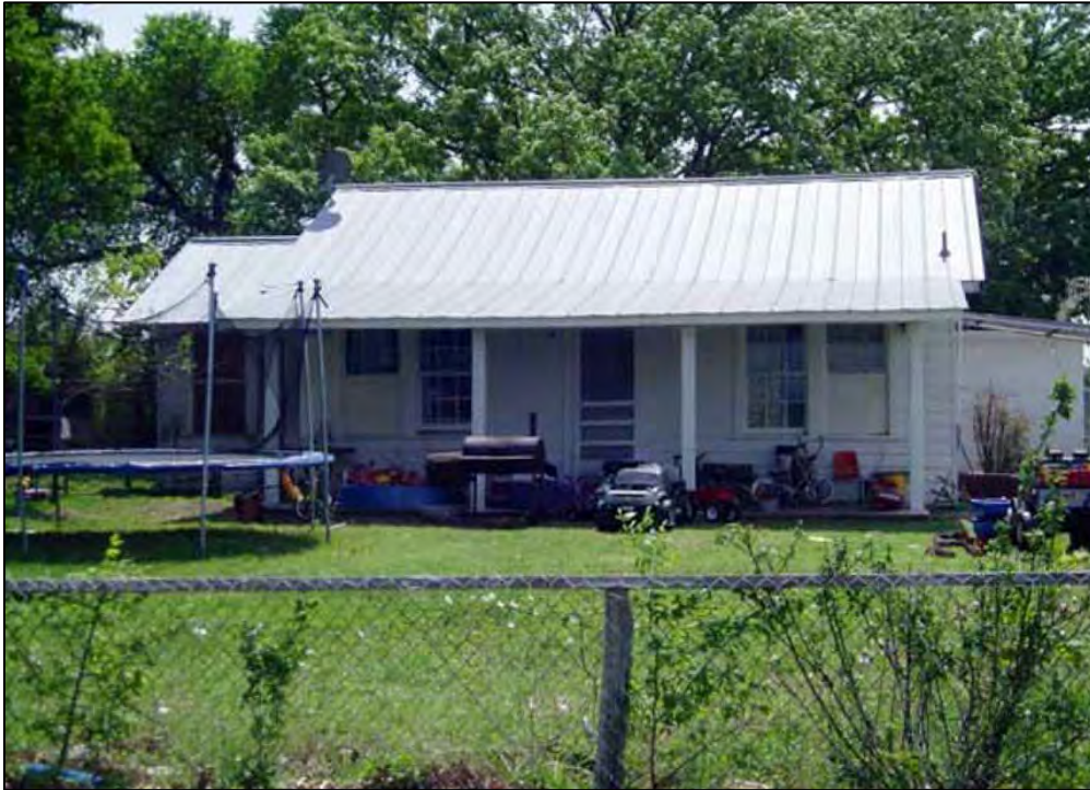
Figure 7-5. Resource ID No. 23a is the residence on an agricultural property adjacent to FM 969 east of the Austin State School. The residence was a one-story, wood frame, gable-roofed, rectangular plan structure with a brick addition that was located on the rear façade.
