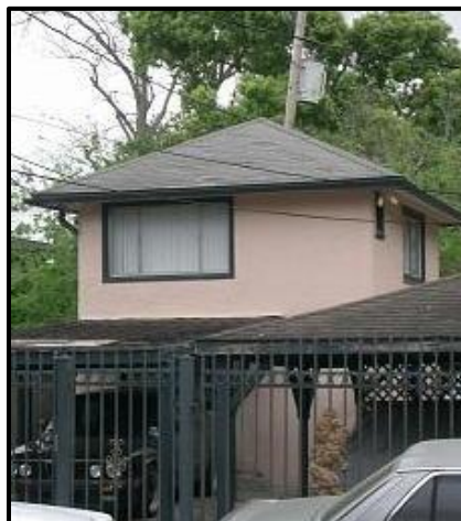
This is the garage behind 520 Branard as it looks today.
