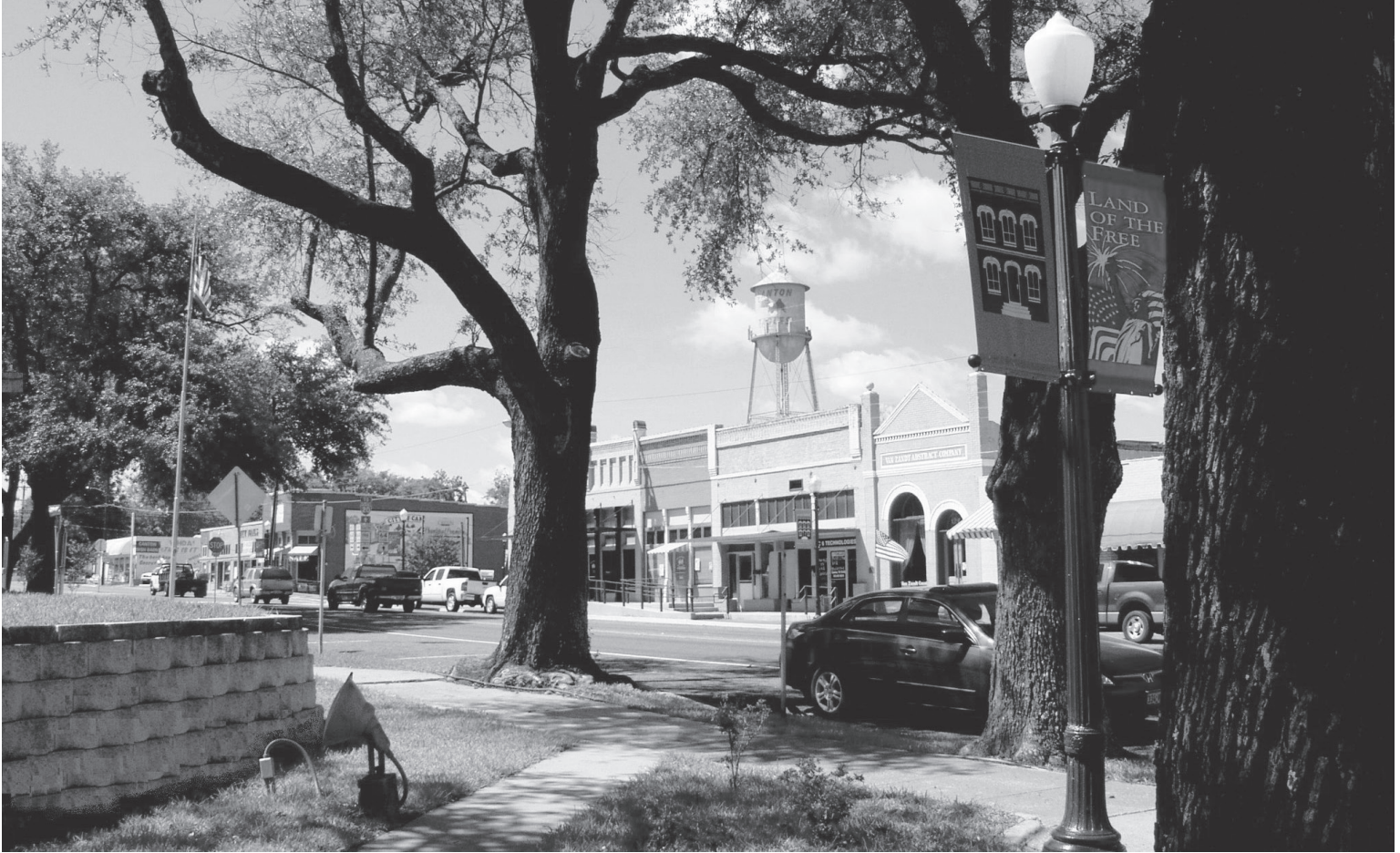
Businesses are thriving in restored historic buildings in downtown Canton. The ones in this image sit across from the town's 1937 county courthouse, built with Public Works Administration funds. Photograph courtesy of Canton Main Street. Original in color.
