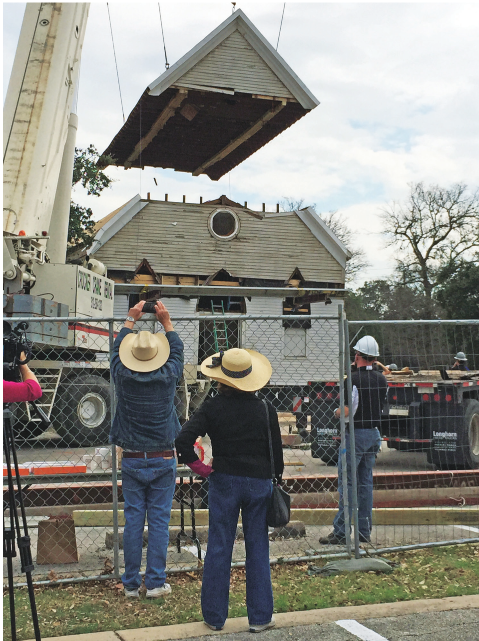
The B'nai Abraham synagogue, originally located in Brenham, was cut in three pieces and moved to Austin in 2015. Photograph courtesy of Shalom Austin and Wendy R. Corn.
