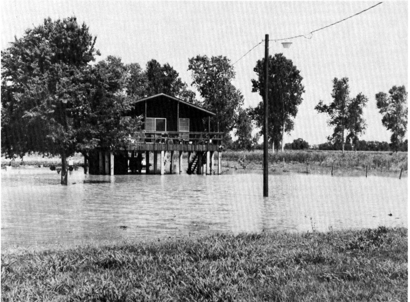
Figure 9.—Flooding in an area of Oklared-Norwood complex, frequently flooded.
