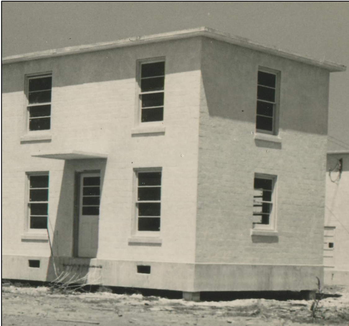
Figure 24: Detail of historic construction photo of D. N. Leathers I, Building Type E (09/09/1940) shows original windows and doors as well as the original cantilevered concrete roof above the exterior door and foundation vent placement centered under windows
