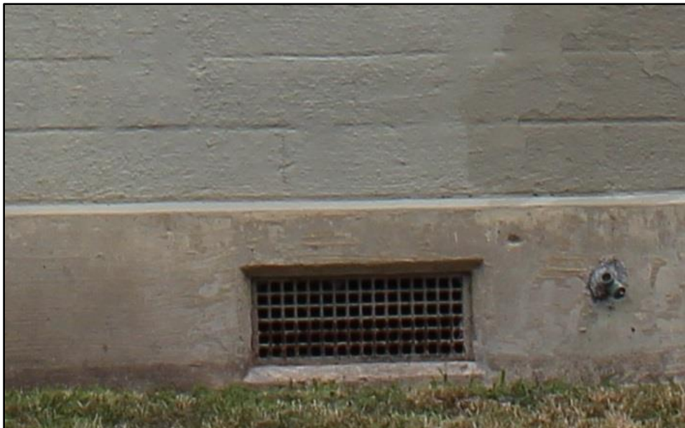
Figure 52: East facade of Building 16 (Building Type A), showing an original foundation vent
