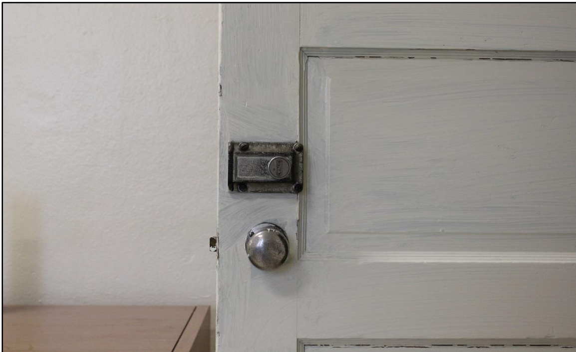
Figure 63: Example of interior view of Yale-brand rim lock thought to be typical original lock
