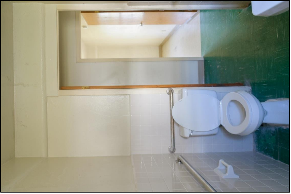
Figure B – 27: Bathroom modified to be handicap accessible c. 1997; View facing south toward bedroom showing widened doorways
