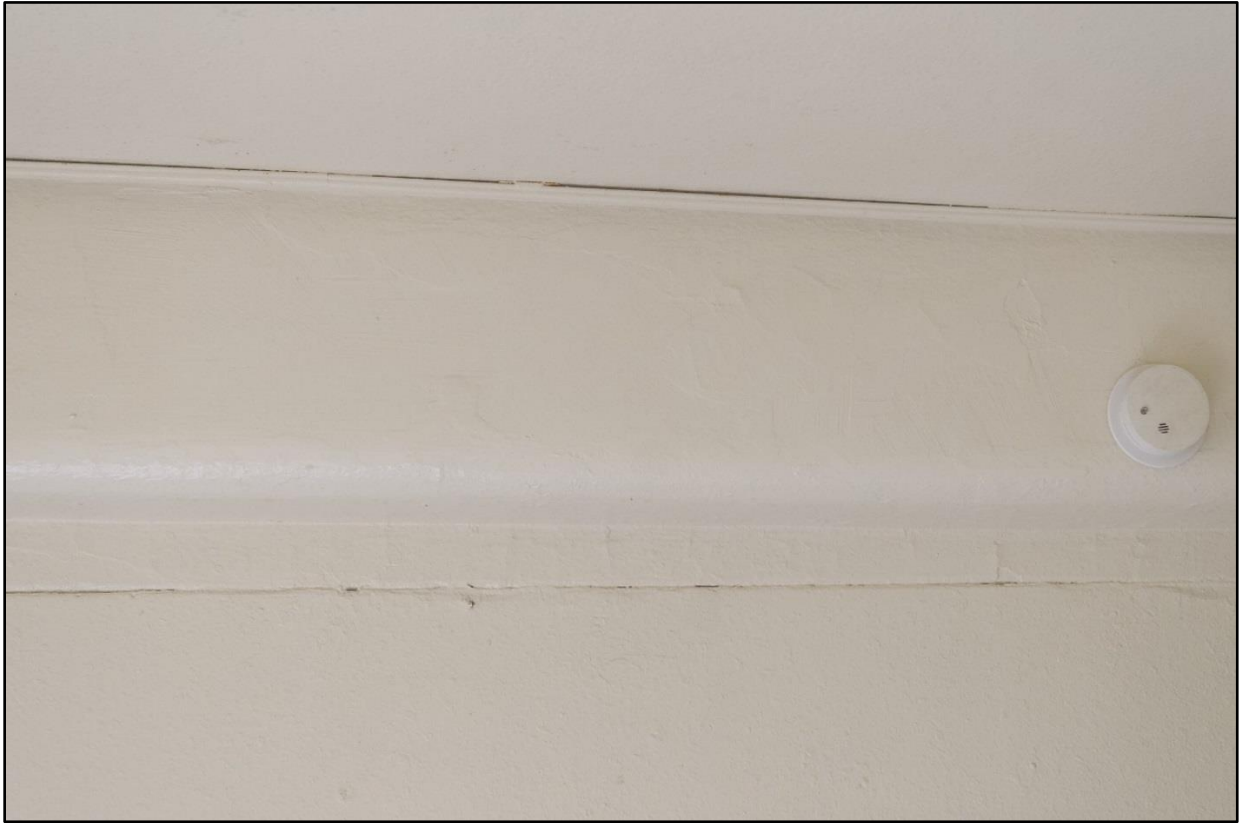
Figure 58: Interior room detail looking up at an exposed structural concrete beam
