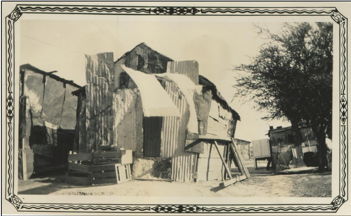
Figure 5: Substandard housing near the intersection of Sam Rankin and Antelope Streets c. 1938
