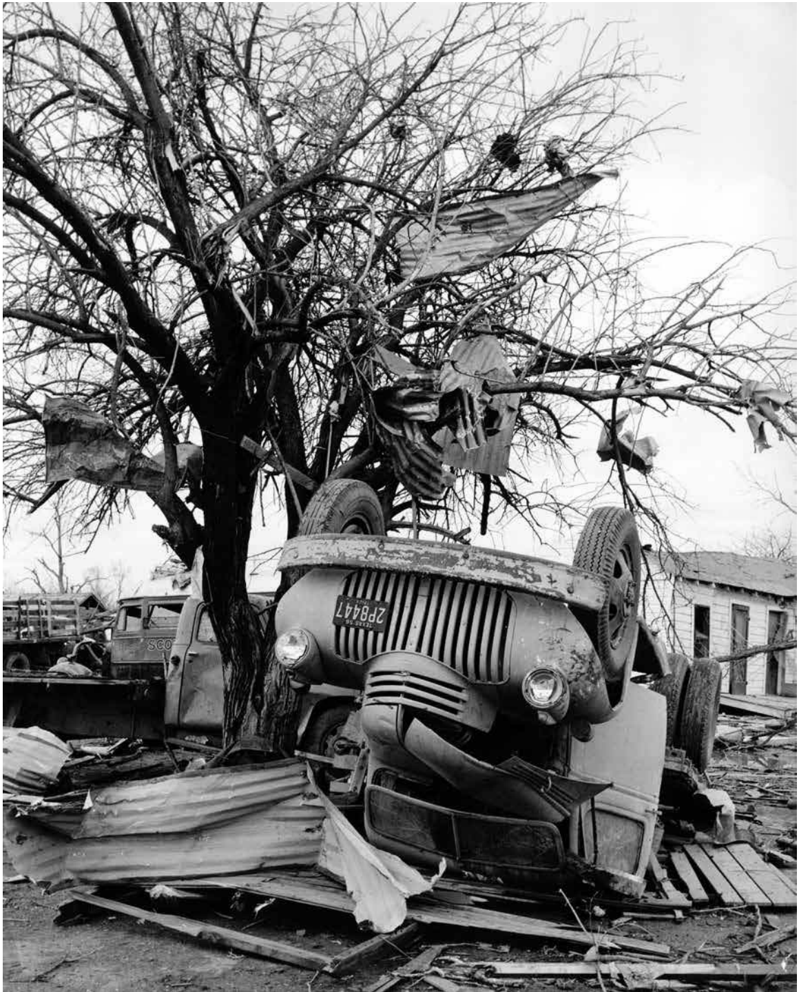
Wrecked and overturned cars, sheet metal and other debris in trees, and ruined buildings were just a few of the hallmarks left by the tornado as it churned through Dallas neighborhoods.
