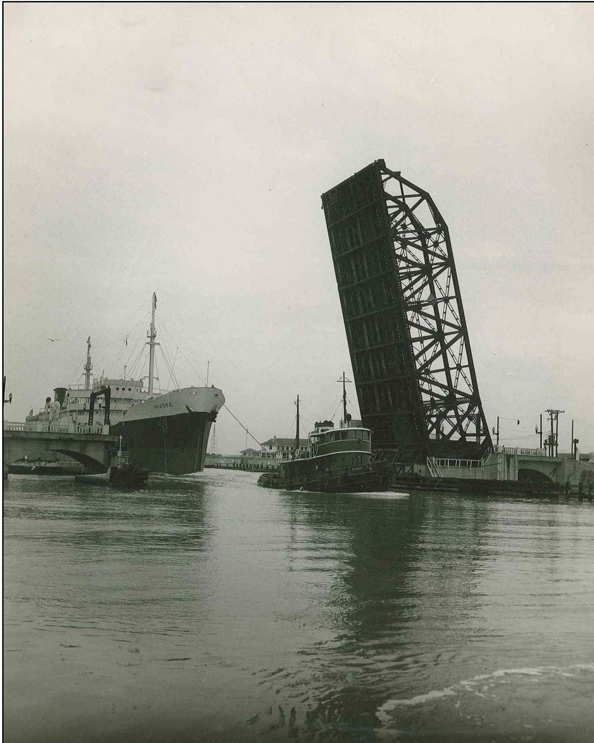
Figure 58: Bascule bridge raised to allow a tugboat to pilot a ship through the entrance to the Port Main Turning Basin
