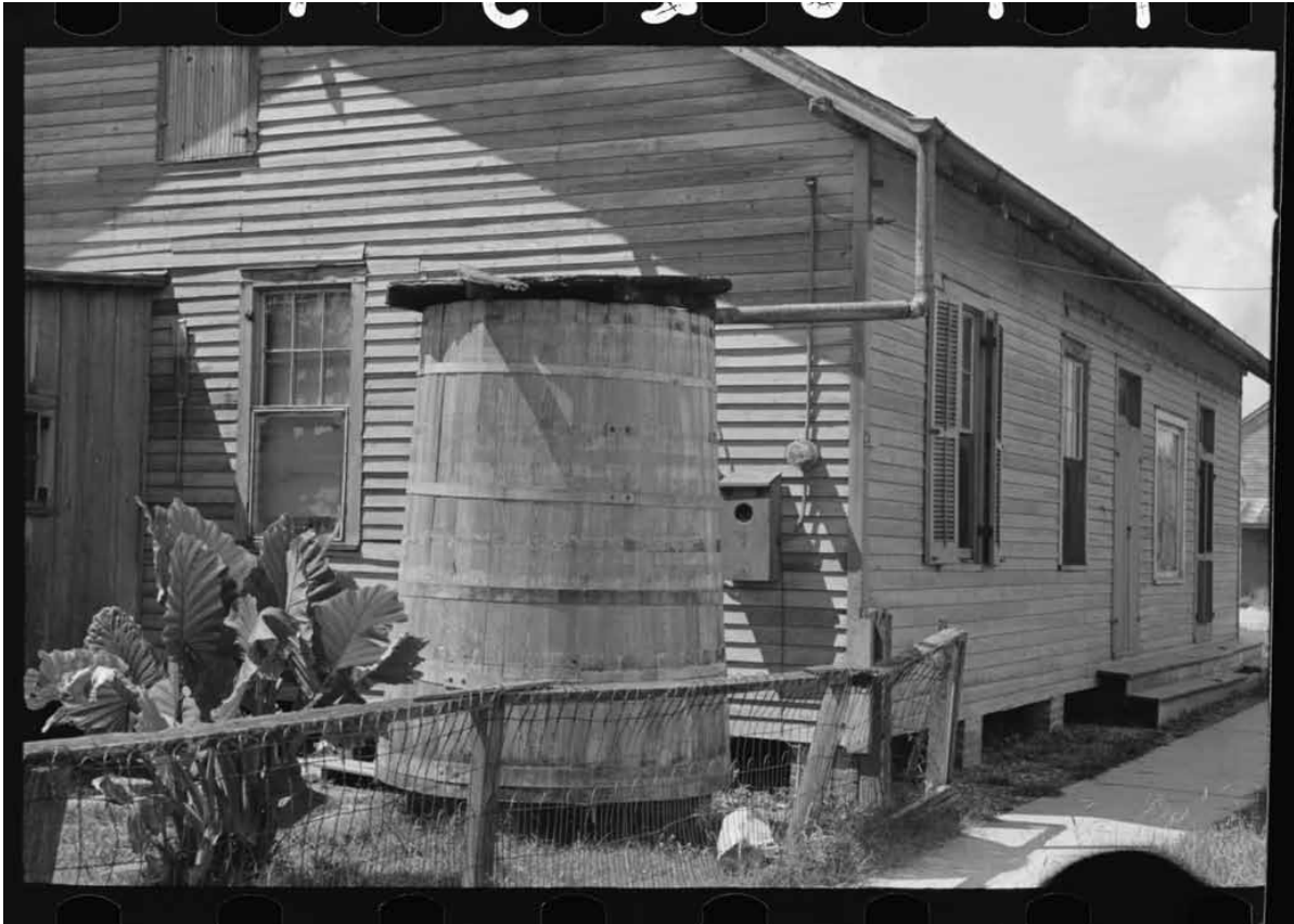
Figure 1. Photograph of a wooden barrel cistern take in 1938 by Russell (1938). From the Library of Congress's Prints and Photographic Division, this image is titled: "Outdoor cistern of house near River Road, near Destrehan, Louisiana. These open cisterns are a great breeding place for mosquitoes and are prevalent throughout southern Louisiana."
