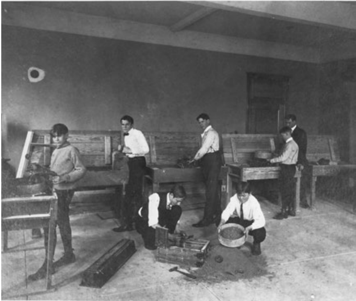
When the new Dallas High School opened in 1908, it included dedicated spaces in the basement for various vocational training programs, such as this molding class. Teacher O. A. Hanszen is standing at the far right, assisting a student. See “J. L. Long: Bringing Dallas Schools into the 20 th Century,” beginning on page 14.
