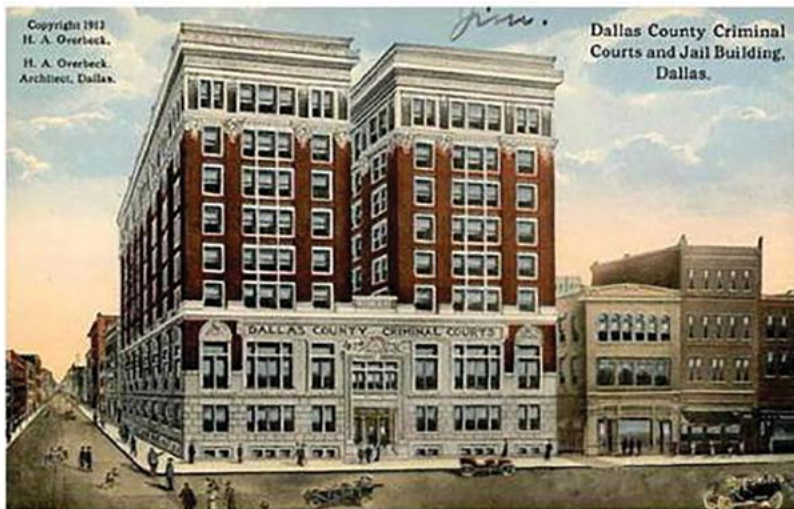
The Renaissance Revival Criminal Courts Building provided an interesting contrast to the Romanesque Old Red Courthouse across the street when it opened in 1913.
