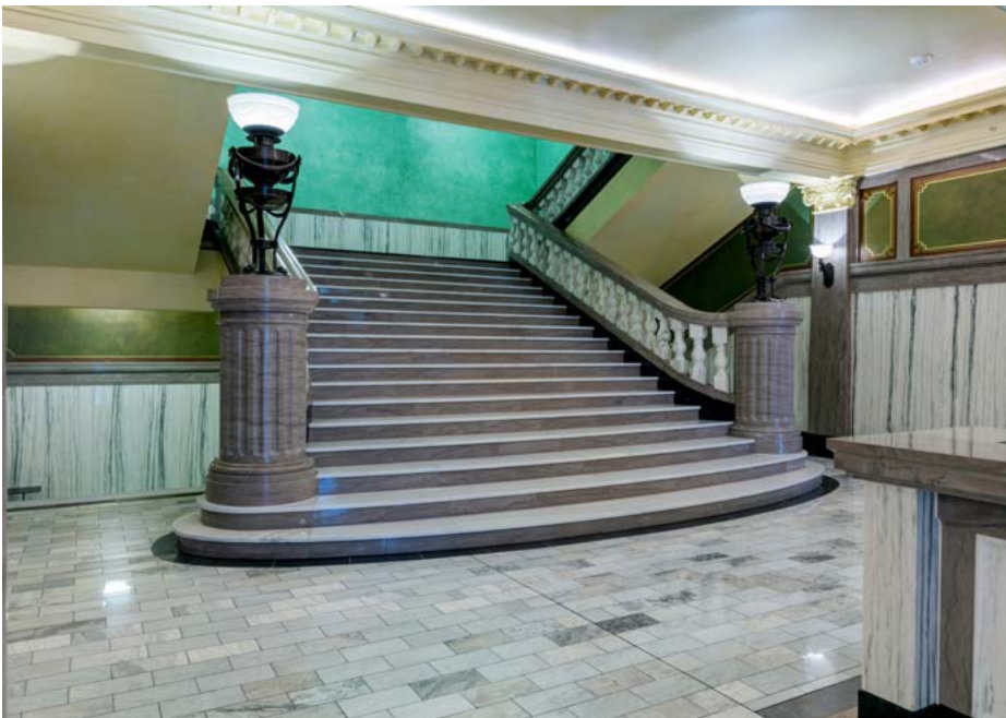
The marble stairs in the lobby have been re-created as part of the recent restoration of the Municipal Building.
