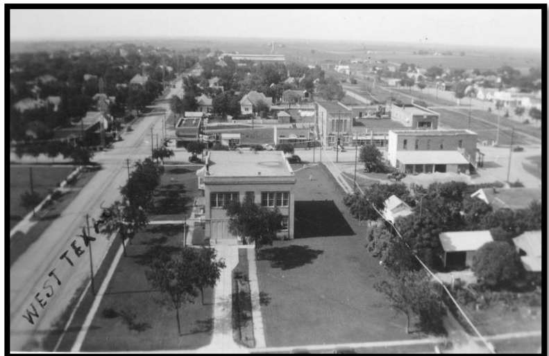
✪ Skyview of West with interurban tracks on Reagan Street.
