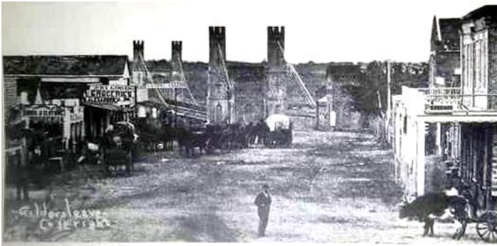
Suspension Bridge across the Brazos River, at Waco, completed 1870. This picture made in 1876.
