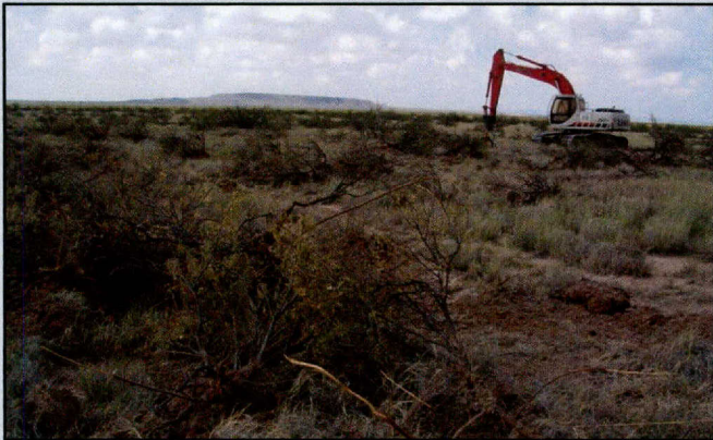
Excavator grubbing western honey mesquite. Photo provided by Bonnie Warnock, Sul Ross University.
