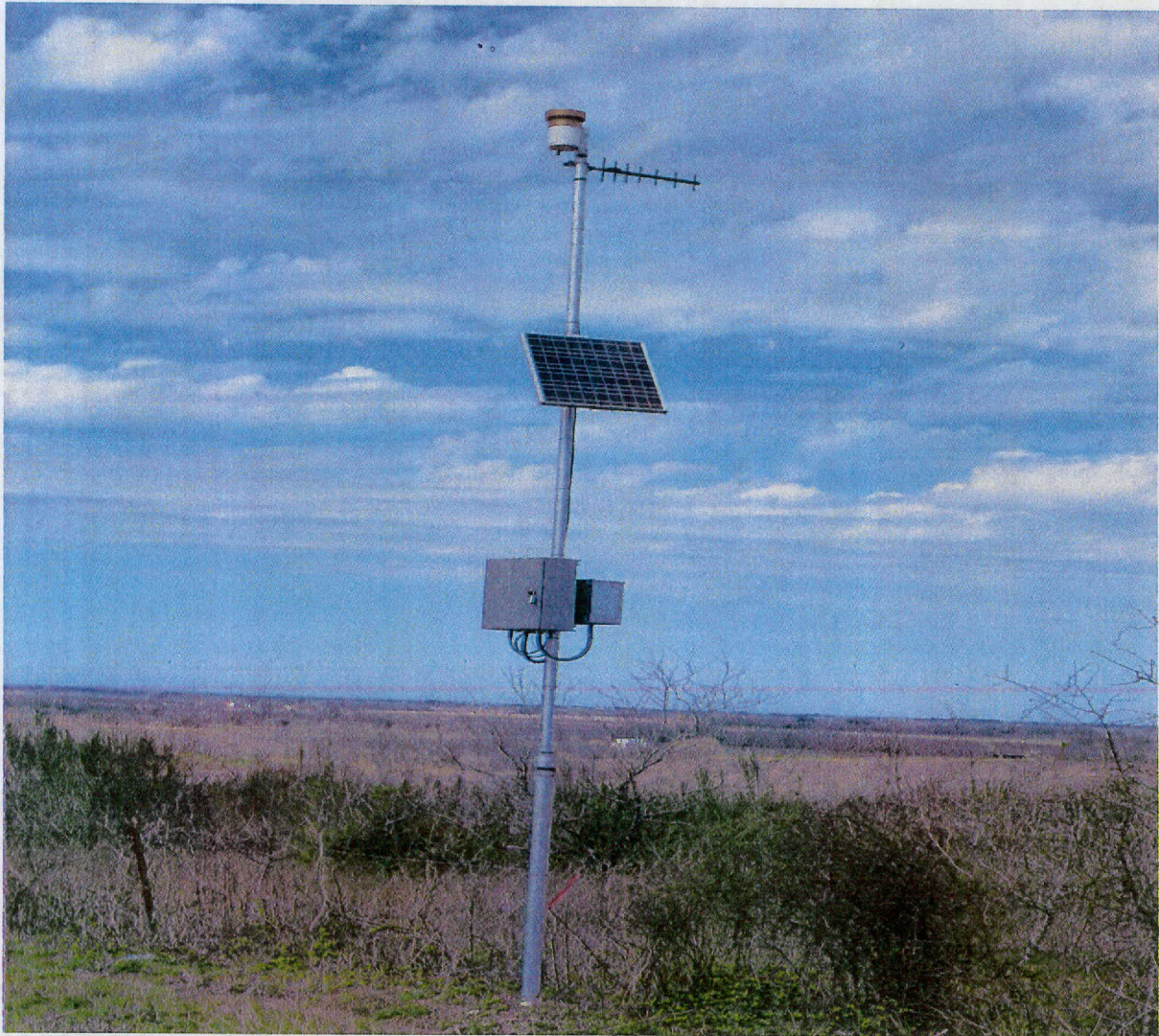
FIGURE "B-7" Rain Gauges Installed
