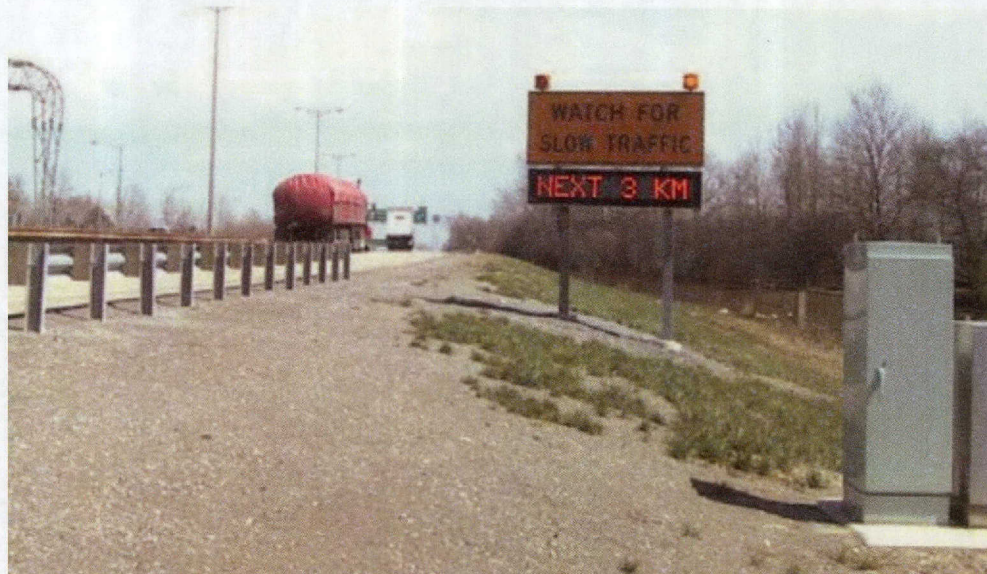
Figure 2.4 Queue warning system in Ontario, Canada (ENTERPRISE Pooled Fund Study, 2014)
