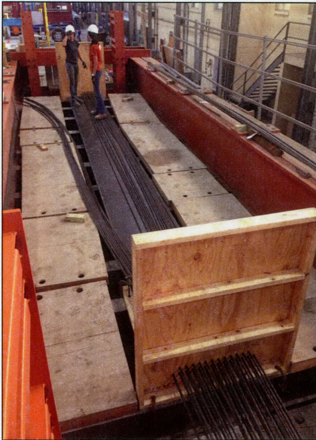
(a) Installing the strands
