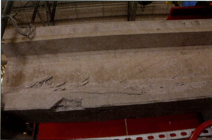
Tx46-I (East side)
