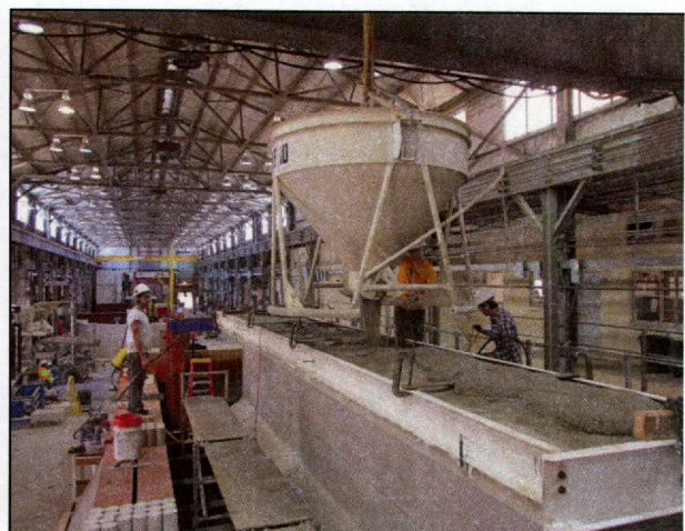
(b) Casting the deck concrete
