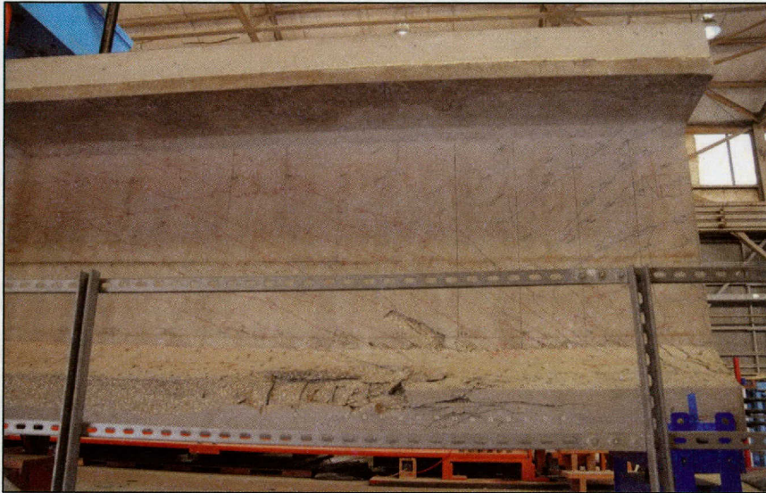
Tx70-II (East side)
