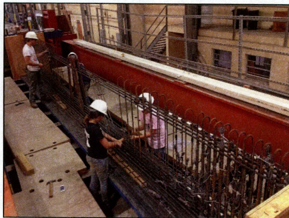
(c) Tying the mild-steel reinforcement
