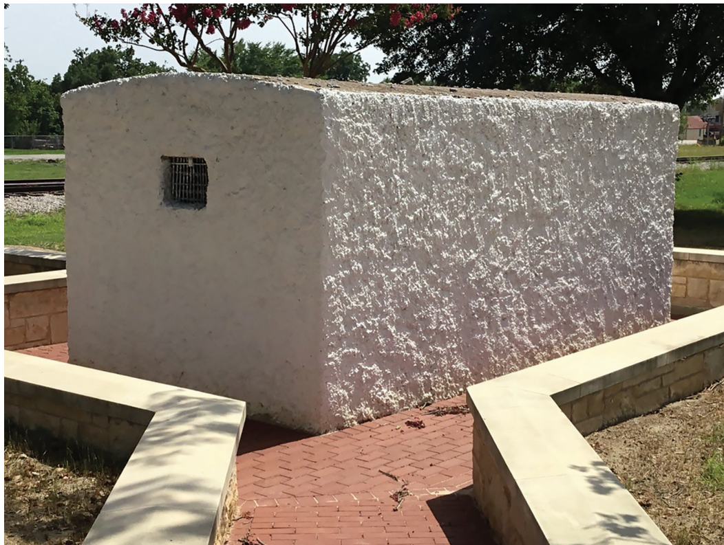
Top: The tiny jail survives to live another day. Bottom: A wheelchair ramp was added to the calaboose to allow access for everyone. Both photographs on this page courtesy of Bobby Gladu.
