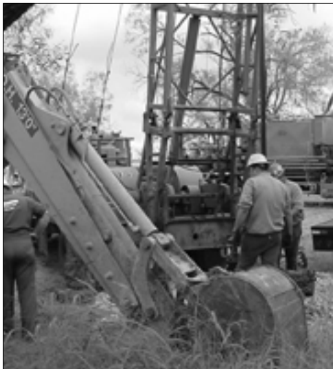
Abandoned wells are pumped out if necessary, then plugged with cement.
