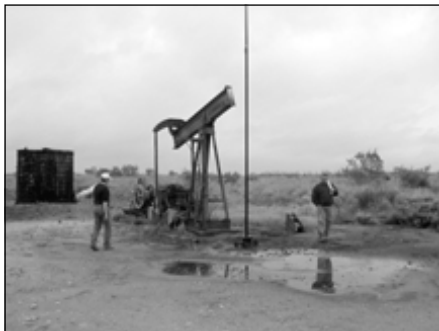
Railroad Commission personnel inspect a leaking oil well in Howard County.
