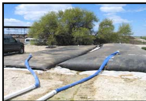
Partially filled Geotubes™
