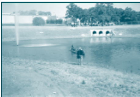
The upper pond of the three-stage wetpond during planting.
