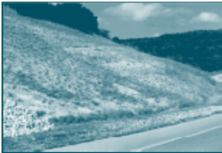
Oasis Bluff Drive site before restoration. Runoff from the site was visibly turbid.
