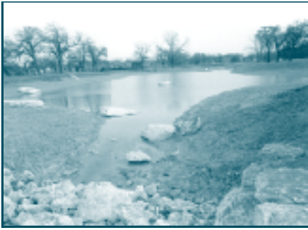
The middle pond during construction.
