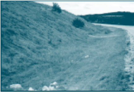
Southwest Parkway site after restoration. Erosion and soil loss was reduced by 70 percent. Total runoff quantity was also reduced.
