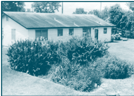
Constructed wetland at the Hadden home. Monthly samples were taken at each site for one year. Effluent quality at both sites far exceeded that produced by a typical septic tank.
