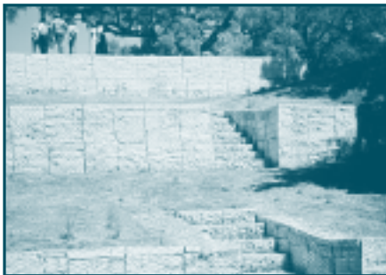
Terraced rock gabion walls form the second stage, and prevent erosion. The terraces were designed to recreate as much of the original bank structure as possible.
