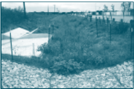
Reach Number 2 outflow and vegetation in September 1997.
