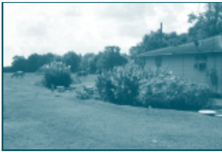
Demonstration wetland constructed at the Deadrick household. Primary treatment at each site was provided by an existing septic tank. A two-cell wetland received and treated effluent from the tank.
