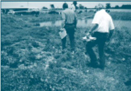
Leaking dairy lagoons in the Running Creek watershed were a waste management problem addressed by the project partners and local dairy operators.
