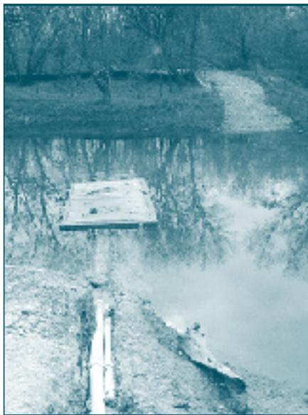
Antioch cave BMP several days after a heavy rain resulted in an 8 to 9 feet deep flood. The first flush has passed and the water is about 6 feet deep and very clear. The valve is open and a small whirlpool can be seen near the far end. The large PVC pipe is a line vent and the smaller one contains monitoring and sampling lines. The stabilized construction entrance and protective fencing can be seen on the opposite bank.
