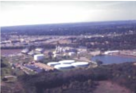
Spencer Water Treatment Plant
