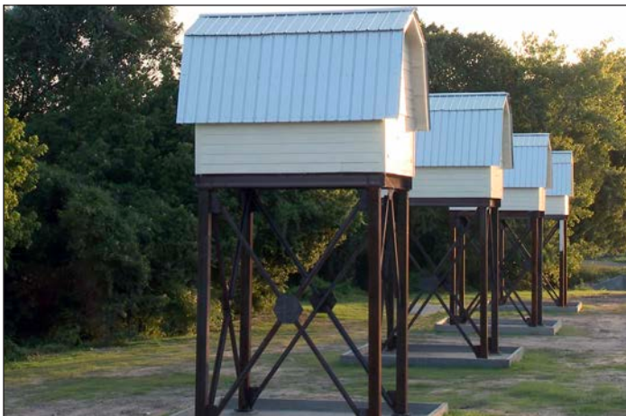
The Facilities Division oversaw construction of bat houses near the Huntsville Unit as part of an effort to relocate a large colony of bats currently living in an old, abandoned warehouse slated for demolition.
