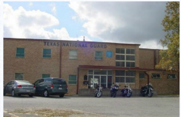
NEW BRAUNFELS ARMORY: New Braunfels (FY - 2021 Project)
