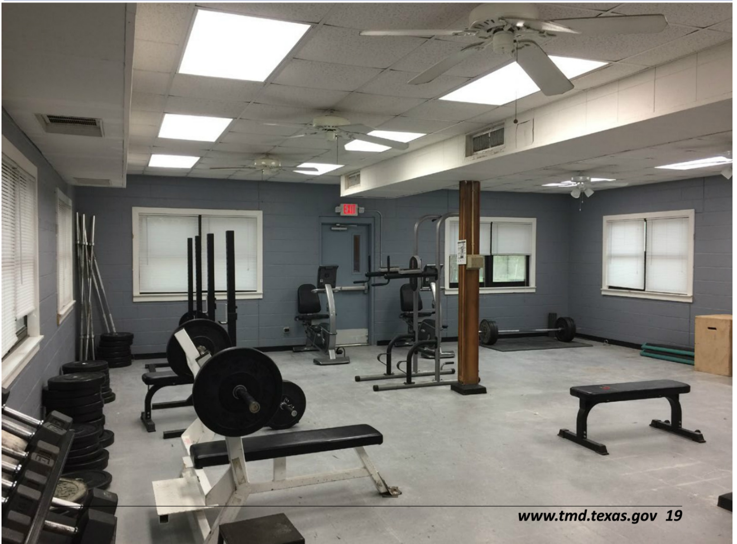
(BELOW) Final product of the Bee Caves Armory gym with painted walls, rehabilitated ceilings, floors and more.
