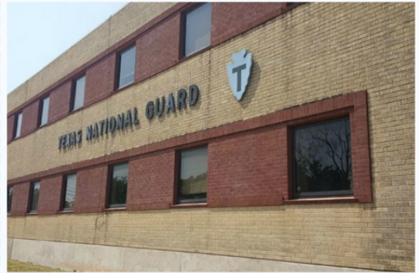
WACO ARMORY: Waco (FY - 2021 Project)
