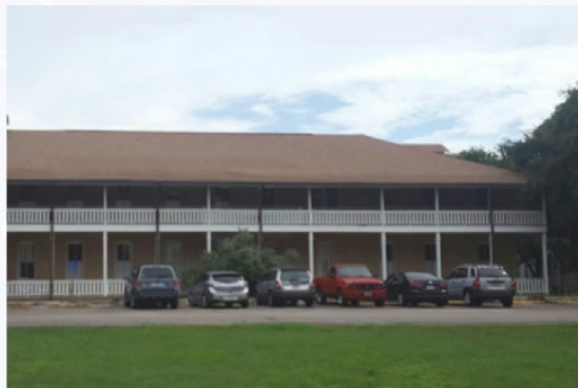
CAMP MABRY (Building 1) Austin (FY - 2018 Project)
