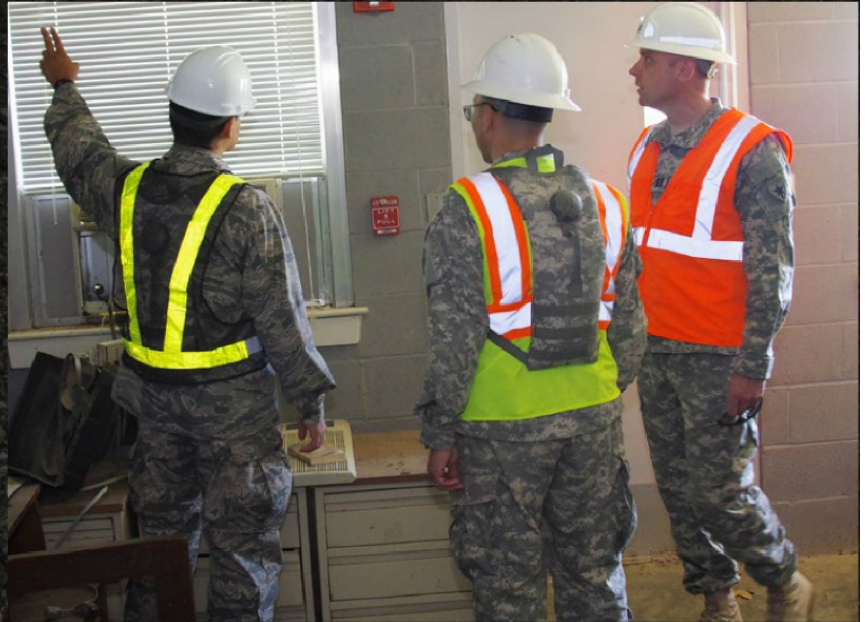
Inspectors from the Texas State Guard Engineer Group check the electrical conduits and structural defects in a building at Camp Swift, Bastrop, Texas, April 2018. (Texas State Guard Photo By: Sgt. 1st Class Malcolm Cowdin)
