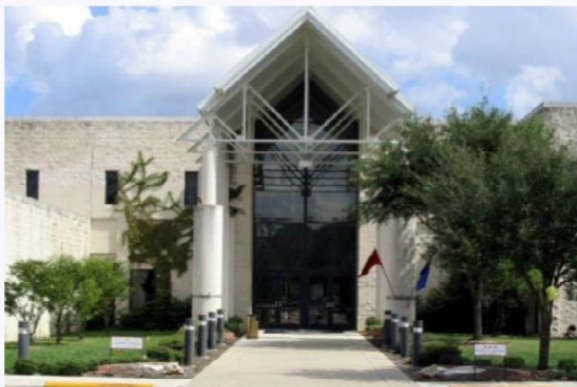
CAMP MABRY (Building 8) Austin (FY - 2020 Project)
