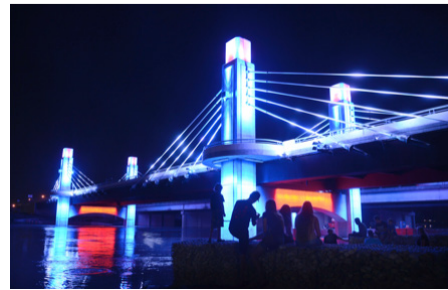
I-35 Frontage Road Bridge at Brazos River, Waco
