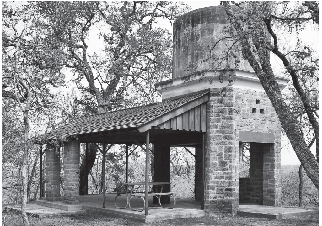
Top: More than eight decades later, this stone arch bridge remains a visible reminder of the work completed by CCC enrollees. The Lockhart project was one of more than 50 parks completed by the New Deal program. Bottom: The stone masonry surrounding the state park’s historic water tower was designed to support the concrete tank. Photographs courtesy of Larry D. Moore. Originals in color.
