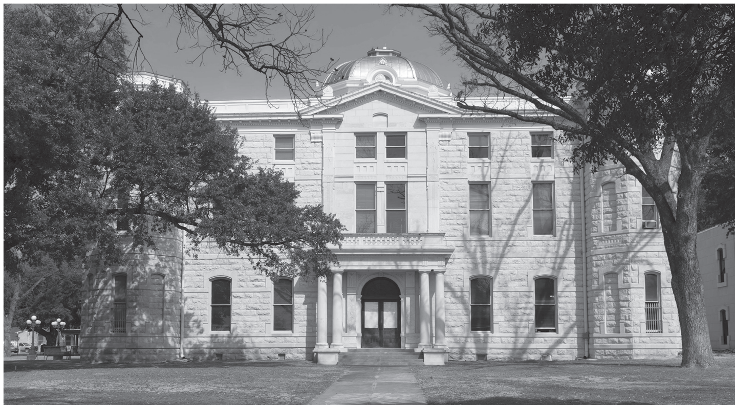
Above: The Val Verde County Courthouse was one of the first masonry commissions for Italians G. B. Cassinelli and John Taini. The limestone came from a quarry about six miles north of Del Rio. Photograph by Carol Highsmith. Courtesy of the Library of Congress, Prints and Photographs Division. Original in color.
