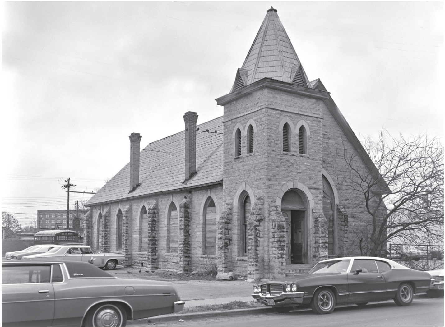
Above: The masonry on Del Rio's old Methodist Church was completed by John Taini. The stonework was painstakingly repointed during a restoration project in 2017. The historic structure now serves as a community center. Photograph courtesy of the Texas Historical Commission Historic Resources Survey Collection, University of North Texas Portal to Texas History.
