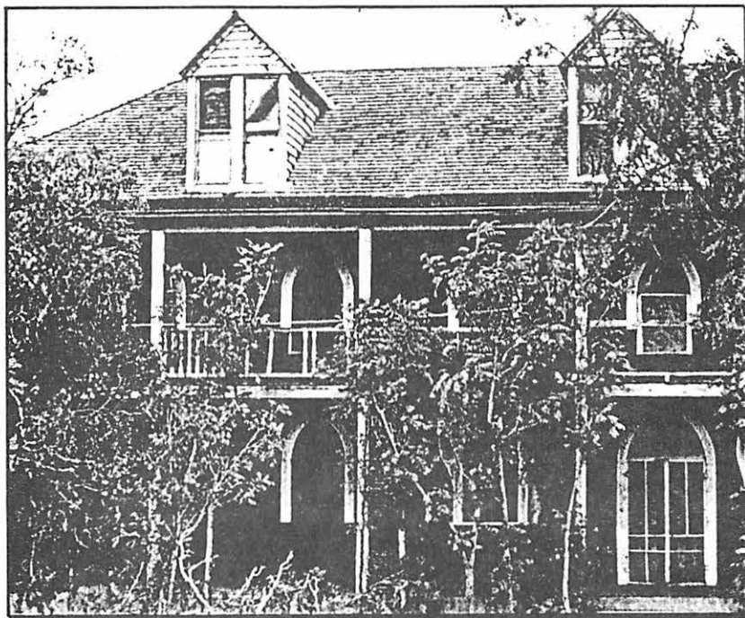
The Academy of Our Lady of Mercy in Stanton was for many years the only school between Dallas and Phoenix. The clapboard covered adobe convent was spared in a 1938 tornado that destroyed the church and dormitories.
