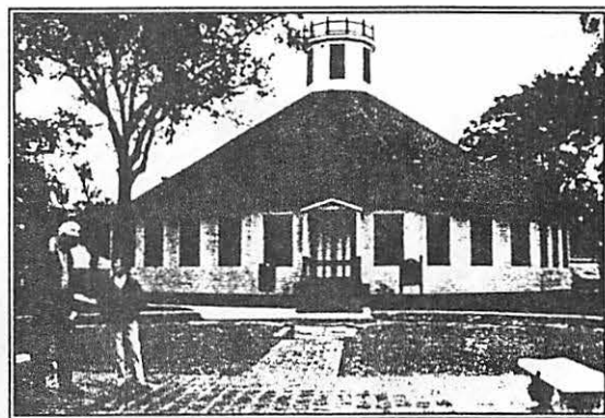
Bellville Historical Society leaders look at engraved bricks in front of the Bellville Turnverein, built in 1889. After a fire, it was rebuilt as a 12-sided pavilion with a center pole for support. It is owned by the City of Bellville.
