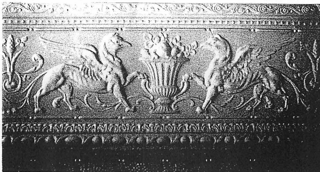
BELOW: The embossed tin ceiling of the front bedroom has a border which incorporates mythological figures such as these griffins.
