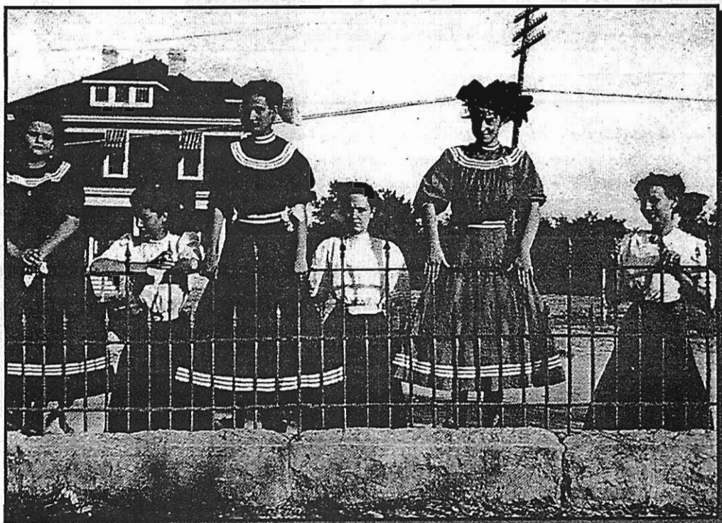
1914 Girls at Iron Fence. Notice the large cement blocks holding up the fence.
