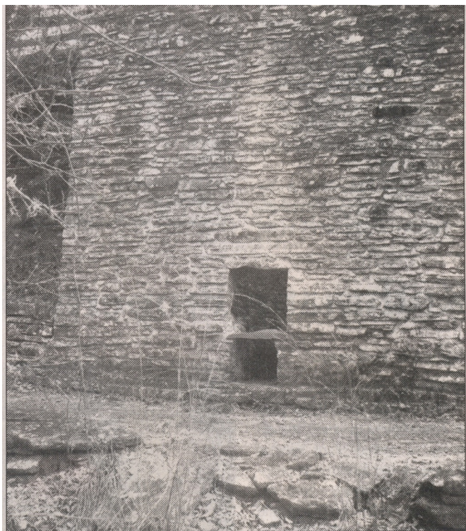
Kreische’s limestone kiln near his brewery at Monument Hill State Park. Photo courtesy of Charles Hebert
