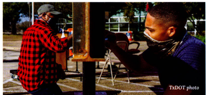
TxDOT employees at the Cedar Park Campus in Austin sign their name to the beam.
