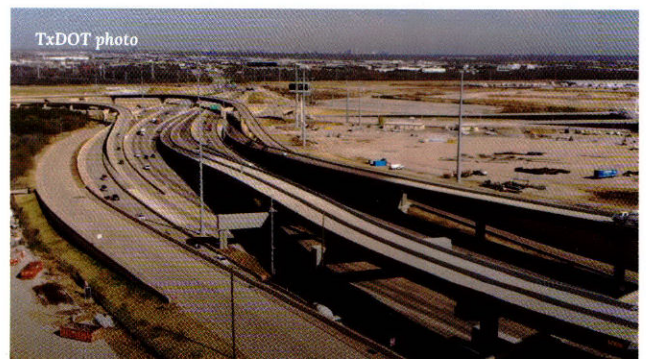
A virtual groundbreaking was held in April for the Irving Interchange Project.
